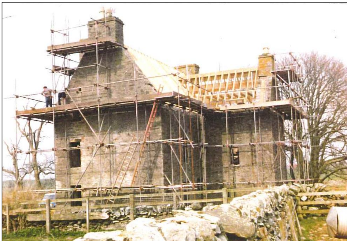
The roof timbers were beyond repair and are new, but the slates were either re-used or replaced by old slates from the steading.
