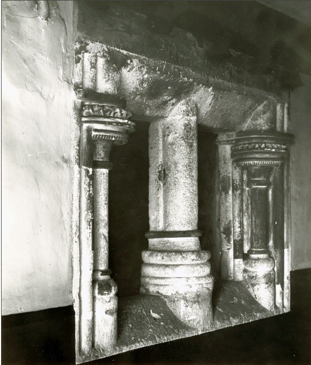
The mysterious window, or hatch, in the South block with its 13 th century shafts.
