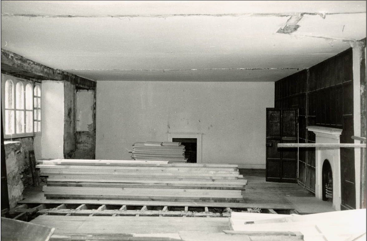
The first floor after the 1819 partitions were taken down. New floor boards had to be laid.
