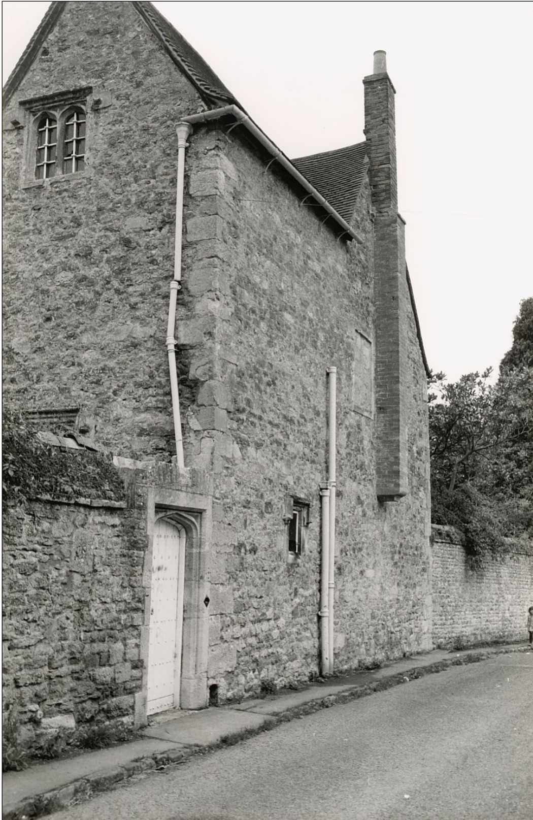
The North end in 1979, before the 1839 porch was pulled down, and the door moved a few feet west, to its present position.
