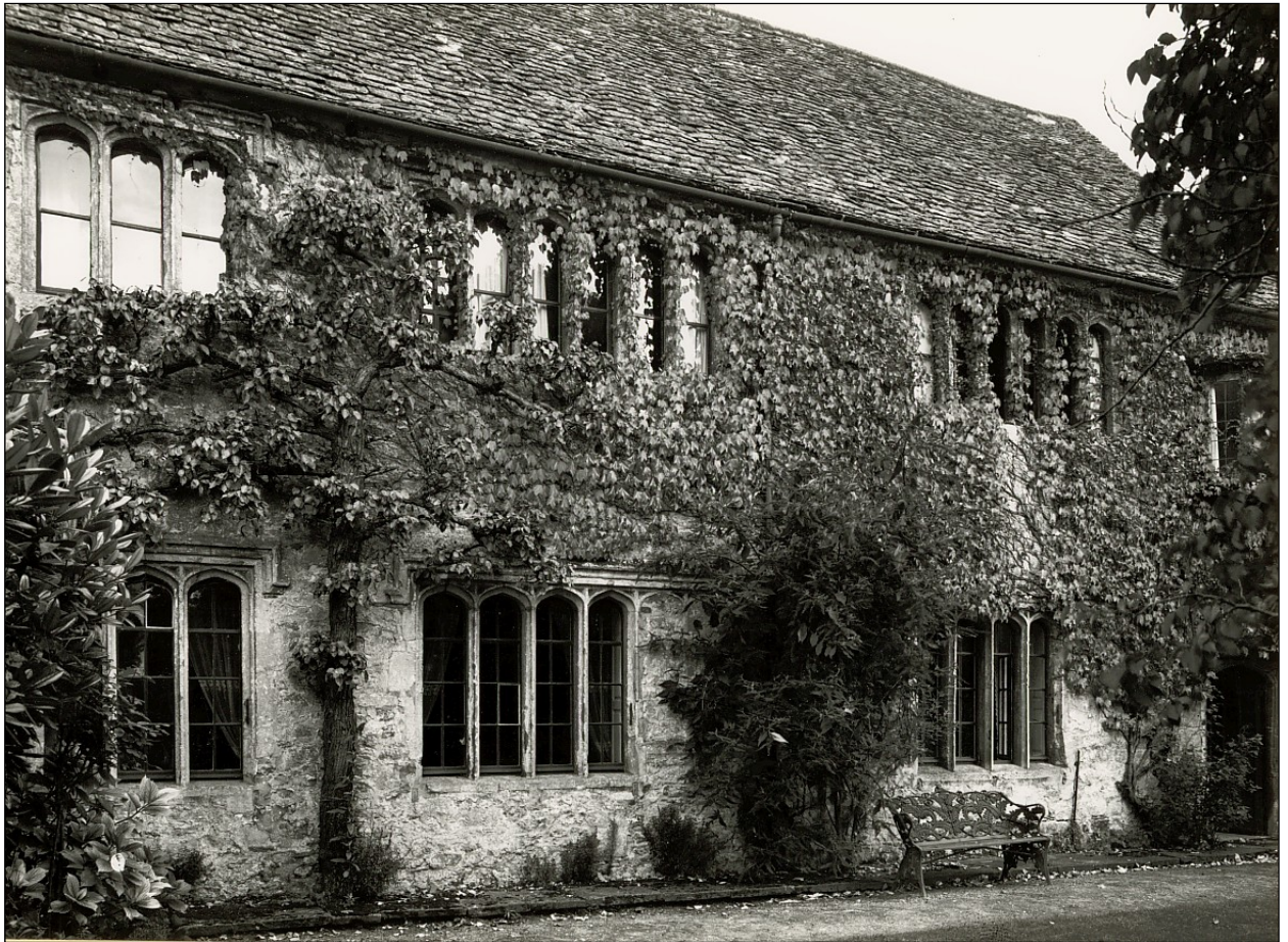
The west front in 1937. The blocked window lights of the central window can clearly be seen.
