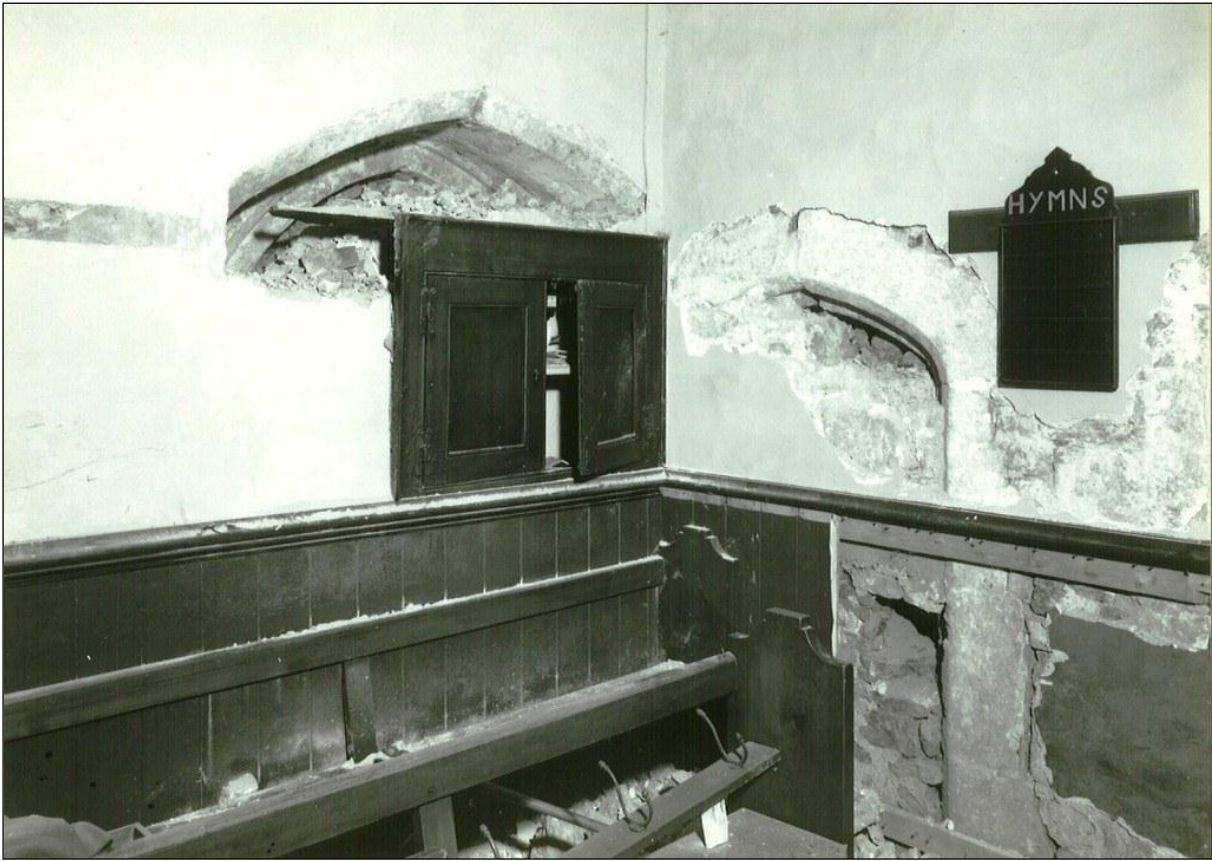
The blocked doorway at the south end of the hall and the staircase door
