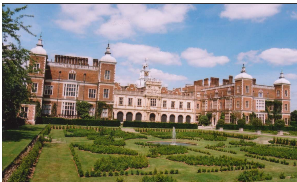
The south elevation of Hatfield House showing the open loggia, portico (with an attempt at Classical orders), Flemish gables and lantern, all of which may have been references for Campden House.
