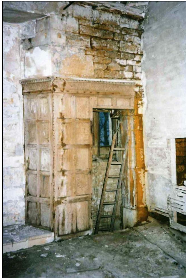
Panelling surviving on the upper floor.
