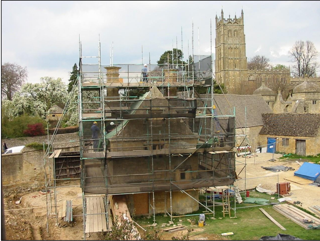
The Almonry viewed from West Banqueting House during repair in April 2002.
