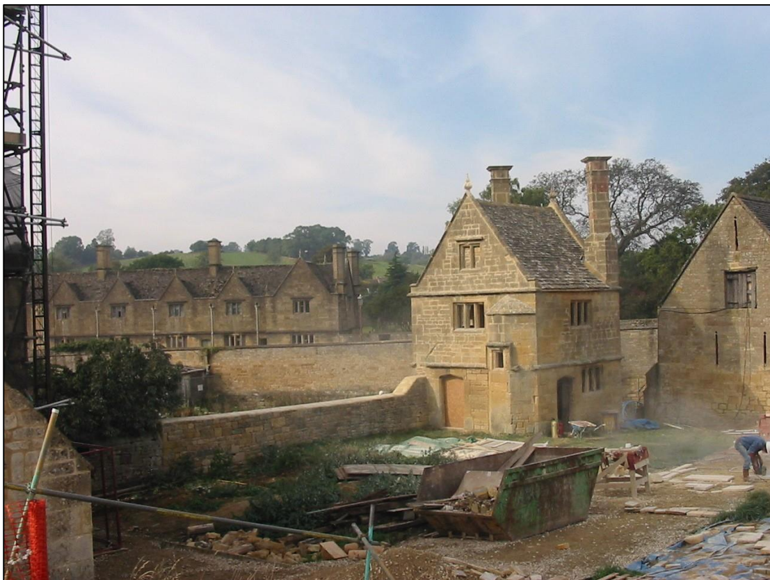
Looking towards the SW corner of the Almonry.
