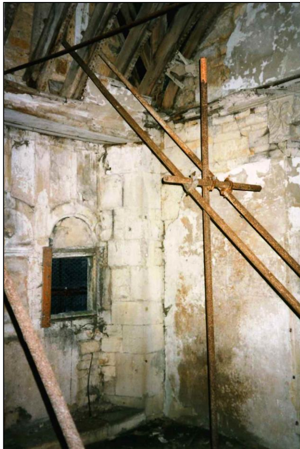
Part of the wall and roof structure of the upper level.
