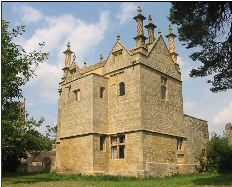
The view of the south-west elevation after restoration showing the unblocked west window and the re-blocked lower half of the window on the south.
