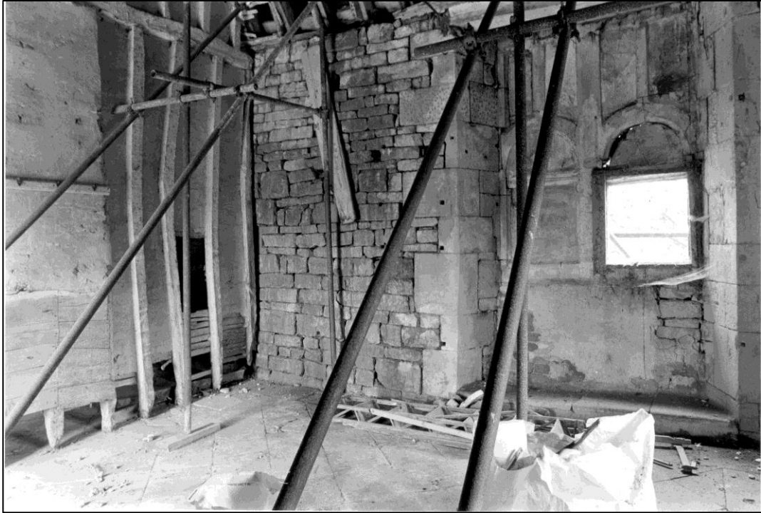
The first floor before restoration.
