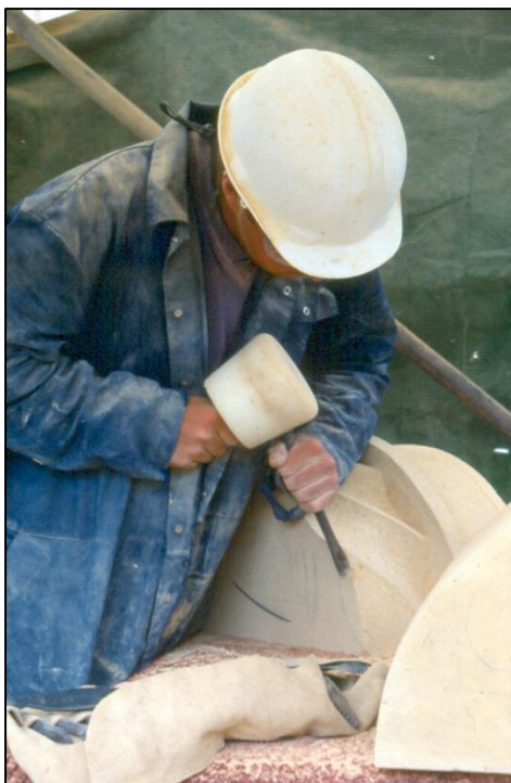
Chiselling the 'barley sugar' fluting on the new chimneys.
