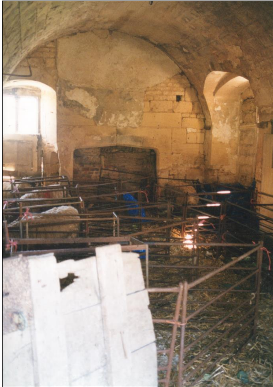
The ground floor of the West Banqueting House in April 1998 before restoration - during the lambing season!
