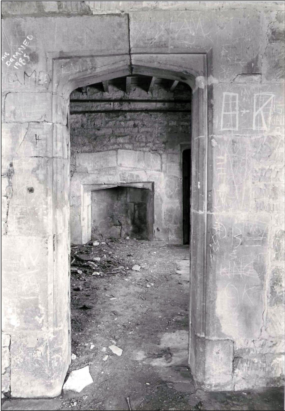
Looking north into the kitchen.
