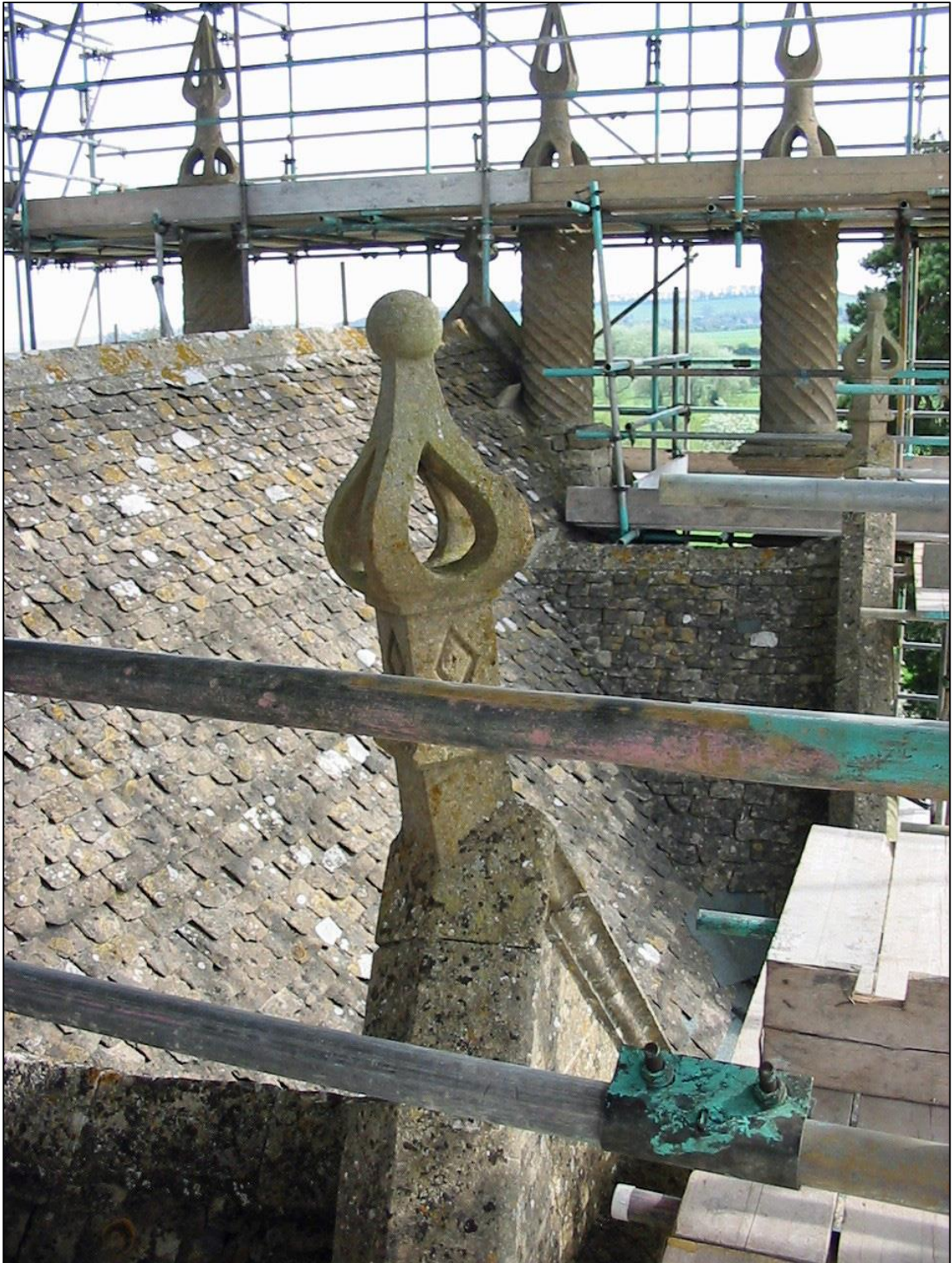
The roof undergoing repair.
