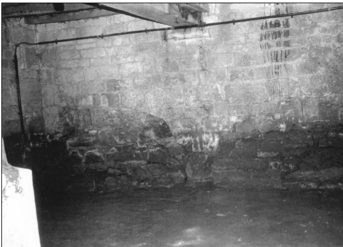
The cellar of the Almonry, showing the possible conduit arches built into the wall (now blocked) and drainage channel down the centre.
