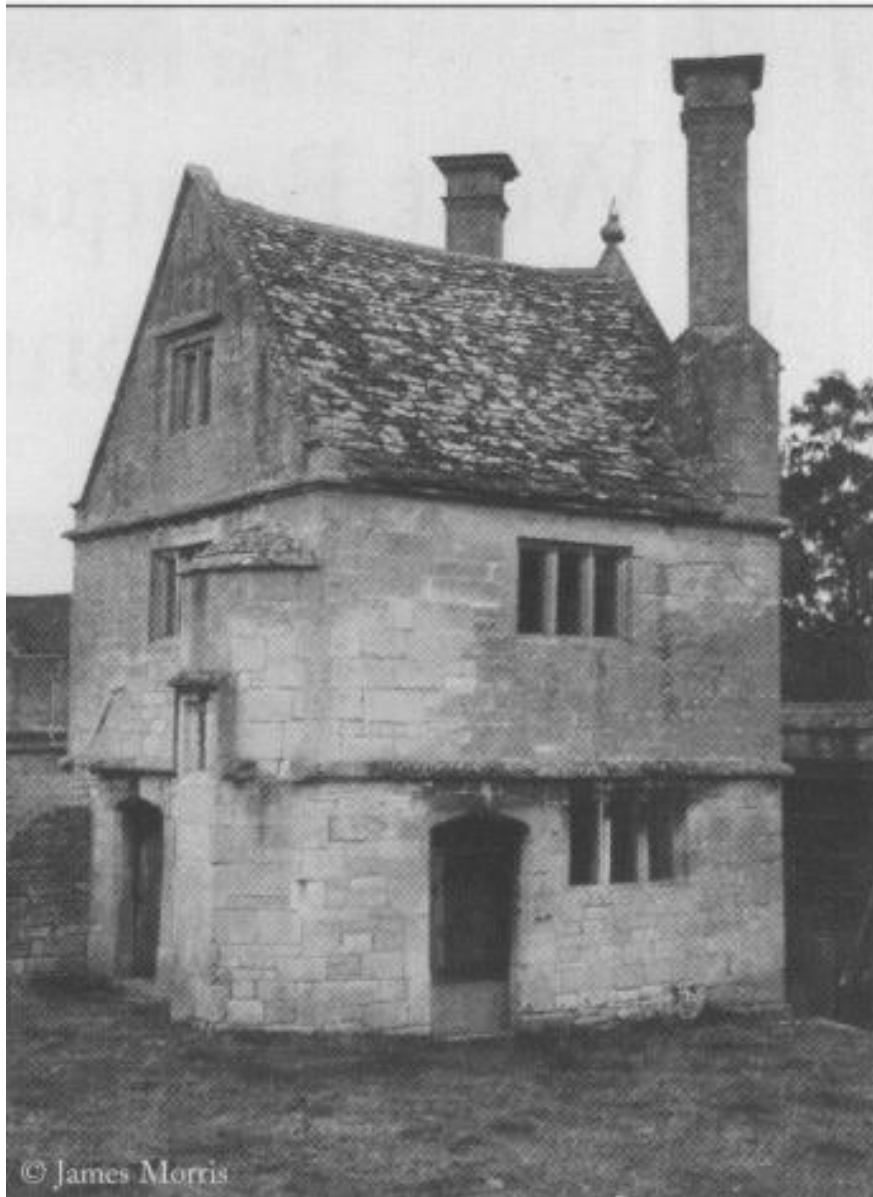
The Almonry before restoration.
