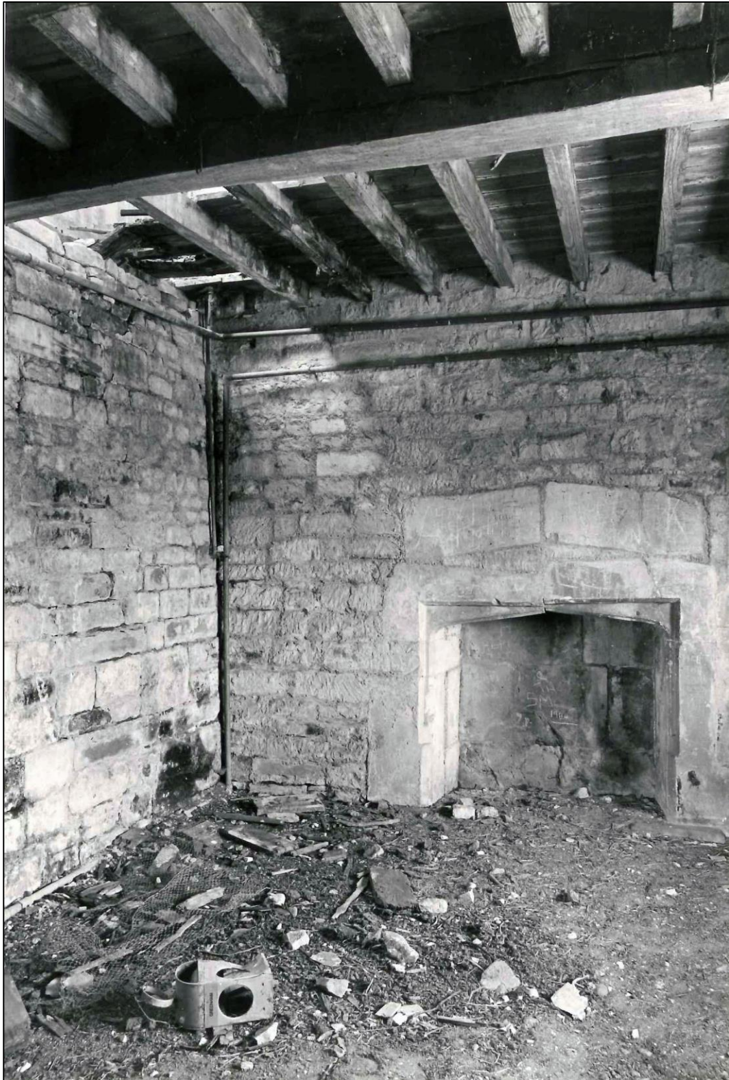
The staircase up to the top floor is now in this corner.
