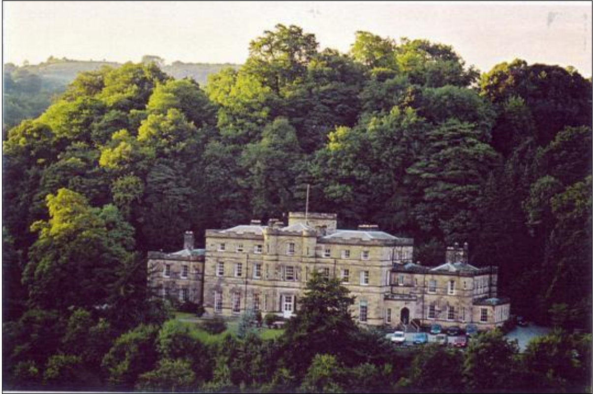
Figure 24: Willersley castle – ‘the house of an overseer surveying the works’.
