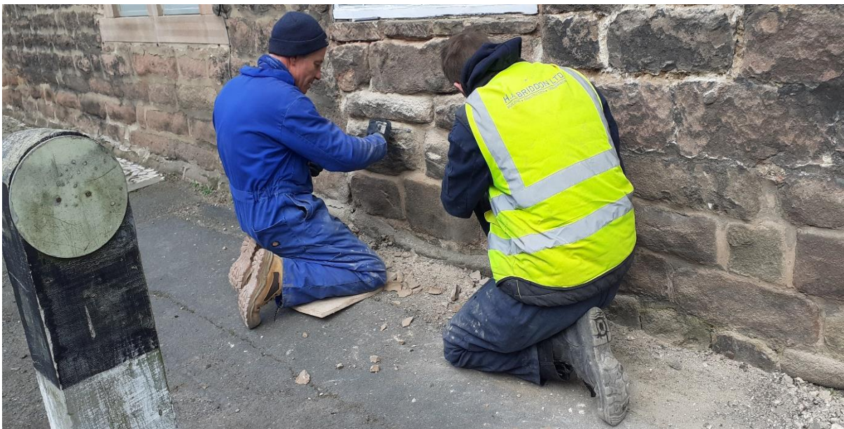
Apprentice Adam Winson worked alongside the experienced masons, gaining valuable experience, here raking out cement pointing with Ian Williams.
