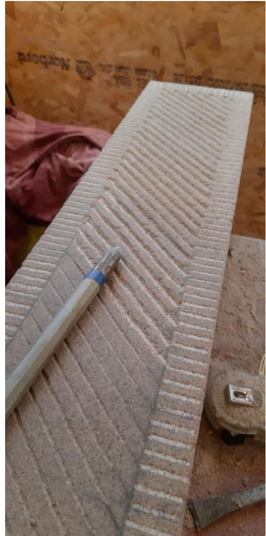
Lead mason Ian Williams working in the bankers shed, and a half-tooled replacement window sill, an example of his work.
