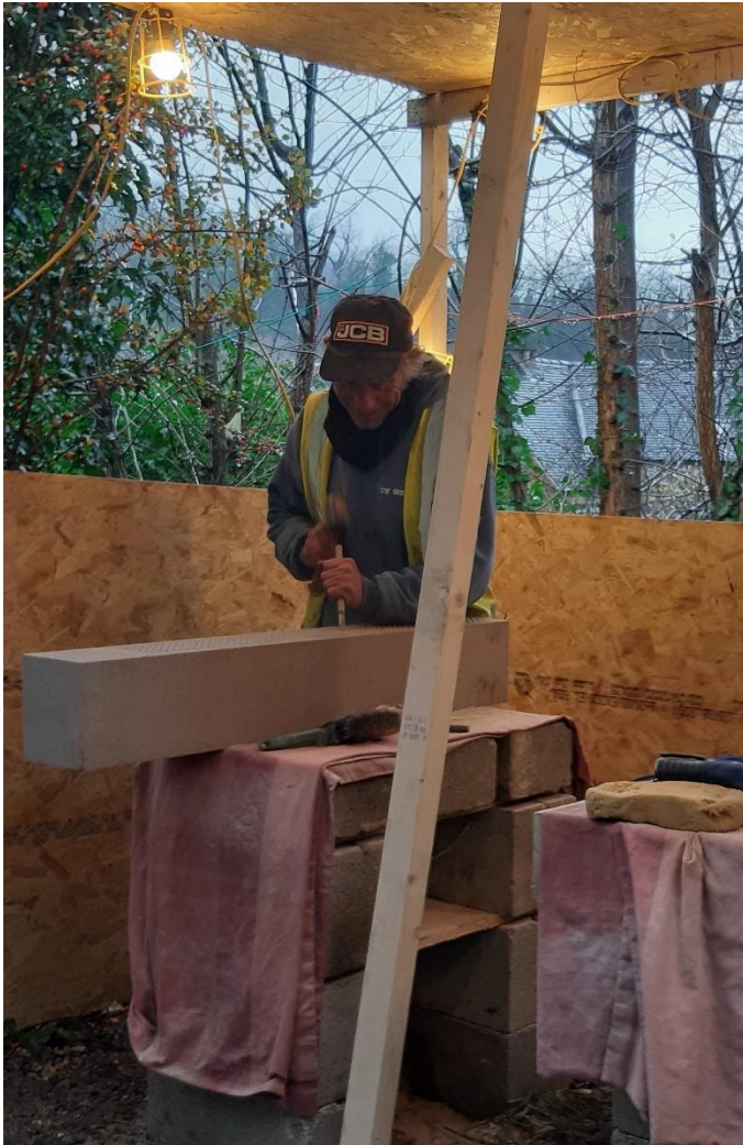
Lead mason Ian Williams working in the bankers shed, and a half-tooled replacement window sill, an example of his work.
