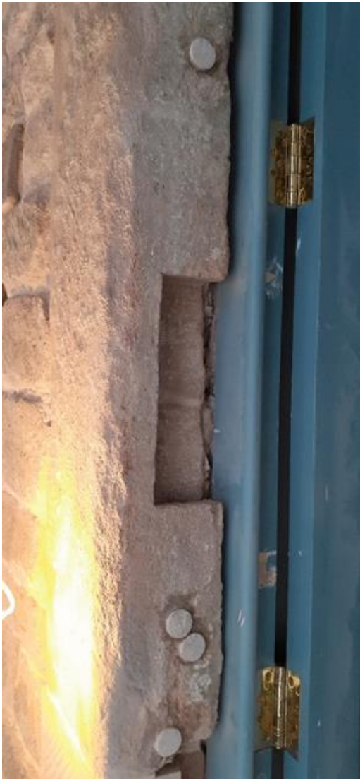
Top: Site foreman Neil Goddall with Stuart Leavy. Below left: new stone dowels tying a door jamb firmly in place. Below right: Stuart and Susan McDonough, Landmark's Head of Historic Estate, inspecting the repaired chimney stacks.
