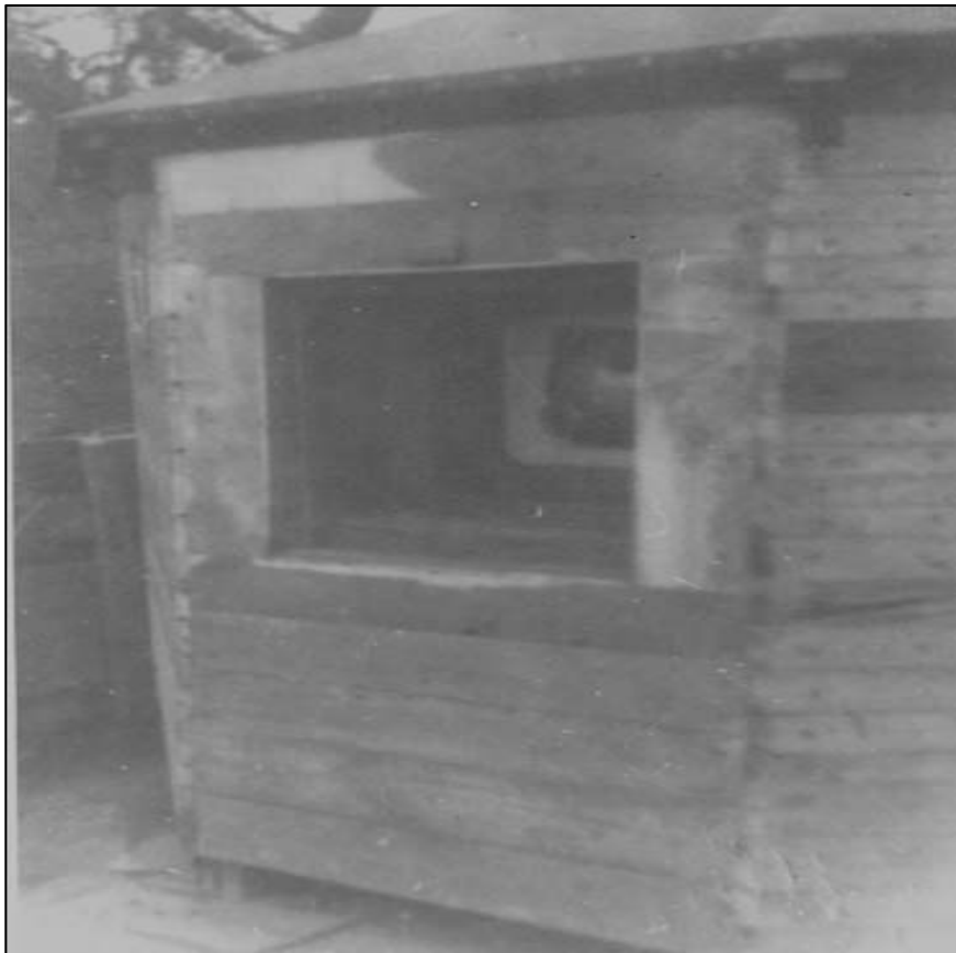
Front view of the summerhouse
