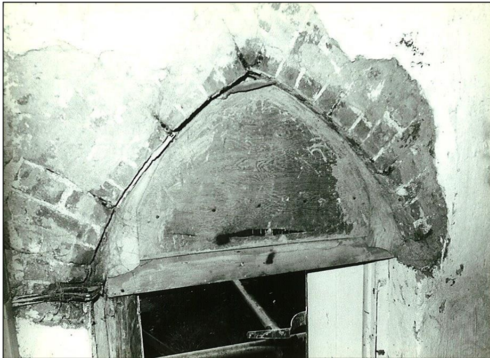
First floor in 1982.
