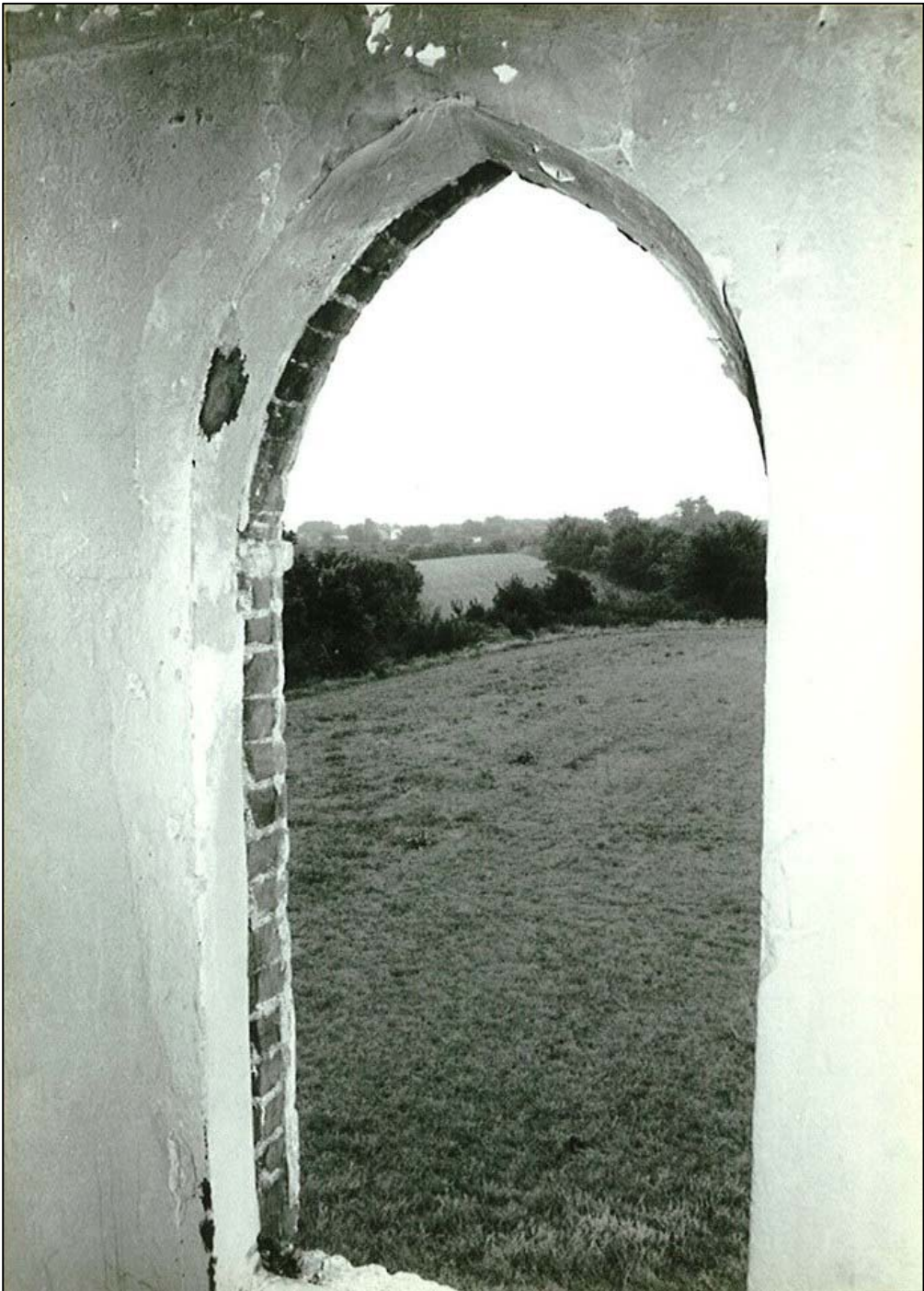
A first floor window
