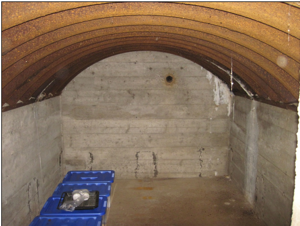
Bunker 4 is a larger Wellbech type shelter and originally had steps going down into it from the front door of the Tower, the steps remain but the entrance is now blocked. This was for troops to quickly access, in case the Tower was attacked.
