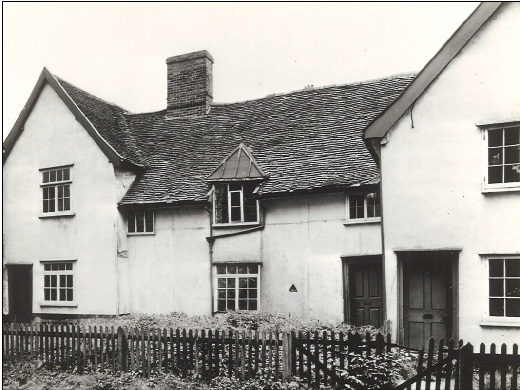
New Inn in the 1930s, with inserted windows, doors and dormer. Note too the large brick chimney stack projecting above the roof from the hall, and removed during the 1970s restoration.
