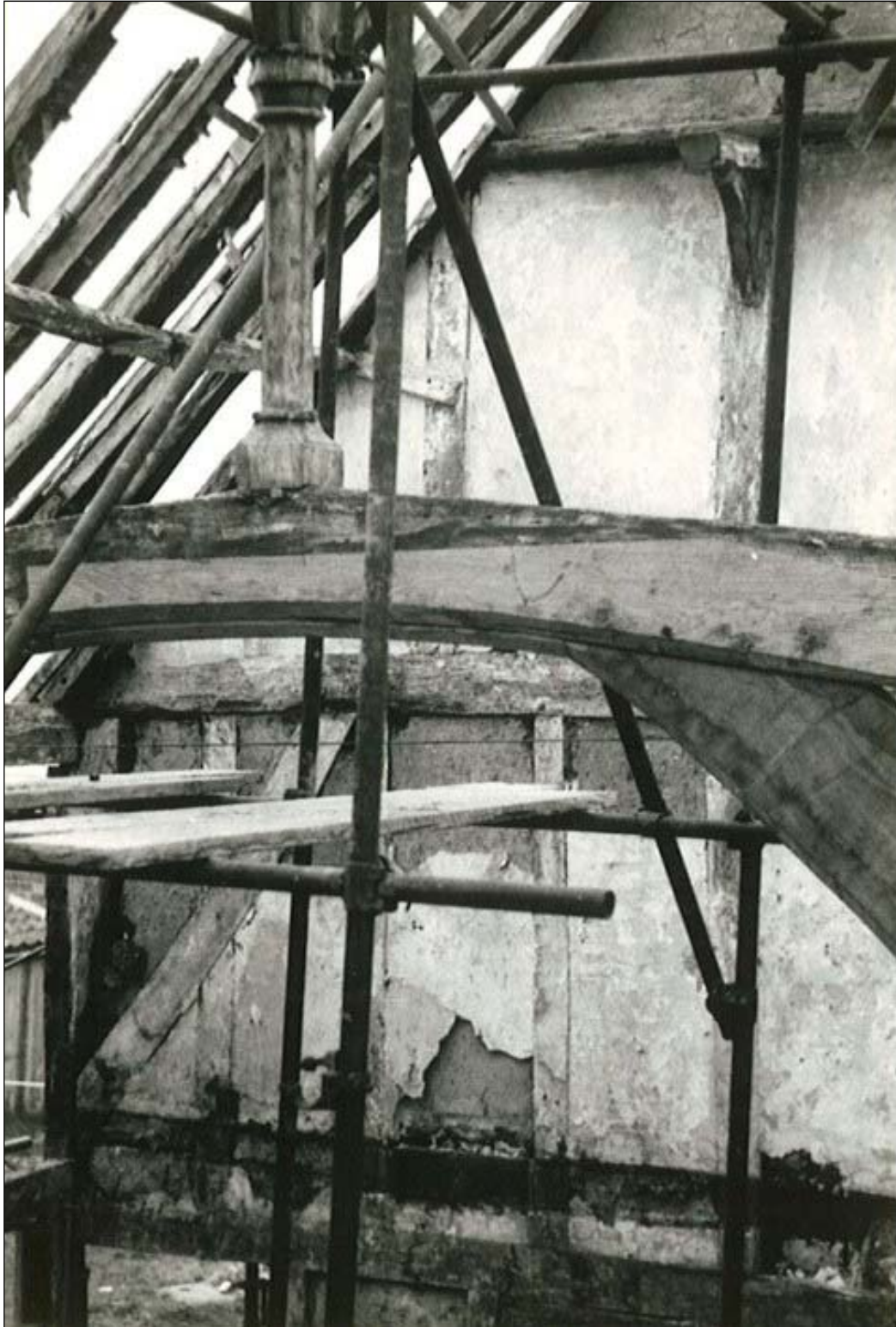
The inserted floor, later ceilings and partition have now been removed from the hall, revealing the crown post.
