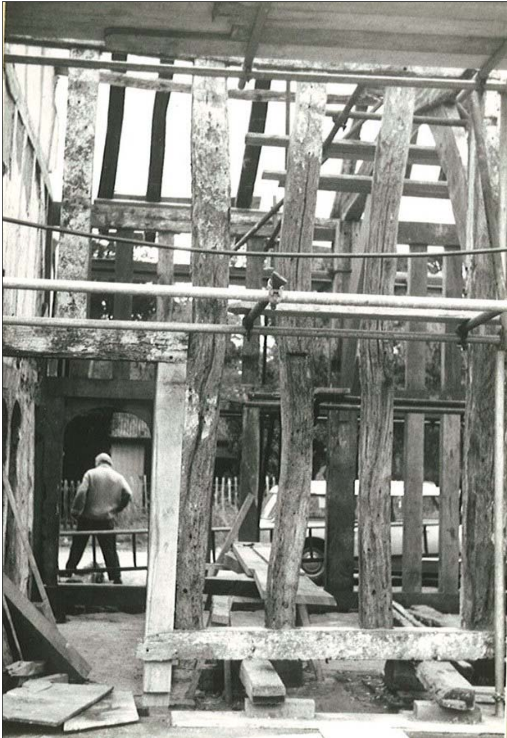
Work in progress, looking into the hall from the rear.
