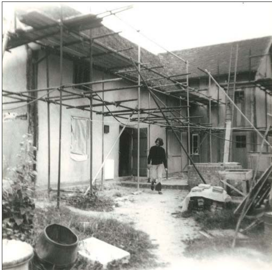
Restoration of the rear nearing completion.
