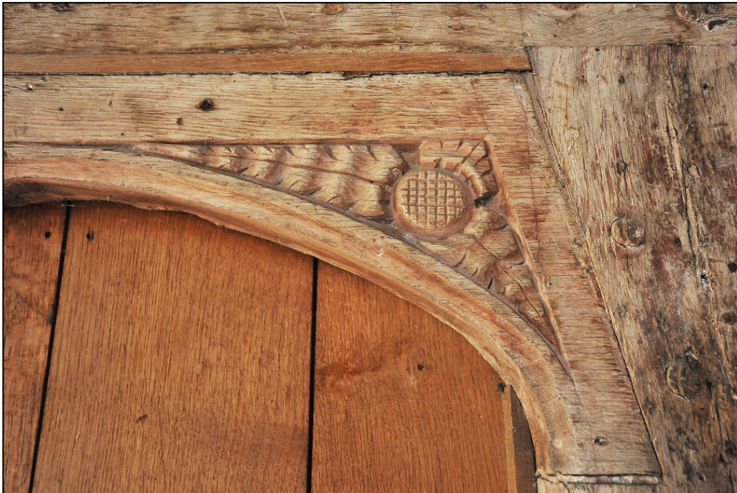
A finely carved spandrel in doorway from the hall to the low end, and the moulded wall plate on the jettied wall plate to the 17 th -century extension to low end.
