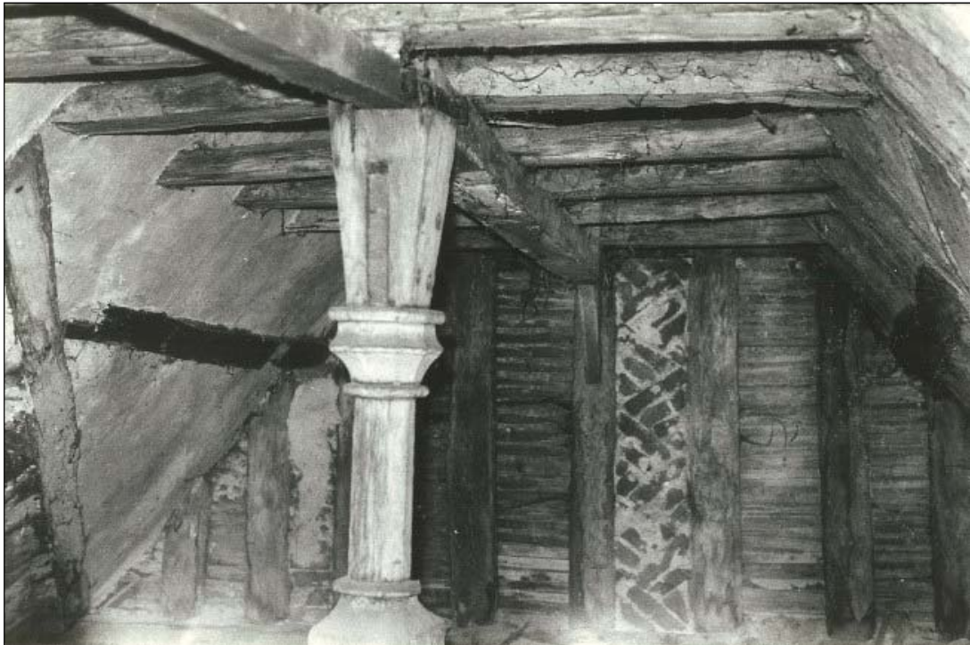
The crown post in the high end chamber.
