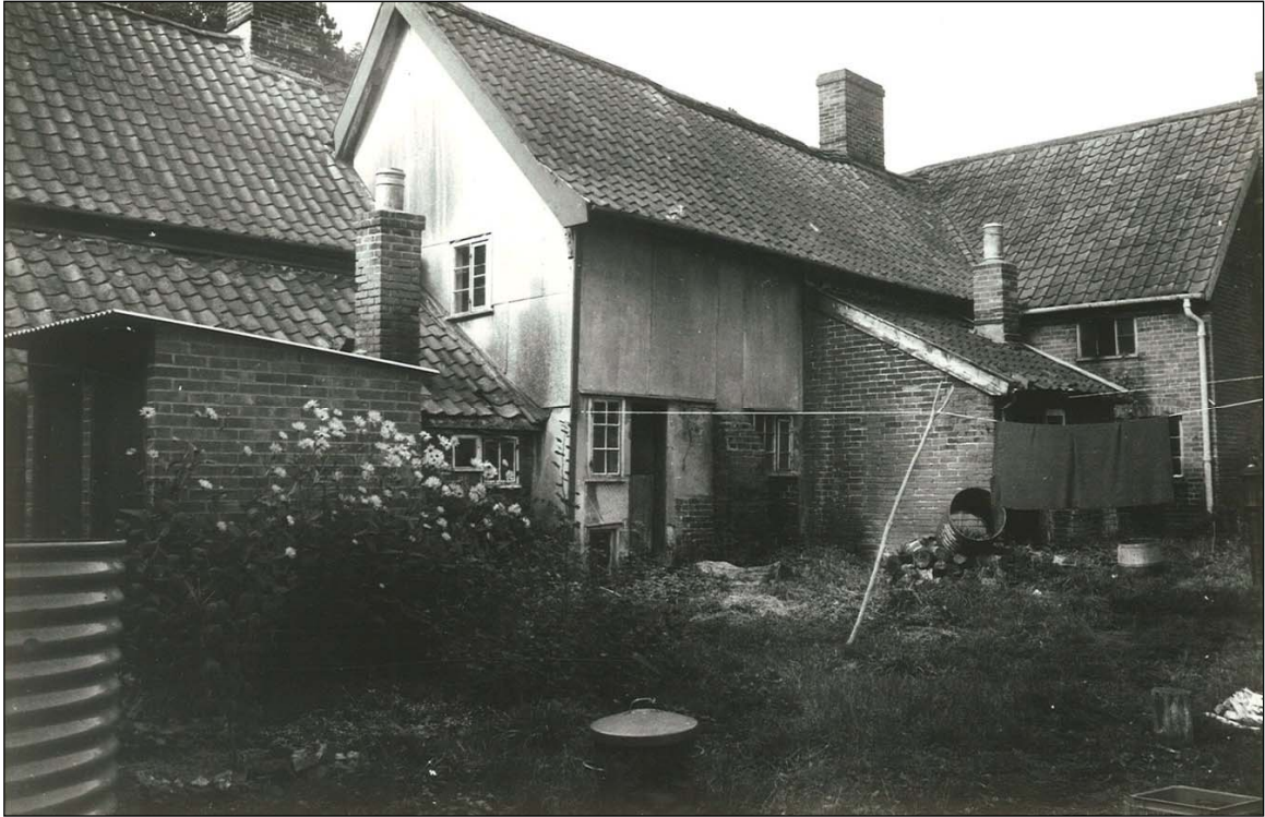
The back of the New Inn before it was restored. The brick lean-to was removed.
