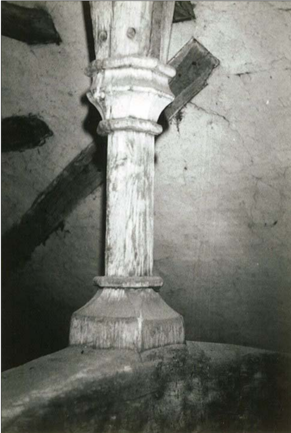
Crown post in the high end chamber prior to restoration. The crown post at that time was completely concealed from view by a ceiling inserted below the tie beam, so it was an exciting discovery.
