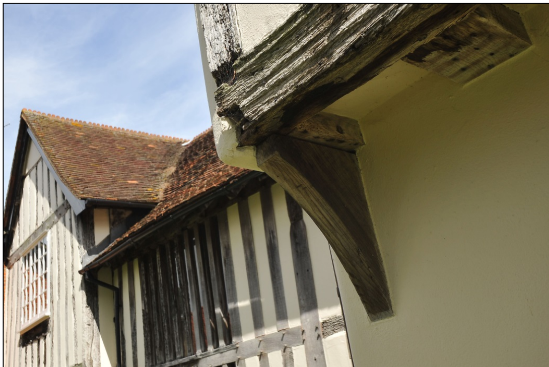
A finely carved spandrel in doorway from the hall to the low end, and the moulded wall plate on the jettied wall plate to the 17 th -century extension to low end.
