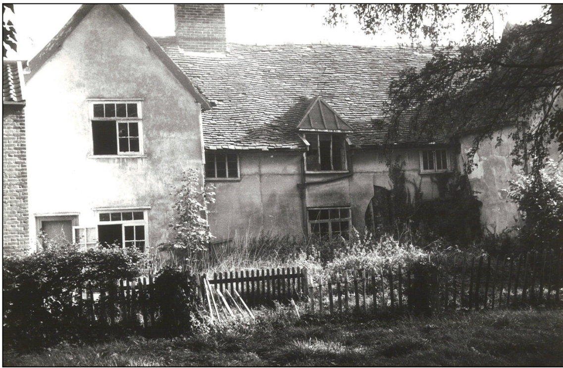
New Inn in 1971, by now known as Knoll Cottages. Its medieval character is hardly apparent behind later render and inserted window frames.
