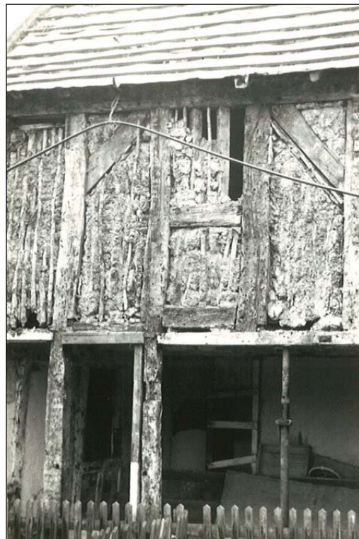
The same wall showing the complete window.
