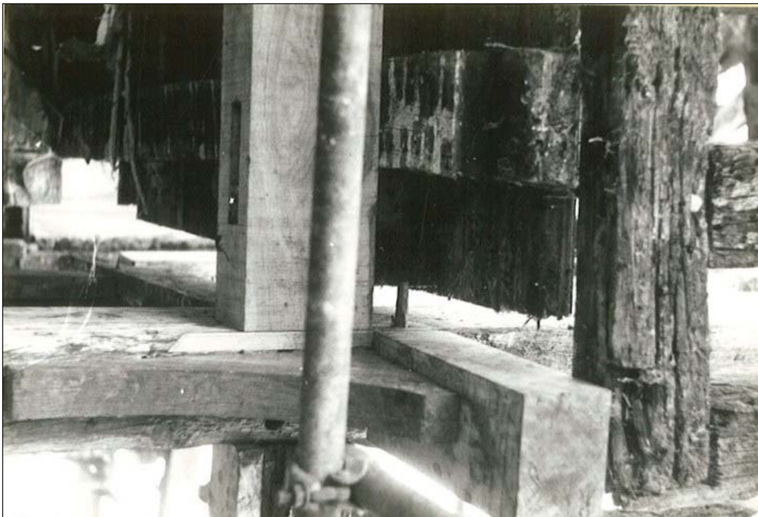
New timbers and bracket inserted beneath the jetty at the high end.
