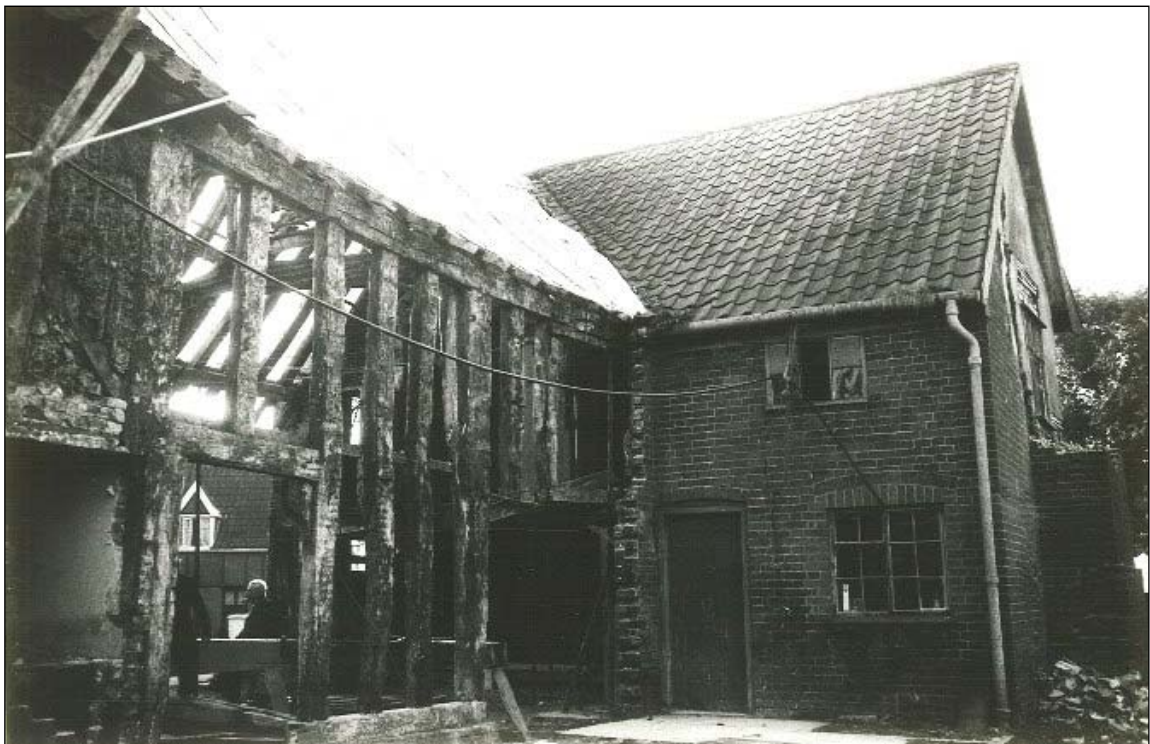
The back of the New Inn being restored.
