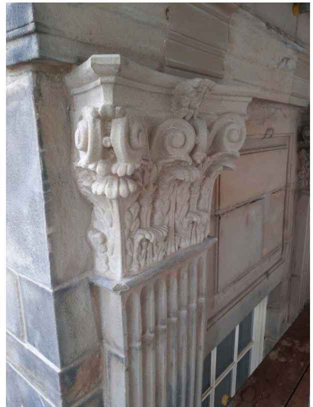
The replacement of the capital, which had 'exploded' due to corroded (so expanded) iron clamps. The craftsmanship of the replacement is clear, as the mason fine-tuned it before it was fitted. Note too the careful repointing.
