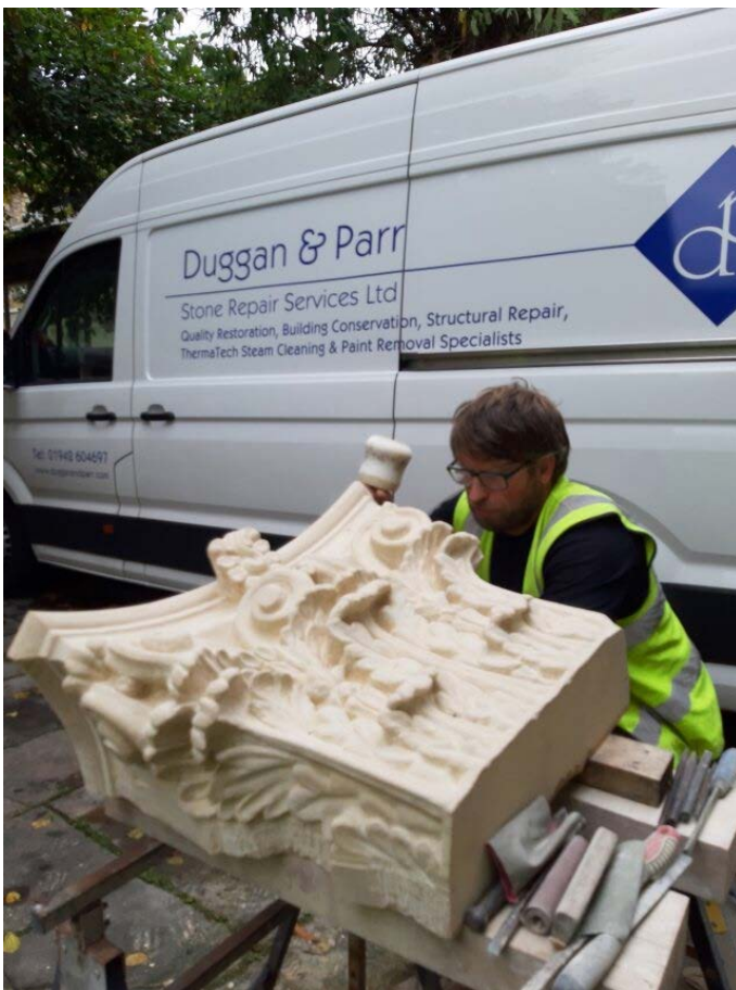
The replacement of the capital, which had 'exploded' due to corroded (so expanded) iron clamps. The craftsmanship of the replacement is clear, as the mason fine-tuned it before it was fitted. Note too the careful repointing.
