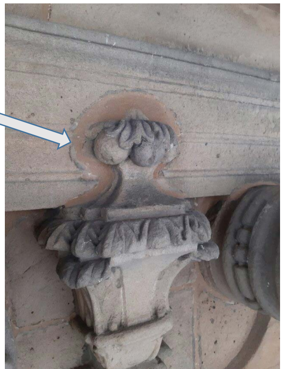
Example of plastic repair on high level stonework: before and after repair.
