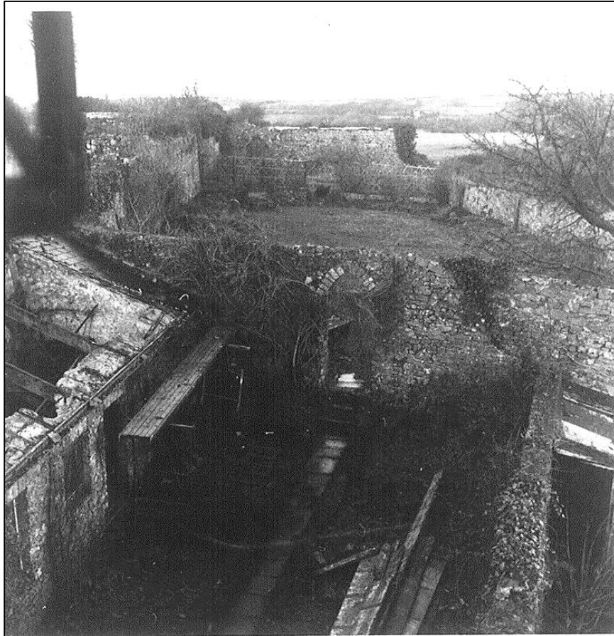
Demolished potting sheds.
