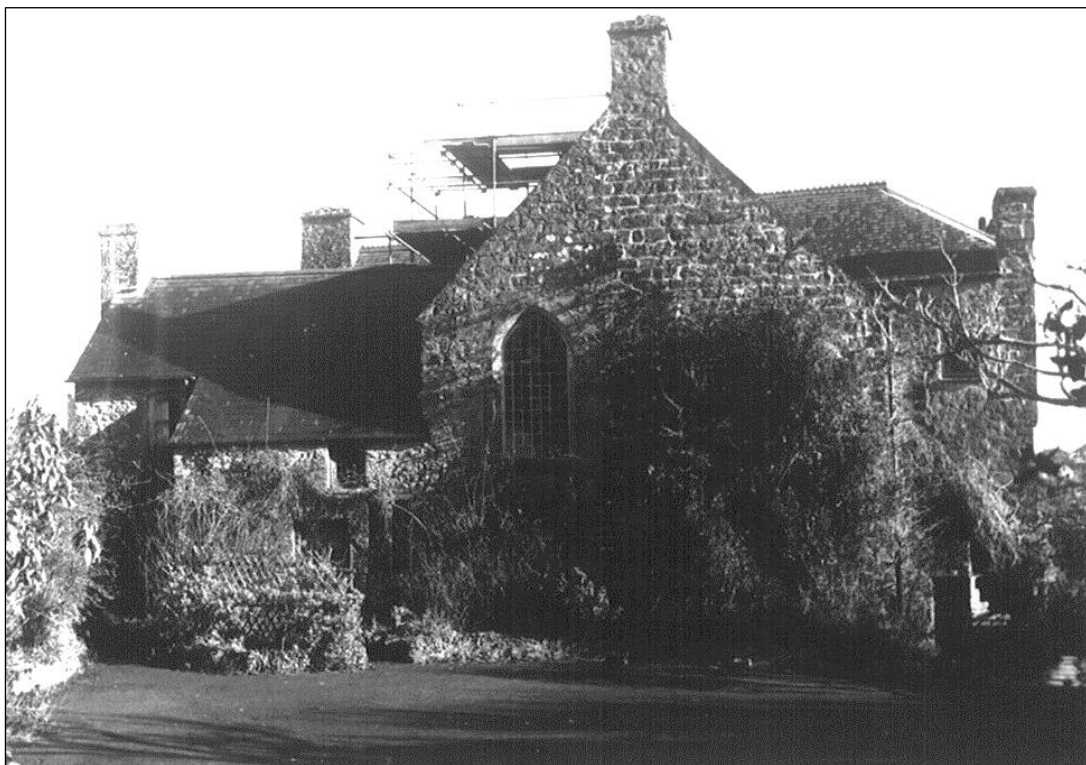
View from the west, with the demolished wing on the left and the former entrance into the SE wing on the right.
