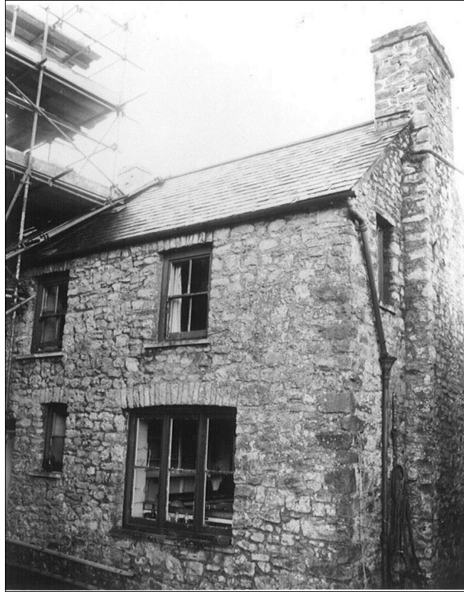
Demolished north west wing form the courtyard.
