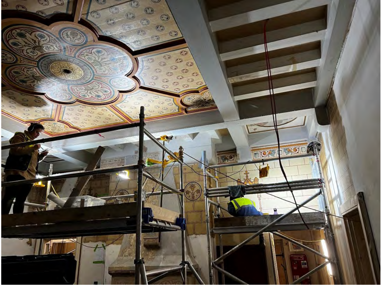
All surviving paintwork on the ceilings was carefully revealed and cleaned using special poultices to draw out the dirt. Only then could touching in begin.
