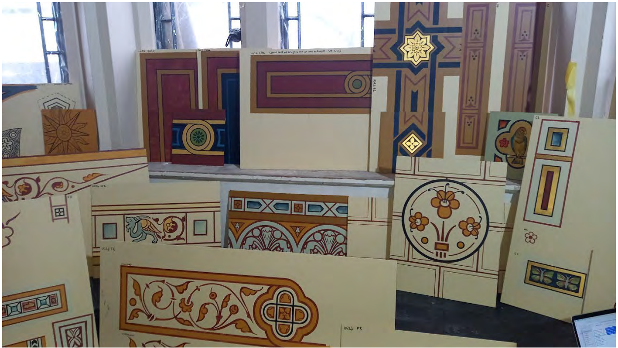
Work underway on the mayor's Parlour decorative scheme, November 2023. Before starting, the conservators created numerous reference panels. Meticulous on-site reference notes were essential.
