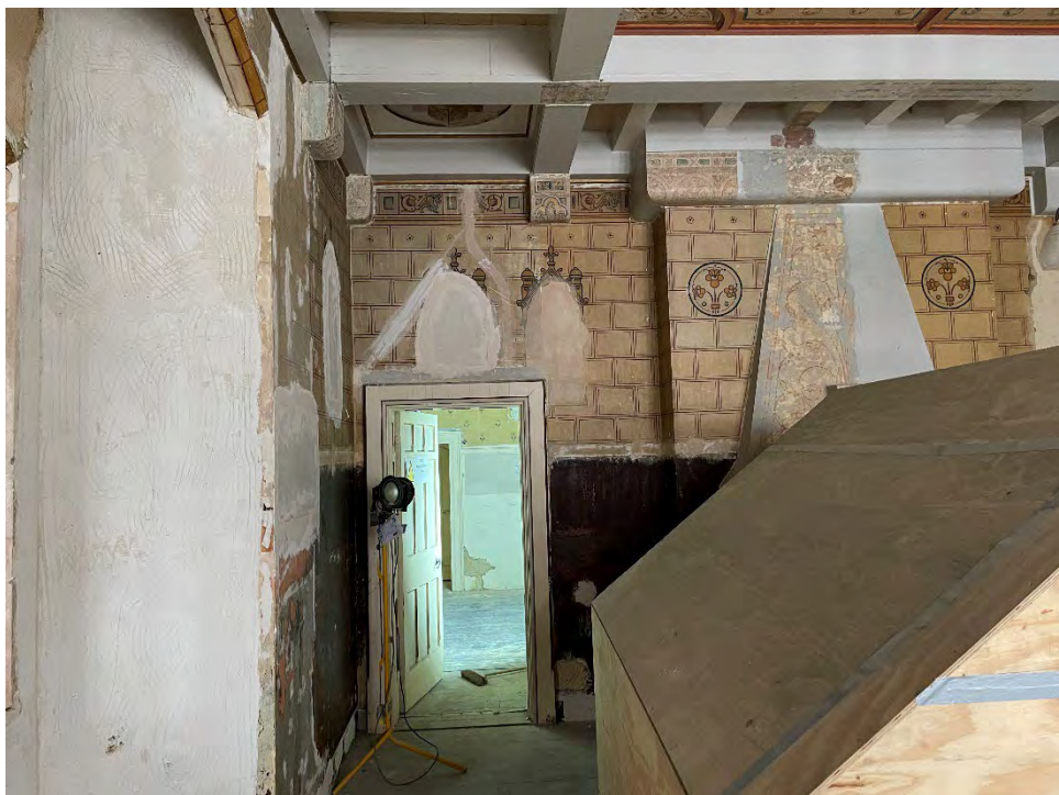
The Mayor's Parlour in 2021. Paint analysis and trial removals had already been carried out and gave a promise of what was waiting to be revealed. The massive table was too large to get out of the building, so had to be boxed in during the works (below).
