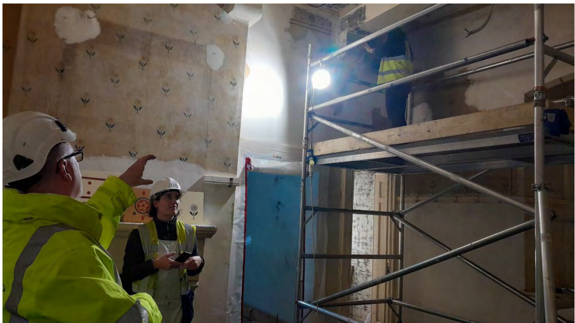
The Magistrates' Retiring Room before work began, now the Landmark's kitchen. Vertical stencils of the daisy runs were used by the paint conservators to ensure the regularity of the setting out.
