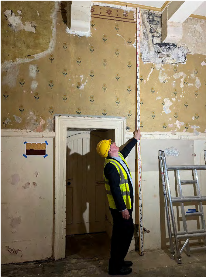
The Magistrates' Retiring Room before work began, now the Landmark's kitchen. Vertical stencils of the daisy runs were used by the paint conservators to ensure the regularity of the setting out.
