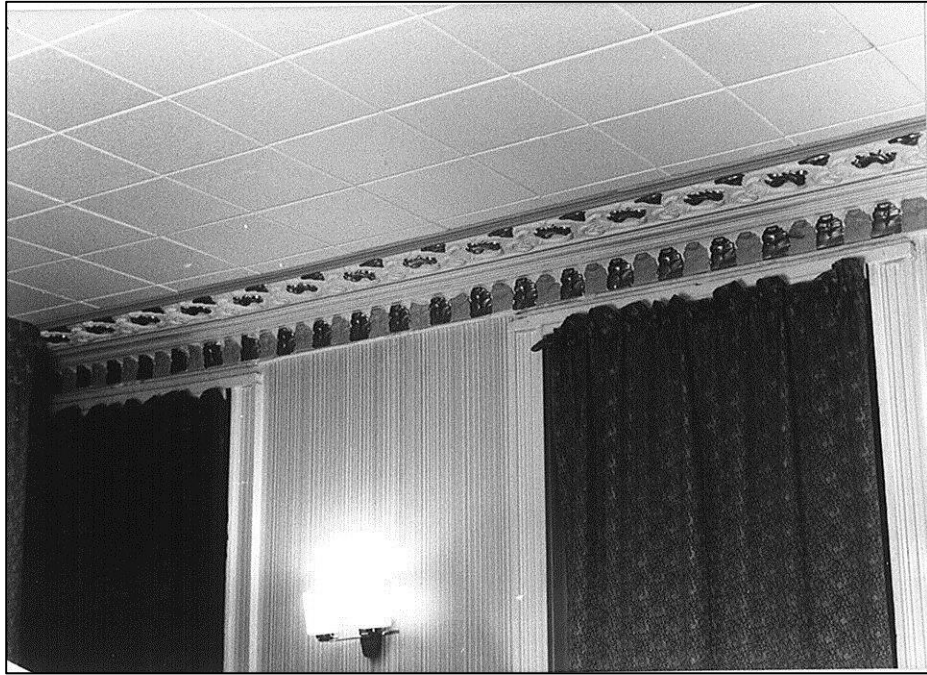
The first floor room in 1975
