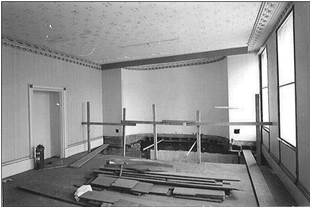
The first floor room in 1975
