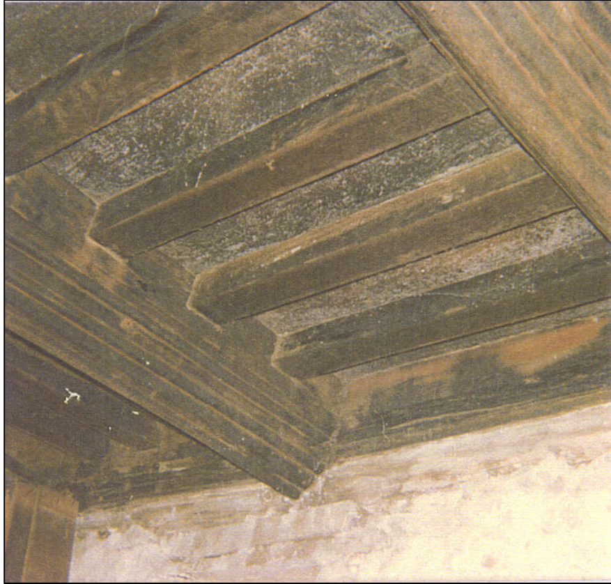
The sitting room ceiling
