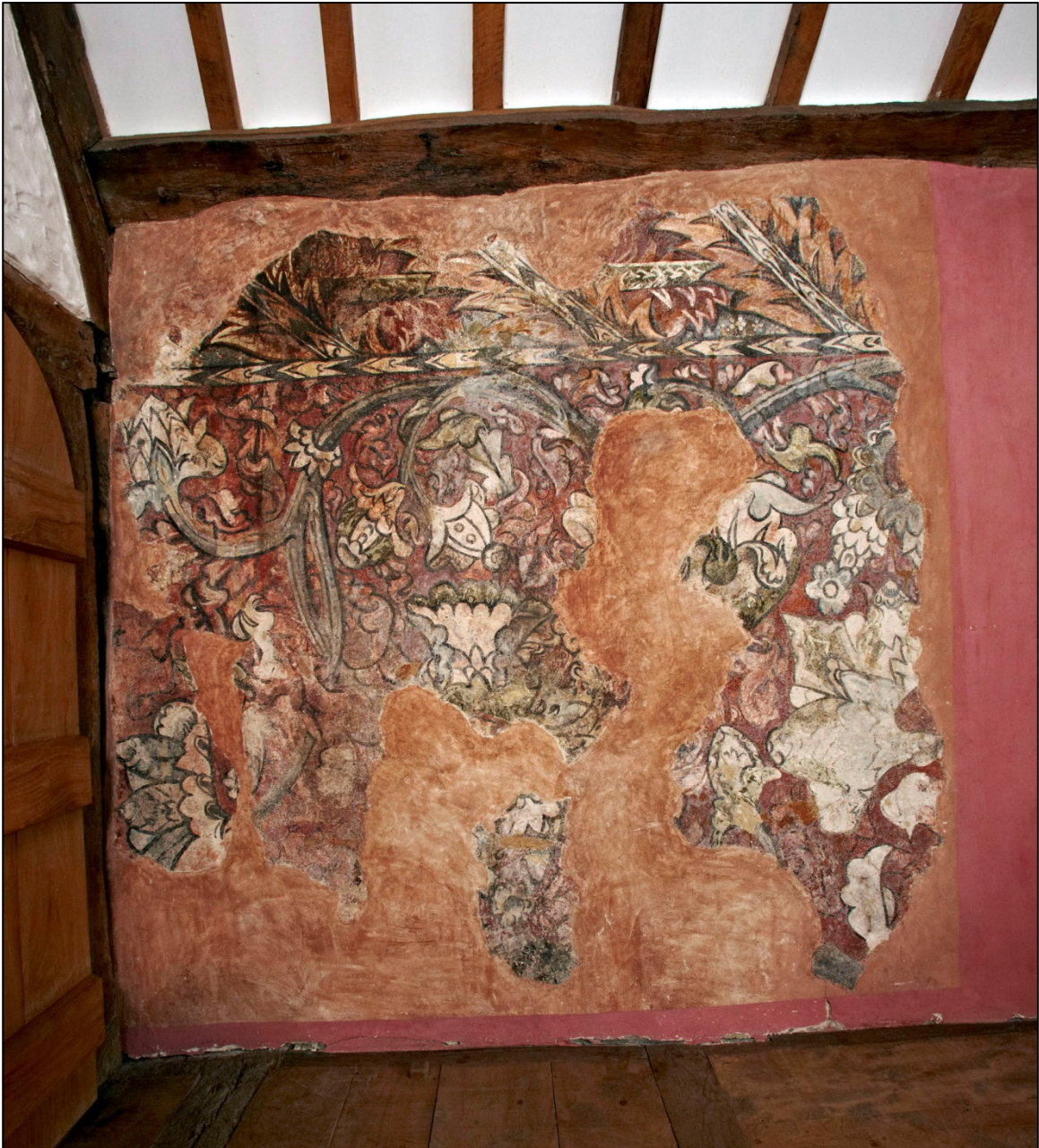
The wall painting after restoration and with the ceiling removed.
