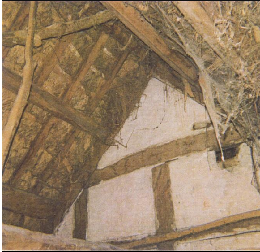
The underside of the thatched roof.
