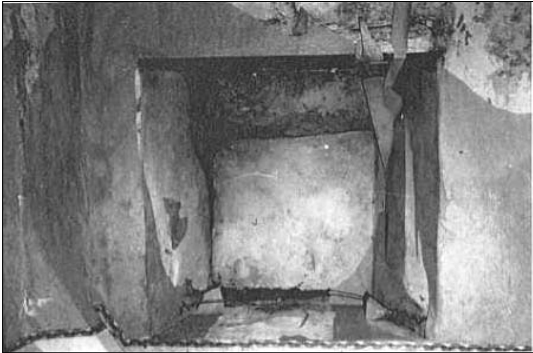
The blocked up east window from inside
