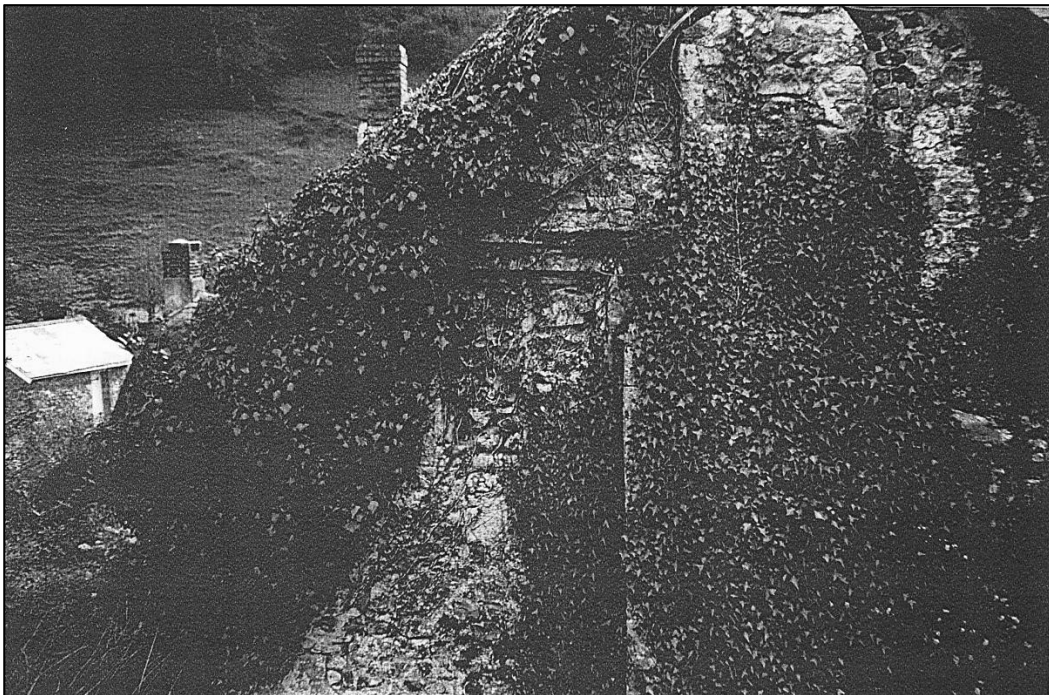
The blocked up east window
