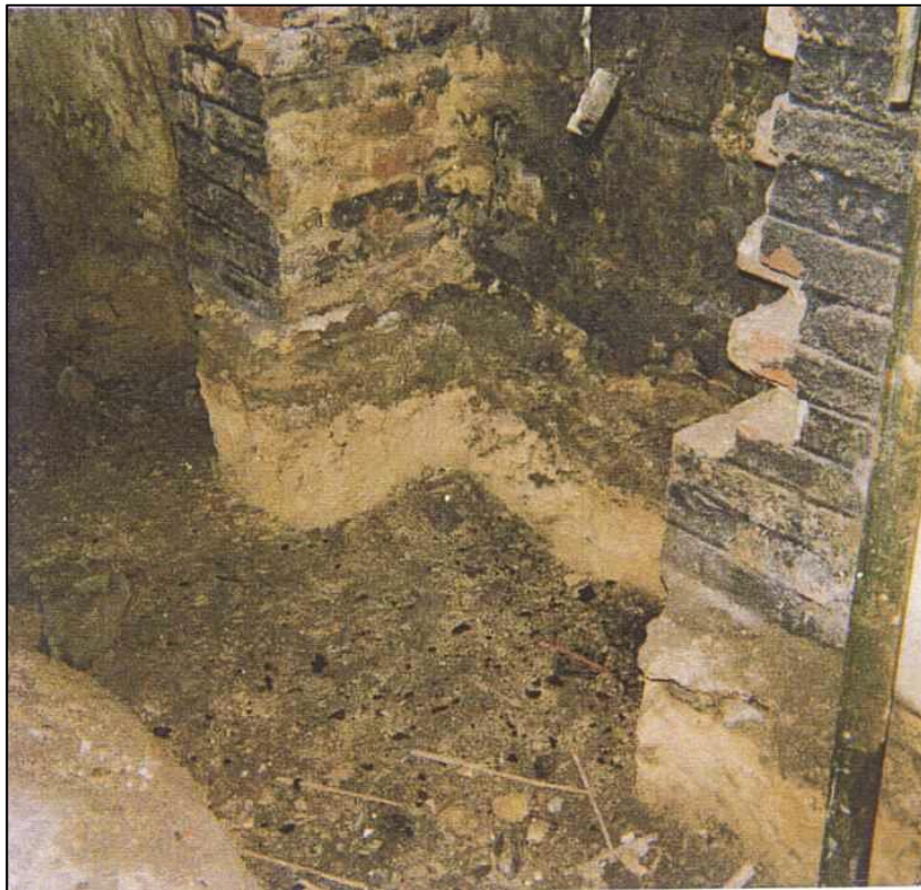
Opening up the kitchen fireplace.
