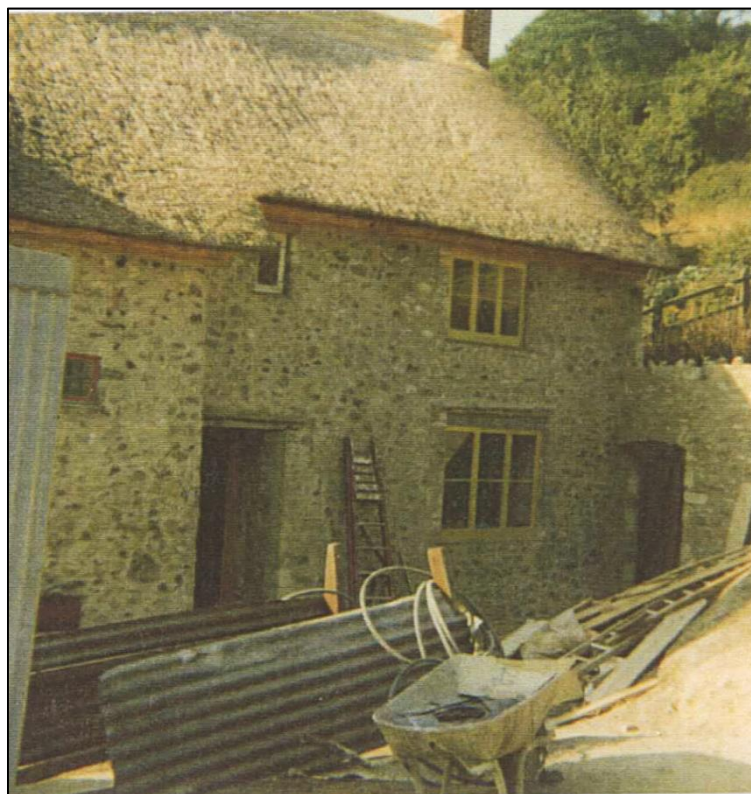
Margells with its new Austrian reed thatched roof.
