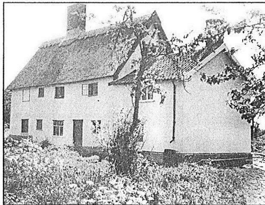
Manor Farm after the completion of repairs.
