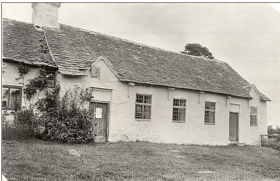
Maesyronnen Chapel before restoration.
