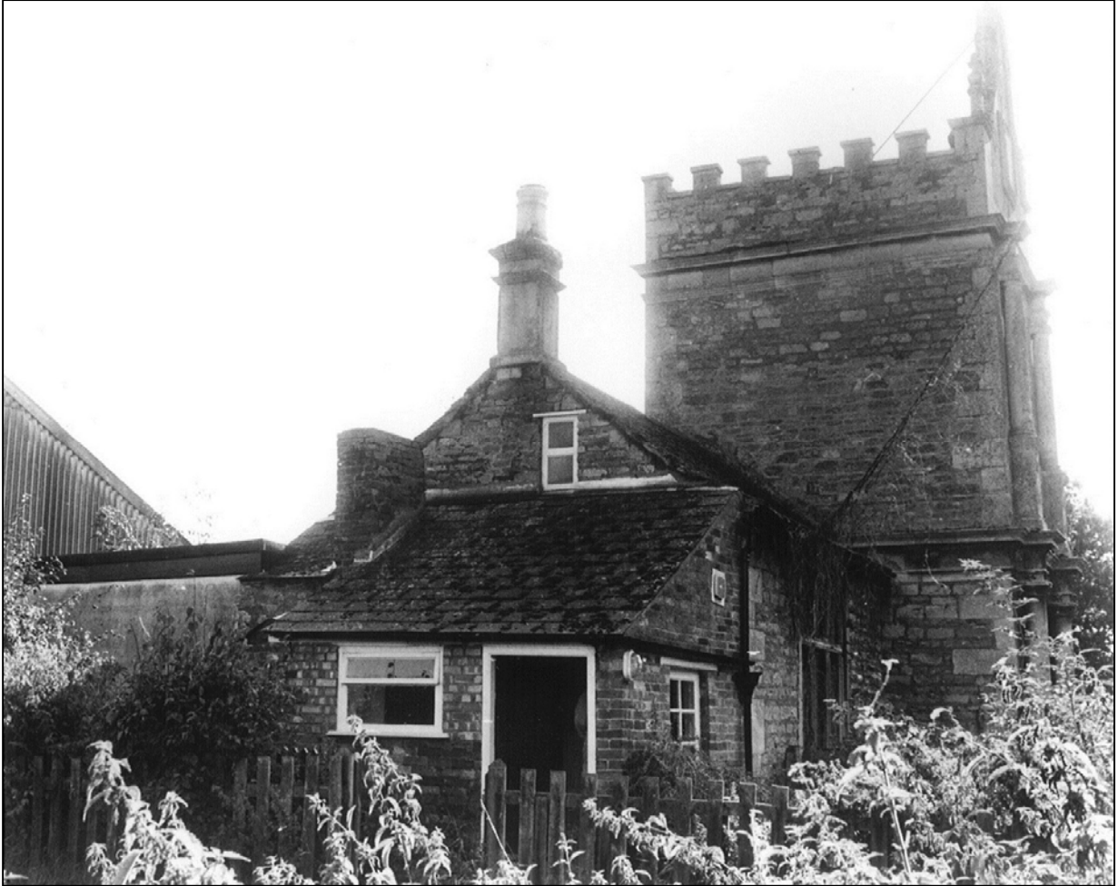
Lynch Lodge from the north showing the 19 th century lean-to kitchen which was removed by Landmark
