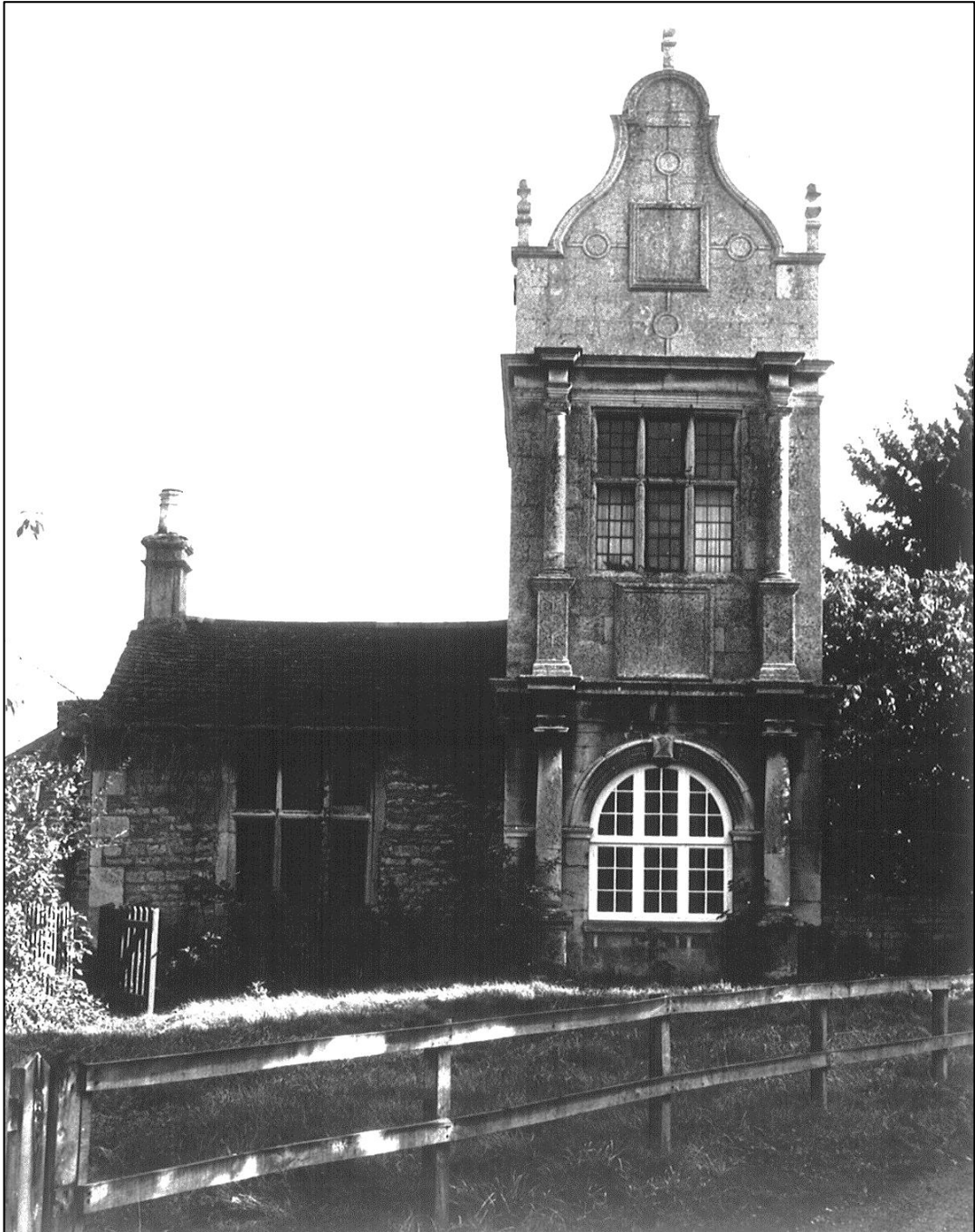
The Lodge in 1981. The window had been inserted into the arch just before, or after the Second World War.
