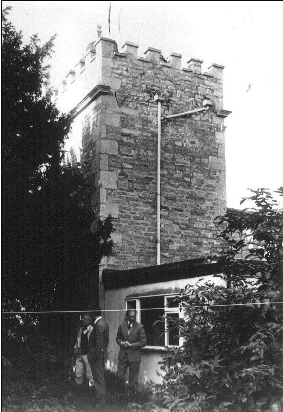
An early reccy around 1981 by Landmark's founder Sir John Smith (right) of the back of the Lodge showing the flat-roofed extension removed by Landmark.
