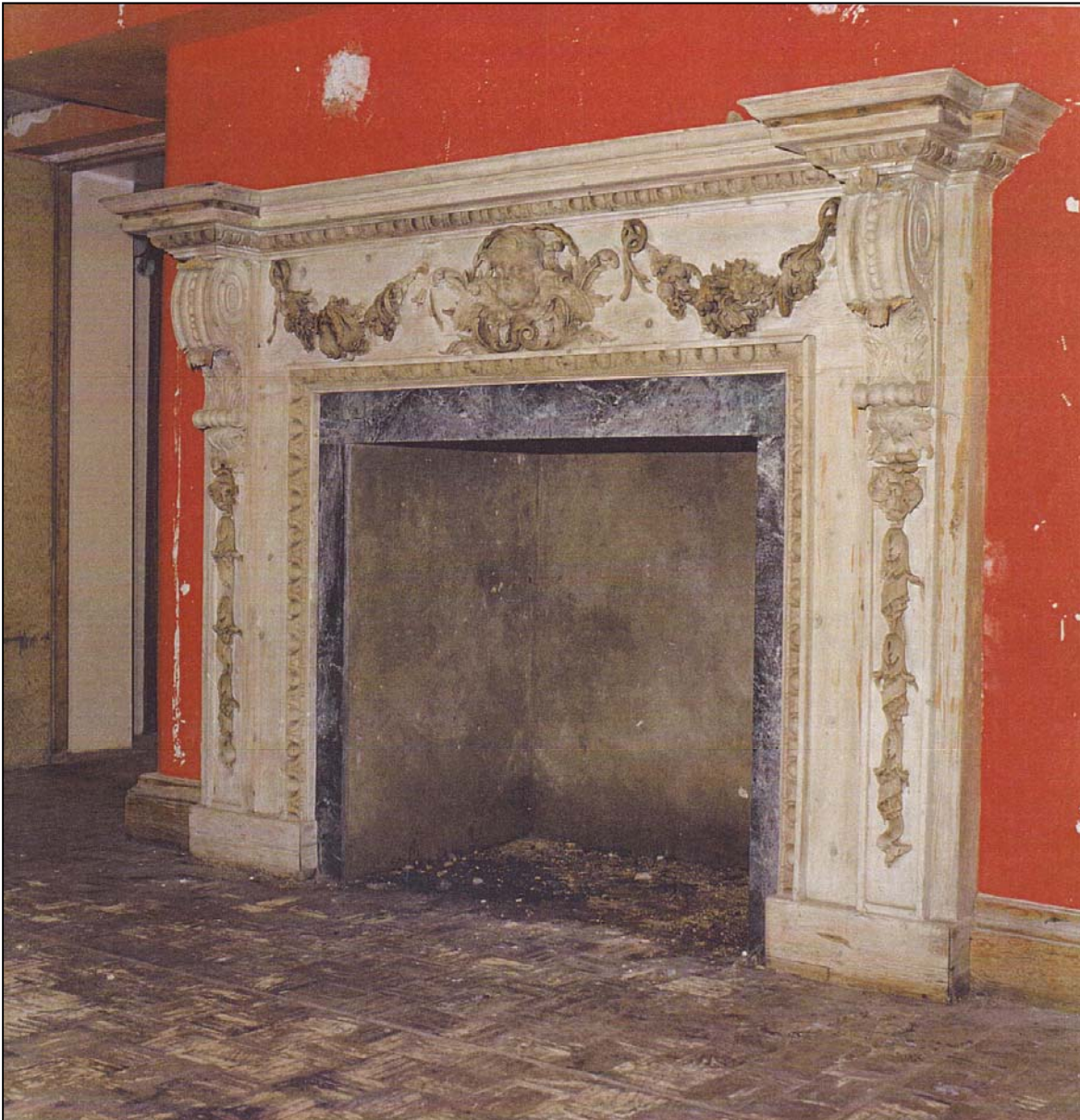
The basement fireplace (now removed).
