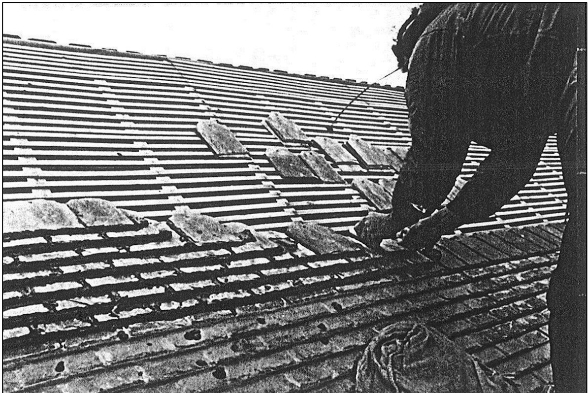
Scantle slate roofing – small slates set in lime mortar
