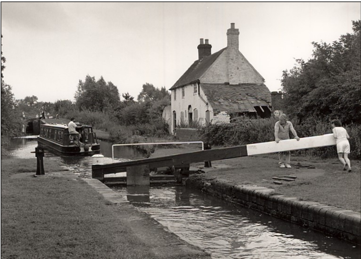
Lock Cottage before repair in 1991.
