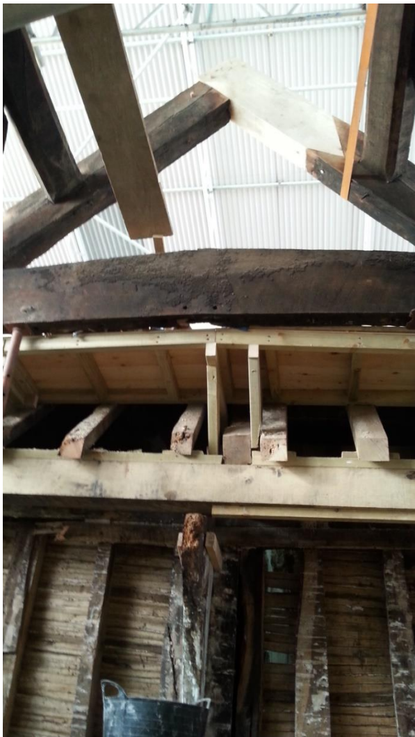
The ground floor of the solar range stripped out, looking south. The ceilings were so low that at some stage a doorhead had been hacked out of the crossbeam (top left). The thickness of the walls is apparent in the window embrasures.
