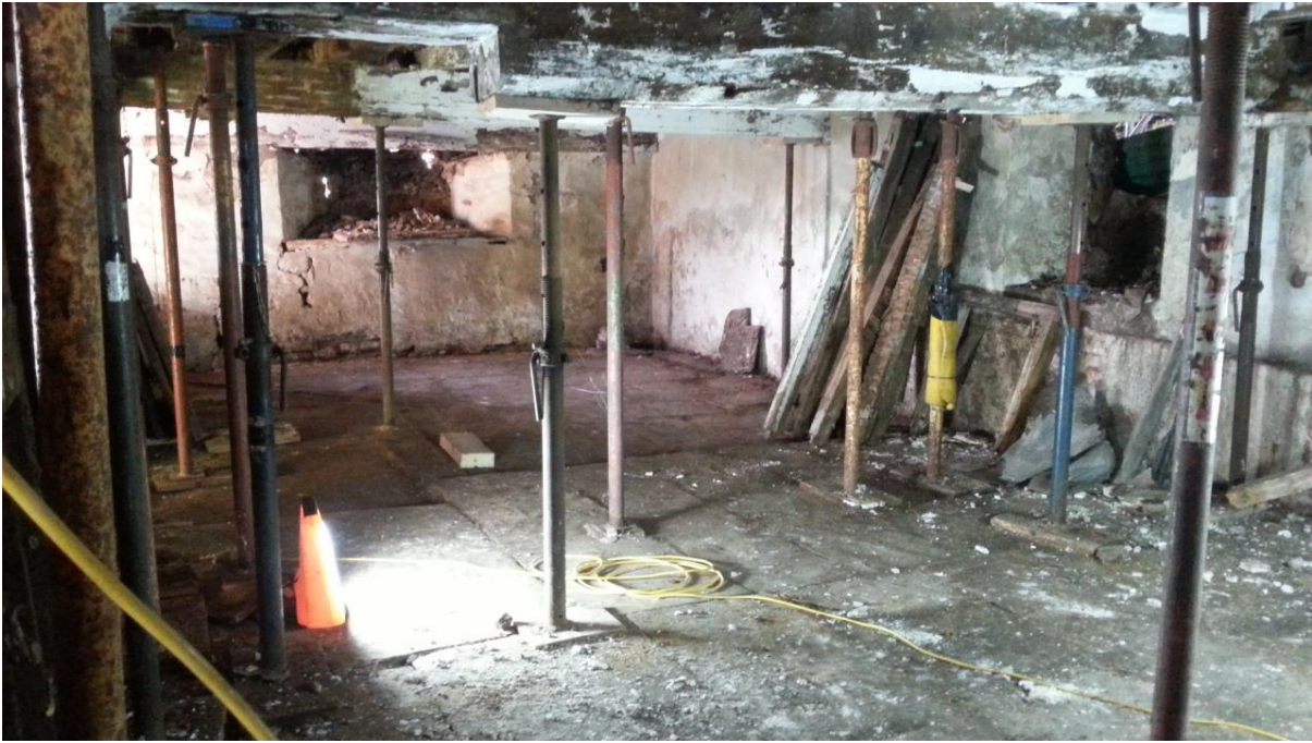
The ground floor of the solar range stripped out, looking south. The ceilings were so low that at some stage a doorhead had been hacked out of the crossbeam (top left). The thickness of the walls is apparent in the window embrasures.
