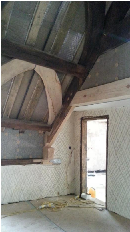
June 2017. Insulation of the underside of the hall roof going in, timber repairs and a first scratch coat of lime render on the walls. Through this door into the solar, plaster repairs are underway to the ceiling, using fibred lime plaster sheets across which the finger moulding can be dragged.
