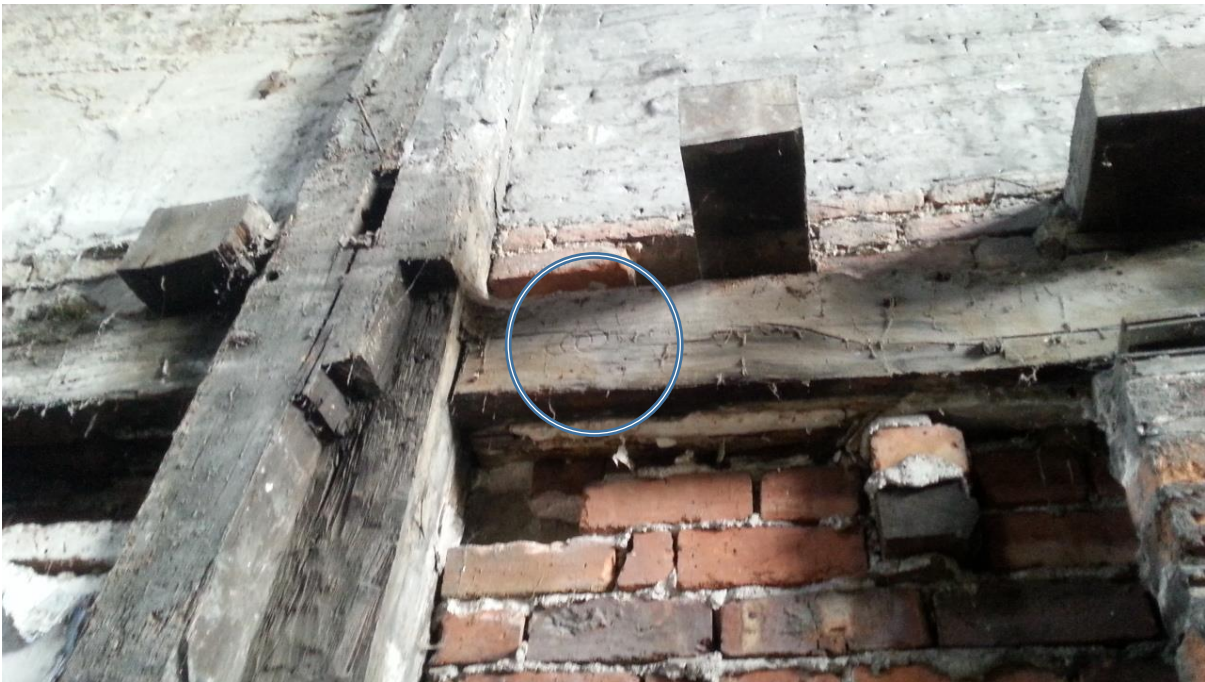
Llwyn Celyn's timbers hold various markings that do not seem to relate to the carpenter's setting out of the building. They may be apotropaic marks, to ward off evil spirits – or they may be someone's idle doodle!
