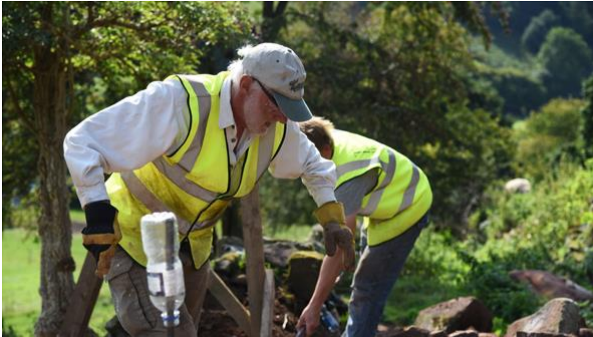
The perimeter drystone wall was continuing its march downhill along an ancient trackway.
