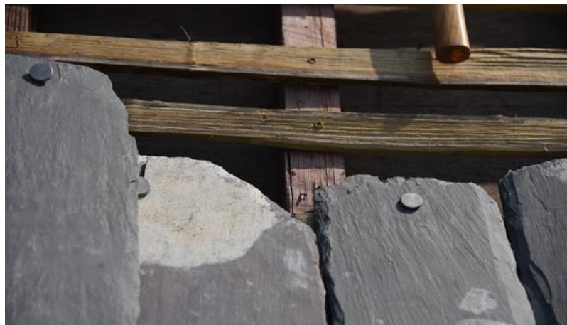
Pegged slates hung over laths
