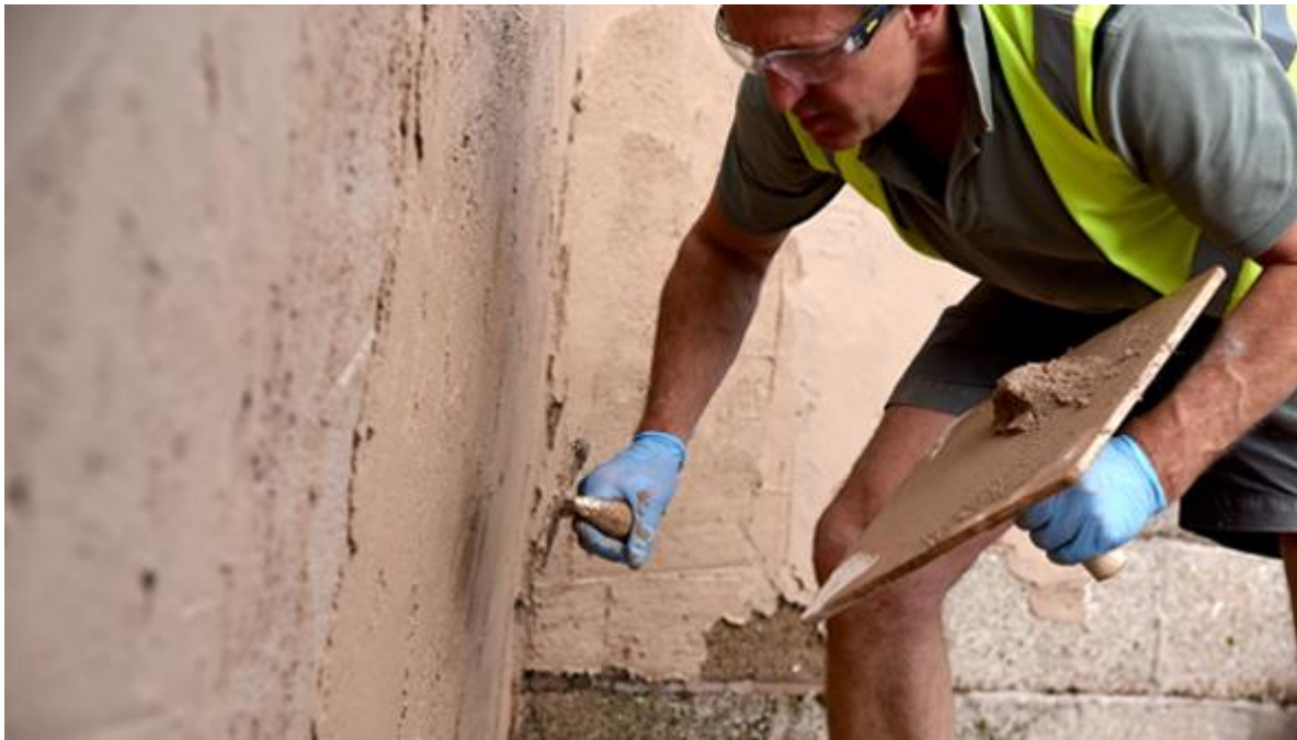
Nigel Jervis from Ty Mawr demonstrates the art of lime plastering.
