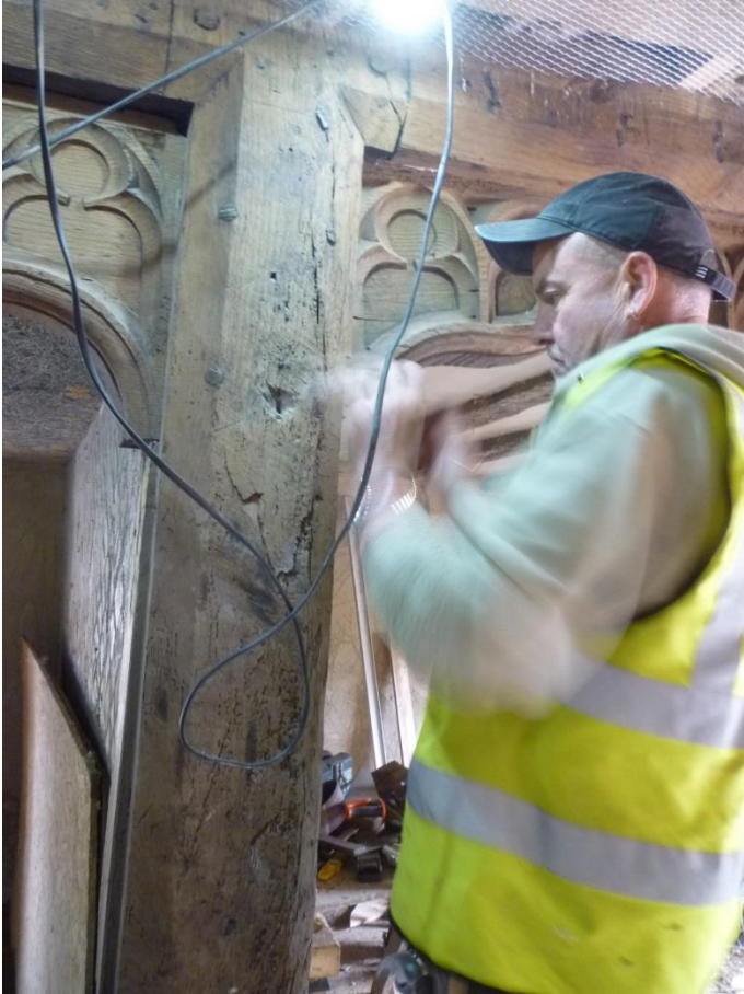
Much of the joinery on the project was done by Simon, here chiseling out the missing point of a spandrel.
