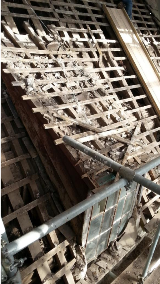
Autumn 2016. The front dormer stripped.
