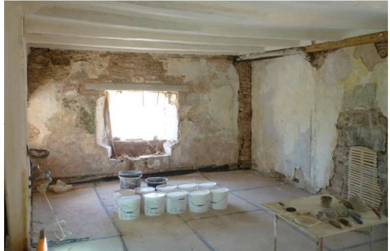
June 2017. Insulation of the underside of the hall roof going in, timber repairs and a first scratch coat of lime render on the walls. Through this door into the solar, plaster repairs are underway to the ceiling, using fibred lime plaster sheets across which the finger moulding can be dragged.
