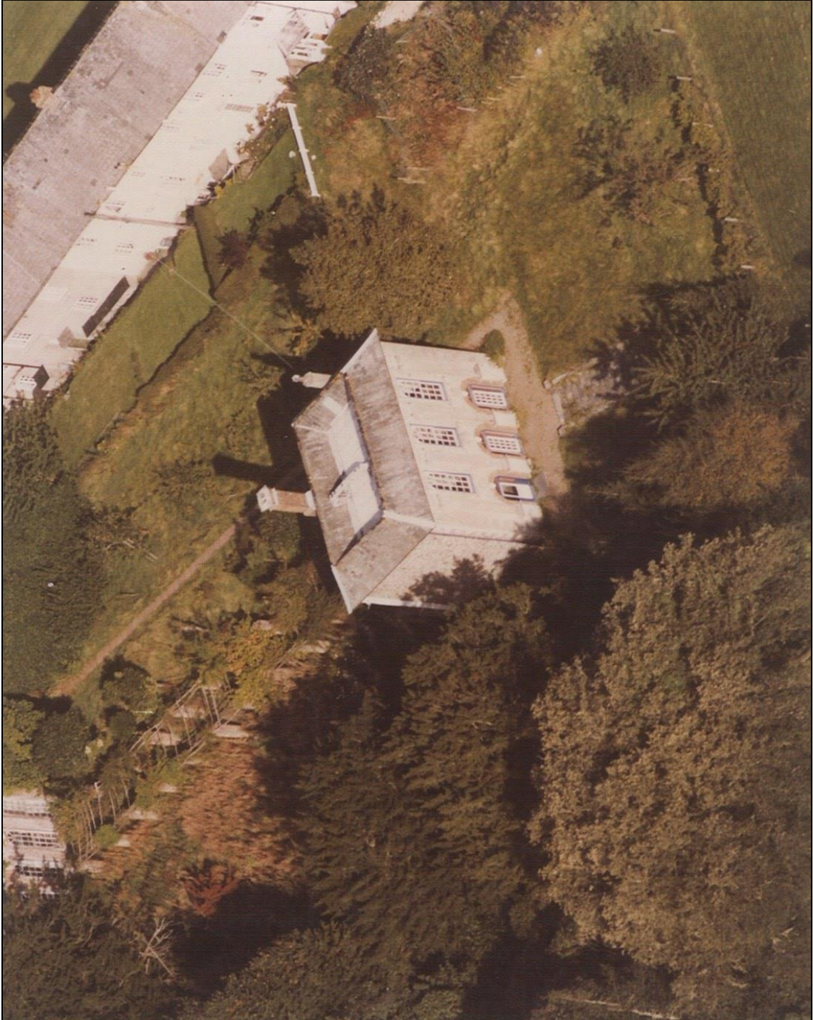
View of The Library 1978, showing the roof put on in 1870.
