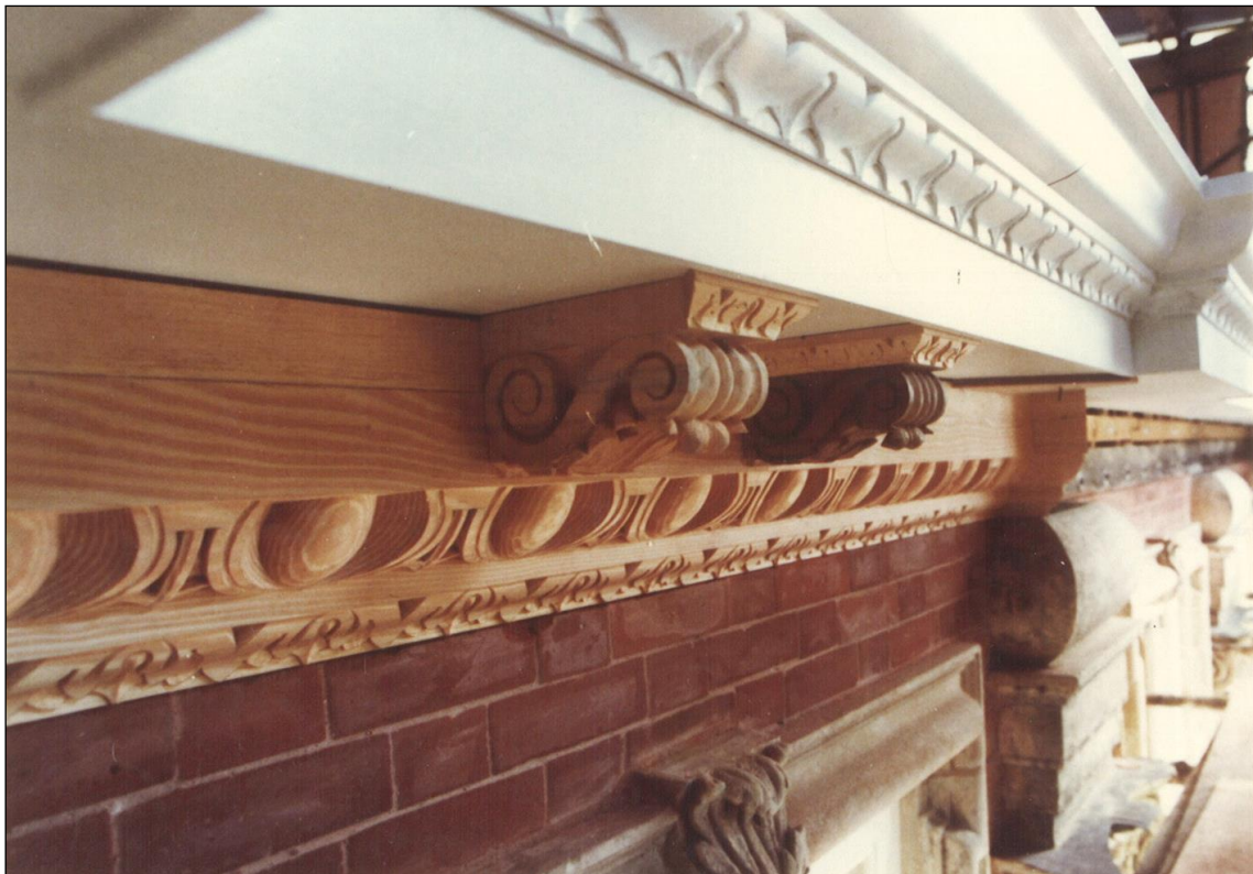
The modillion blocks being fixed in position
