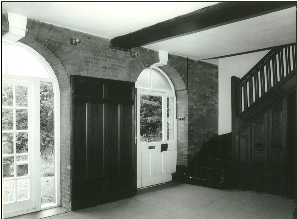
The stairs and panelling may date from 1870, or more probably from c.1945 when The Library was made into a house, using materials salvaged from the main house. The position of the original stairs is unknown.
