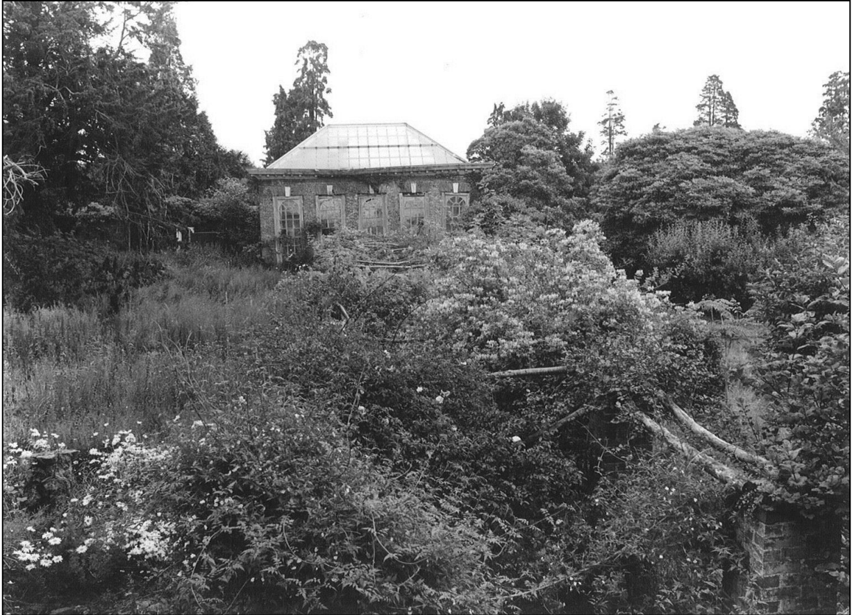
The Orangery in 1978, with the collapsing pergola running between it and The Library
