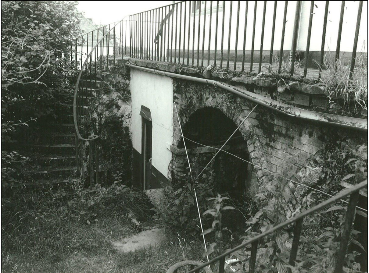
The balcony and steps built against the back of The Library, cutting across the original arch of the loggia, which was uncovered in 1980.
