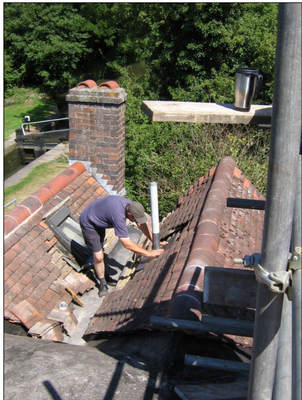
Repairing the bathroom roof.
