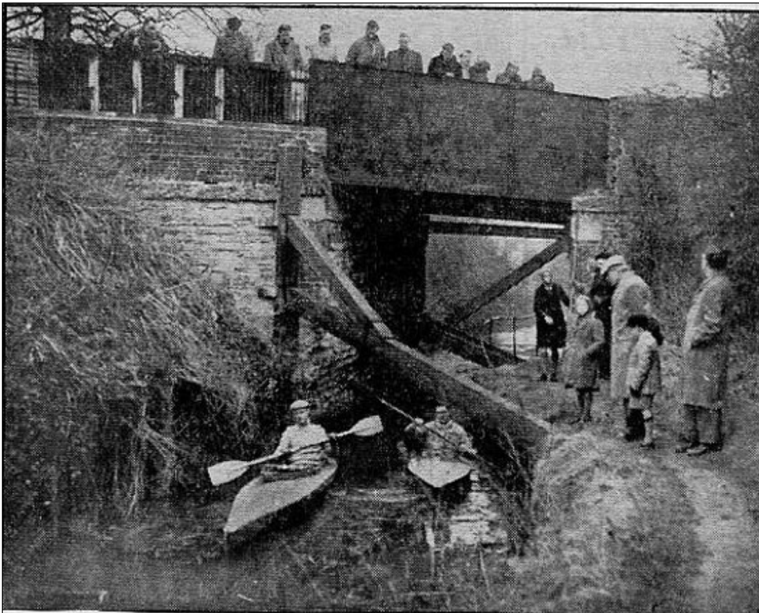
The bridge at Feather Bed Lane at Wilmcote in March 1958, shored up with baulks of timber and passable only to canoeists. It was due to the cost of repairing this bridge that the county council applied for the canal to be abandoned. (SCS)
