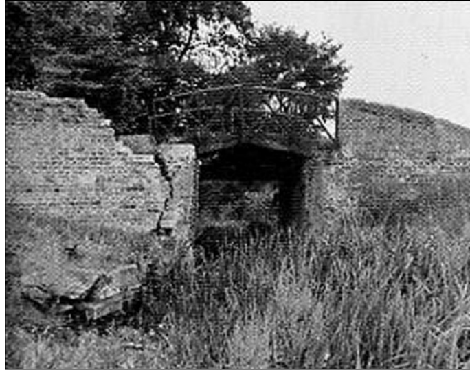
Derelict split bridge above Lock 48, 1962 (SCS)
