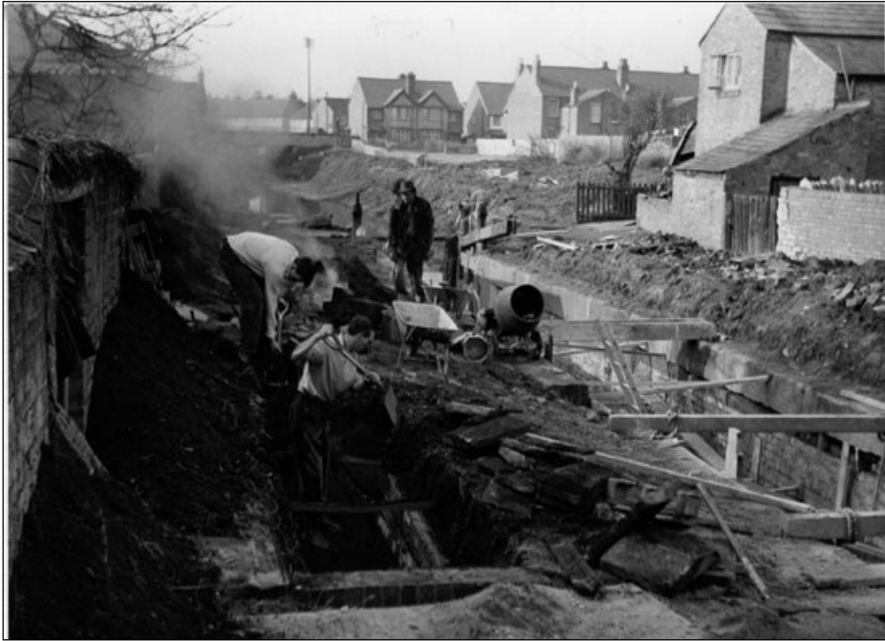
Digging out a collapsed culvert at Lock 54, date unknown (SCS).
