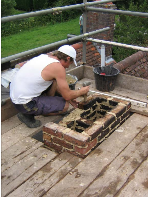
Rebuilding the unstable chimney stack.
