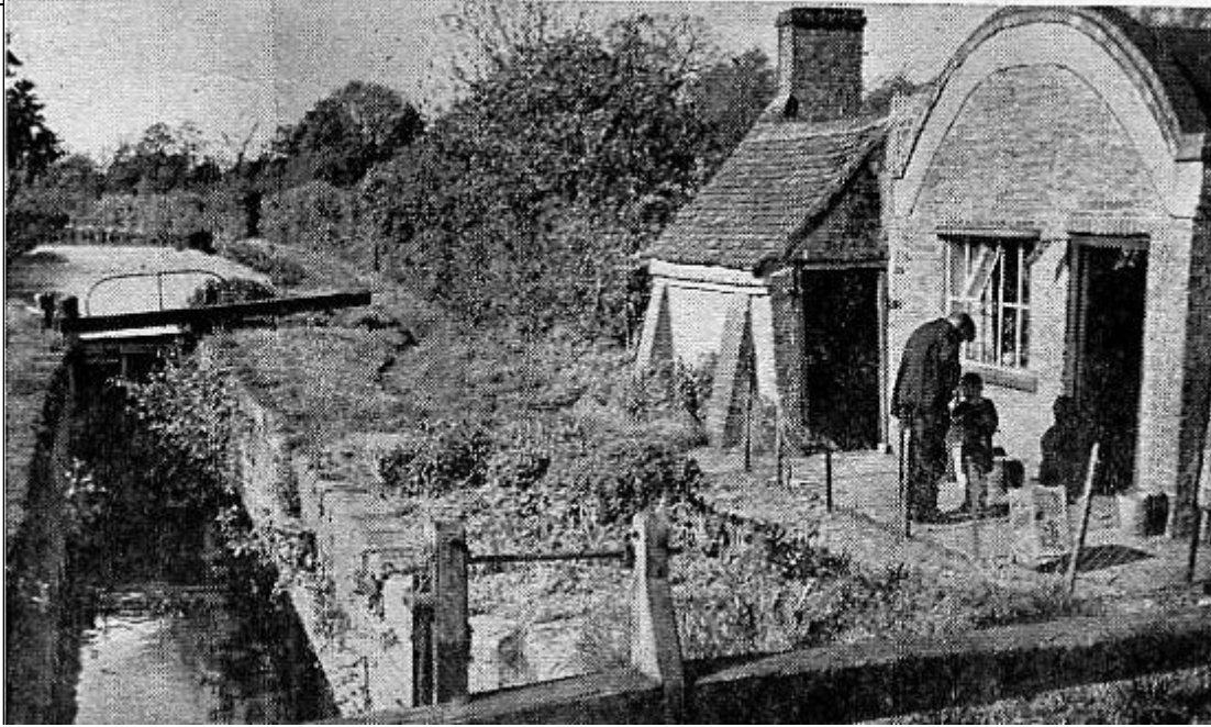
Lengthsman's Cottage (then known as the Lock House) in 1953 when the canal had passed into state ownership and was in the depths of decline. The adult figure is Ned Taylor's father, Edward. The exterior of the cottage at this date does not appear to be painted, but note the 'eyebrow'. (SCS)
