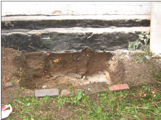
The cottage has no foundations. It is thought the cottages simply sat on timber floor plates, on a layer of the same puddled clay used to line the canal.
