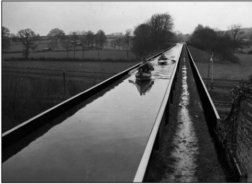
Two canoes crossing Edstone aqueduct in March 1957. The licence issued for the leading canoe proved the navigation of the canal. Edstone is the longest cast iron aqueduct in England. (SCS)
