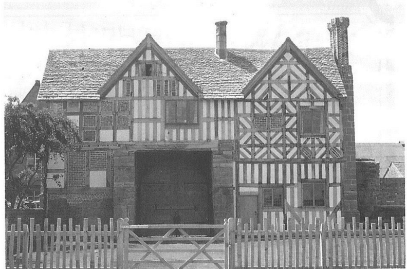
The east elevation after repairs were complete.
