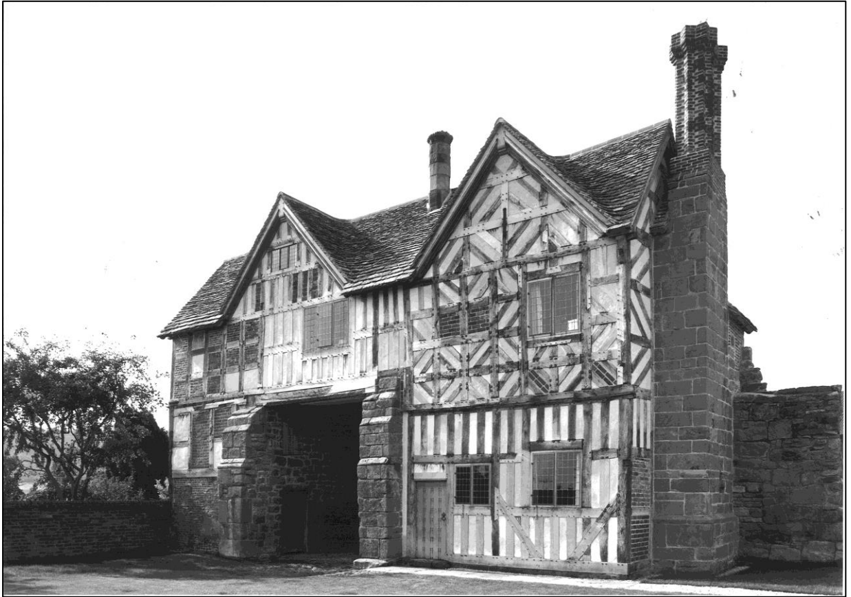
The repairs completed
