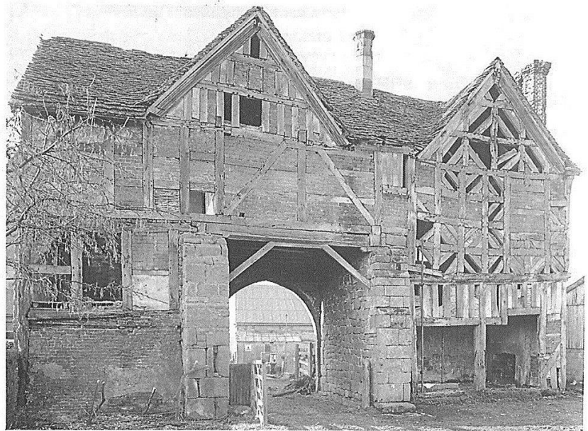
The east elevation before work began
