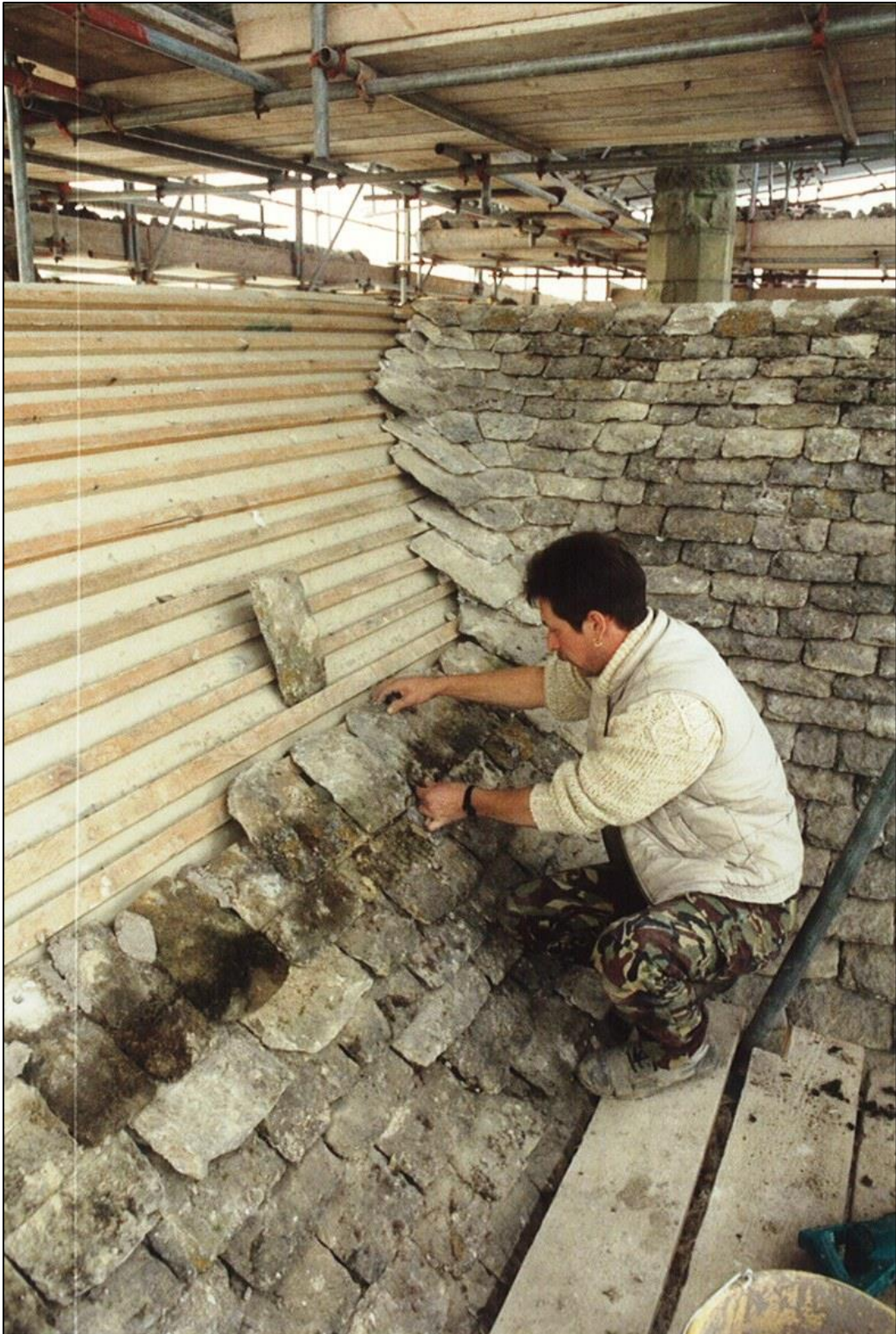
Relaying the Harnage stone slates in carefully graded diminishing courses
