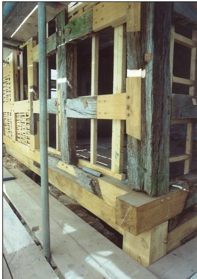
Repairs to the timber-frame
