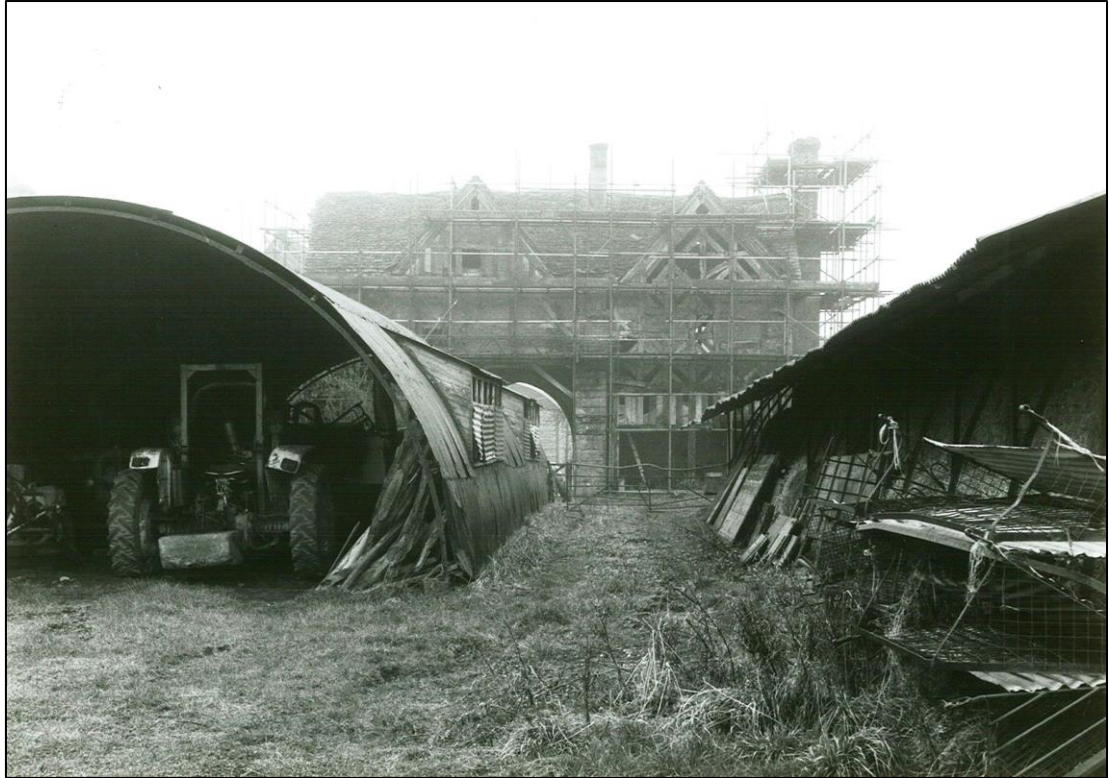
View from the east before repair
