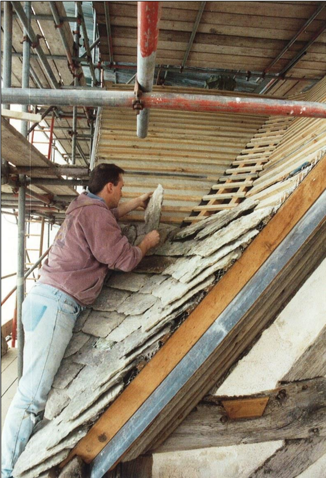
Positioning the re-laid Harnage stone slates for a roof valley
