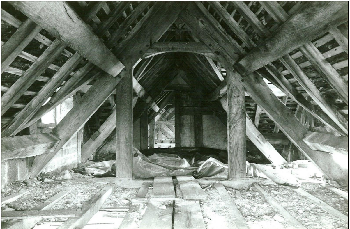
The roof trusses
