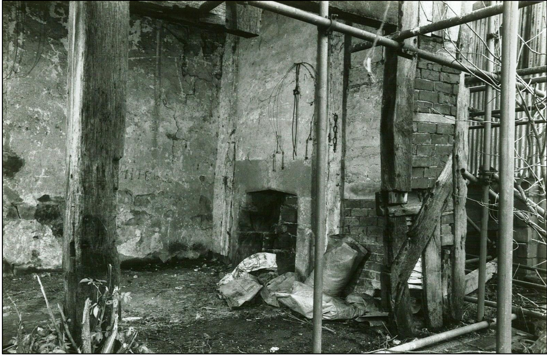
The ground floor, north end.
