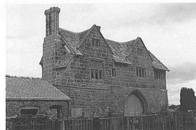
The repaired west elevation.
