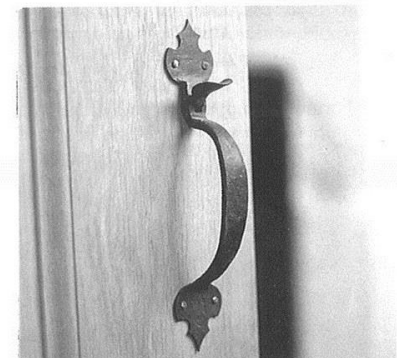
Iron was used for making new latches, hinges, bolts etc. We had to resort to the use of mild steel only when making the hinges for the main gates.
