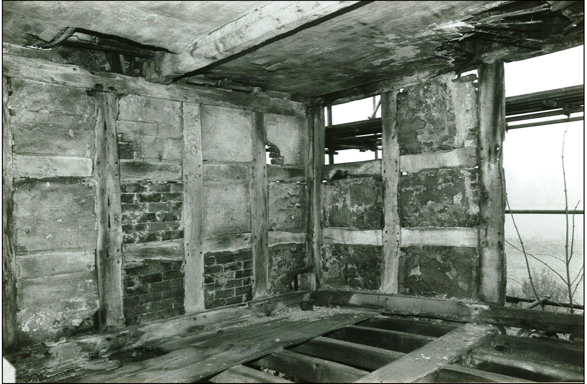
The first floor, south end
