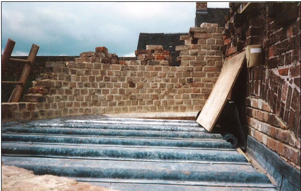
Lead roof on the southern bow.
