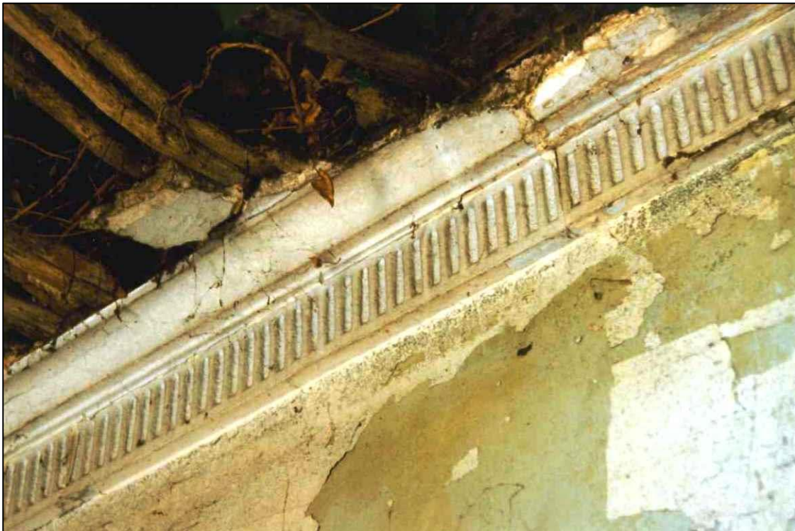
A fragment of the cornice. Small fragments were refixed where possible and the rest was copied by a specialist plastering firm.
