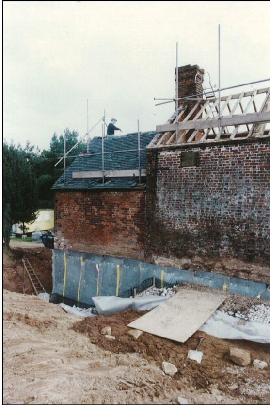
Damp proofing on the west side.
