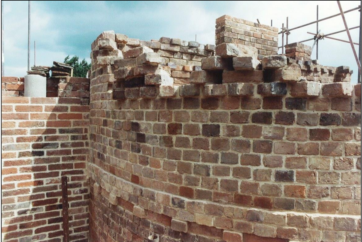
New tuck pointing on the parapet.
