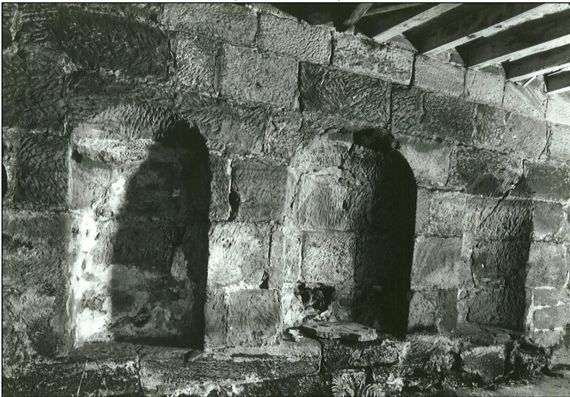
The open terrace below the east range, once enclosed by a ceiling of the floor of a range of rooms which have been demolished.
