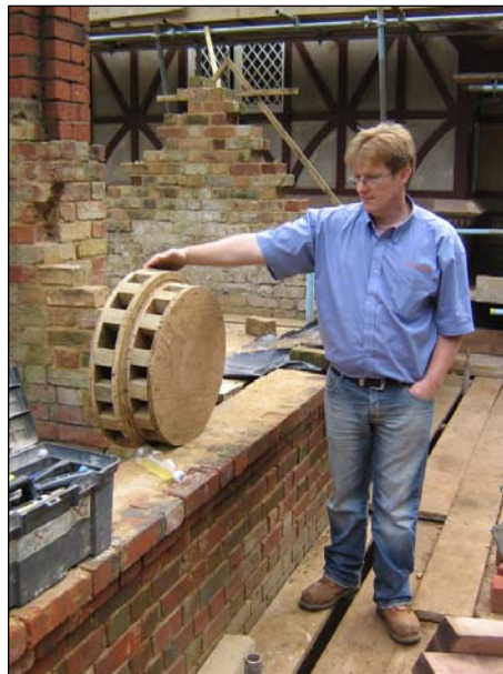
The wooden former used to create the 'bullseye' window in the sitting house.
