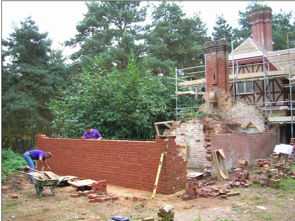
Rebuilding the Sitting House according to John Usher's plans.
