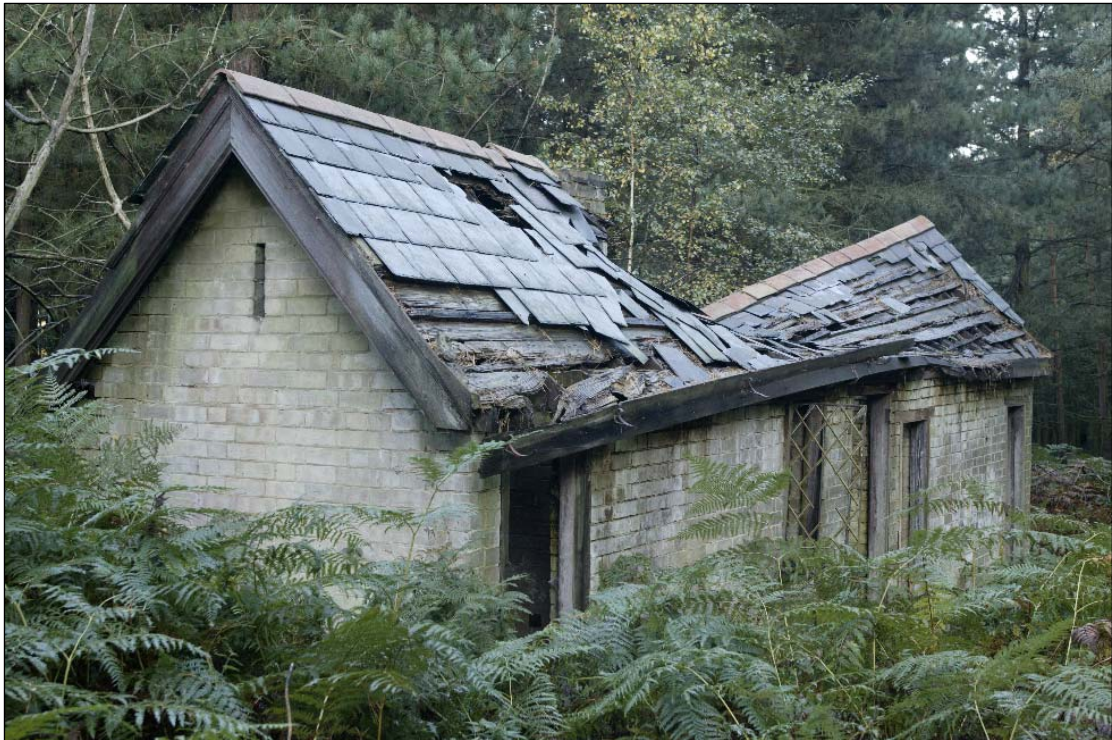
The kennels before work began.
