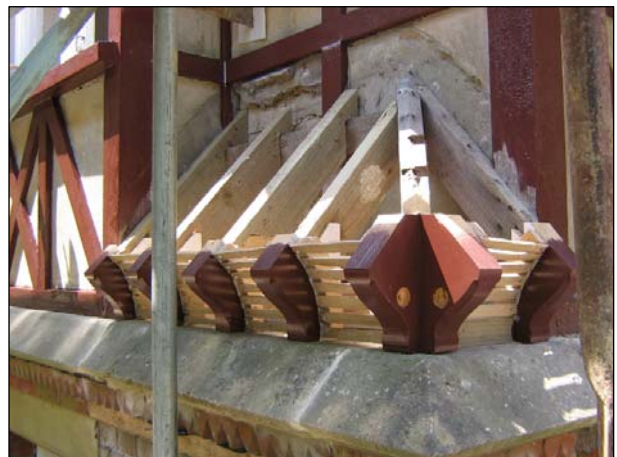
The painstaking re-instatement of the miniature 'hips' at the corners
