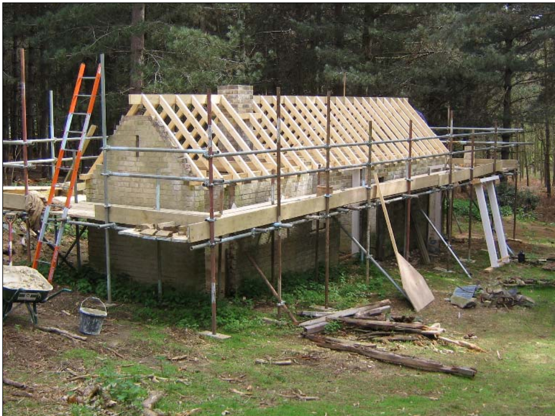
Work to the kennels underway.
