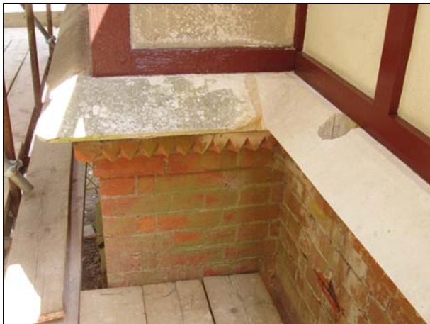
Repaired stone drip mould awaiting its downpipe.
