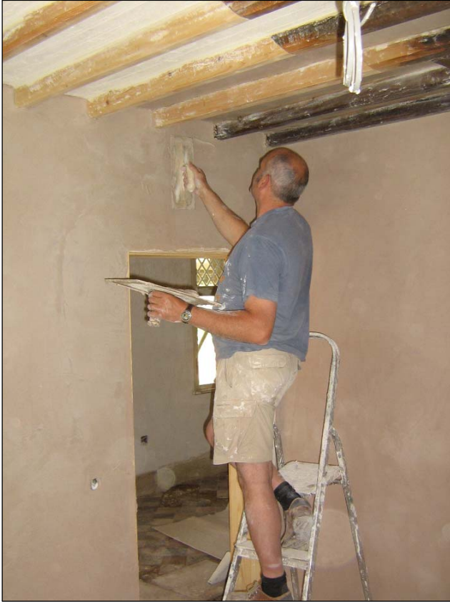
Replastering the sitting room. Note the repairs to the rotten joists.
