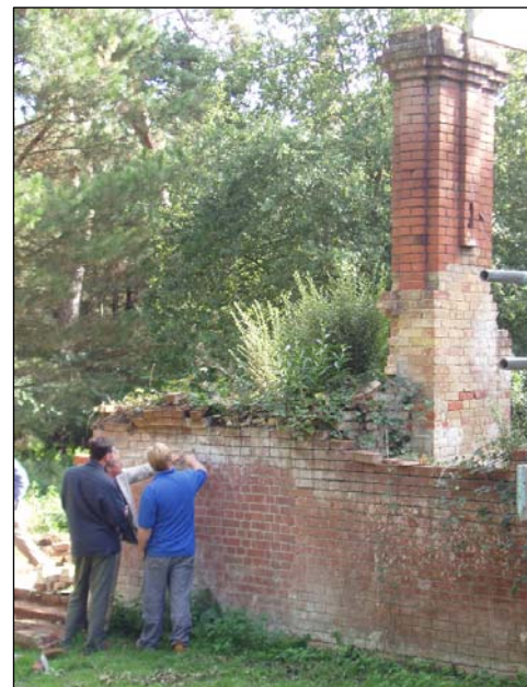
Discussing re-pointing samples.
