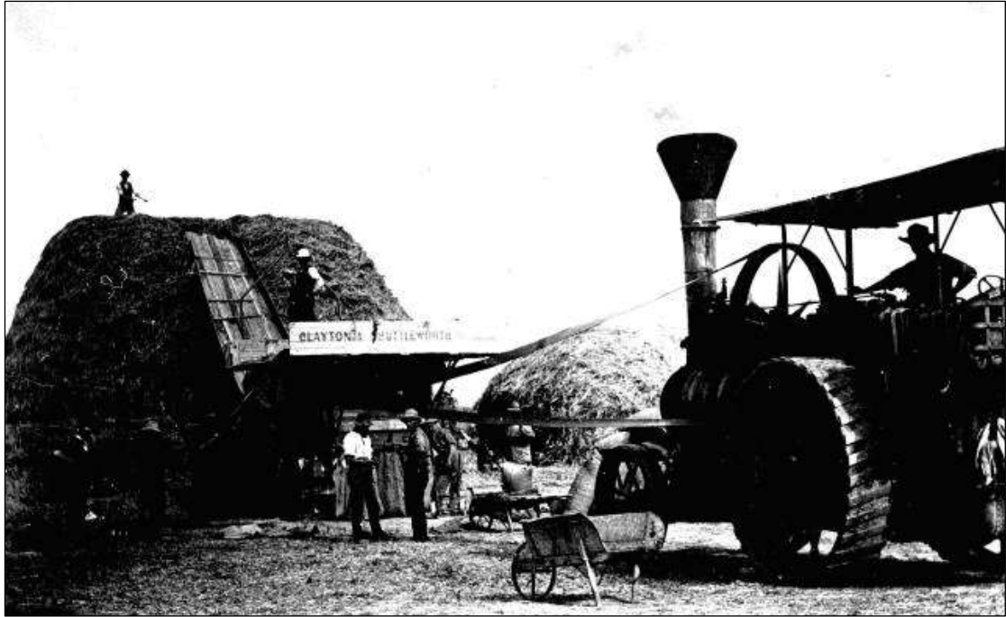
Clayton Shuttleworth threshers in operation in Australia at the turn of the century, powered by the traction engine.
