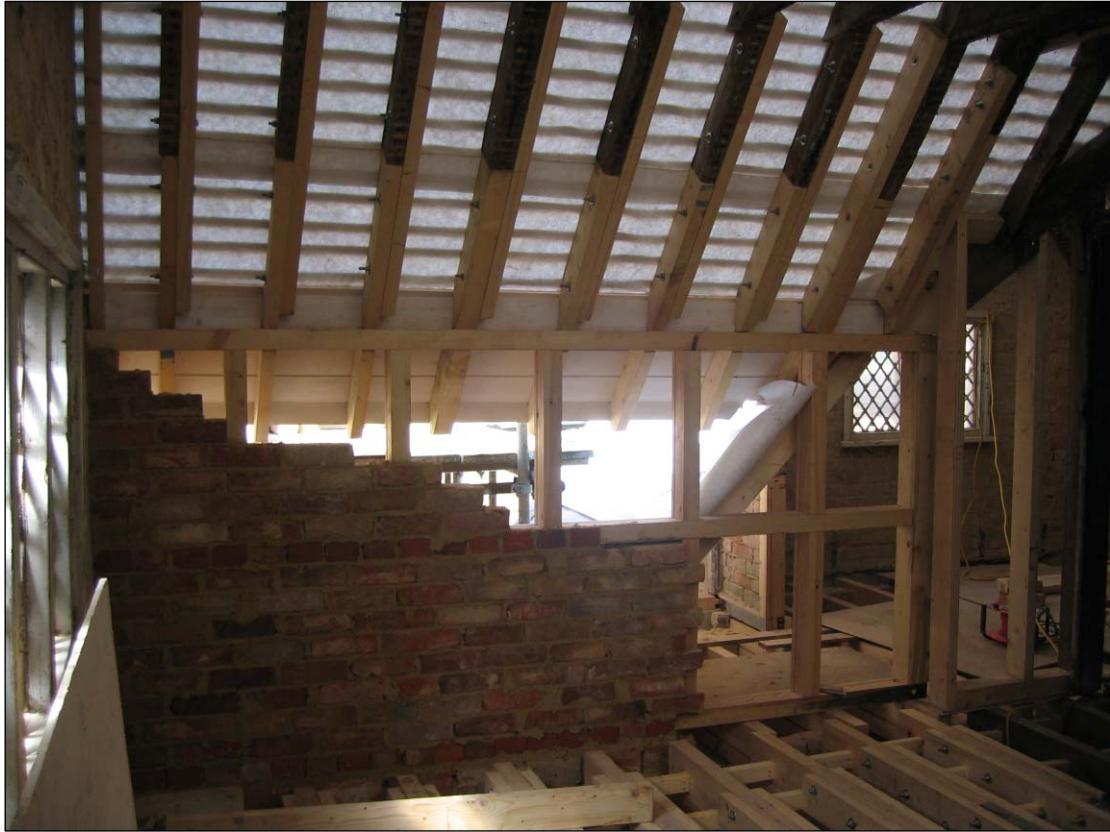
Repairs to the West bedroom.
