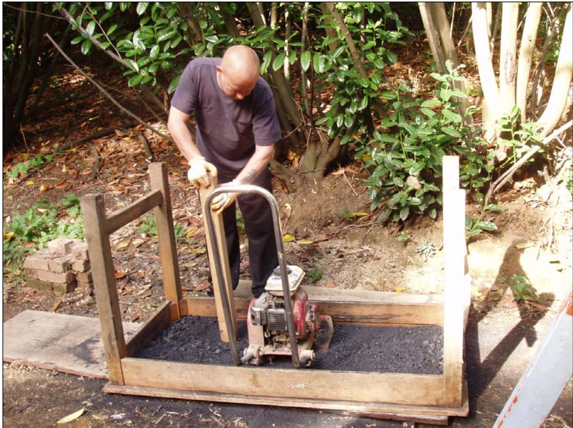
Crushing charcoal in an upturned table to colour the mortar.
