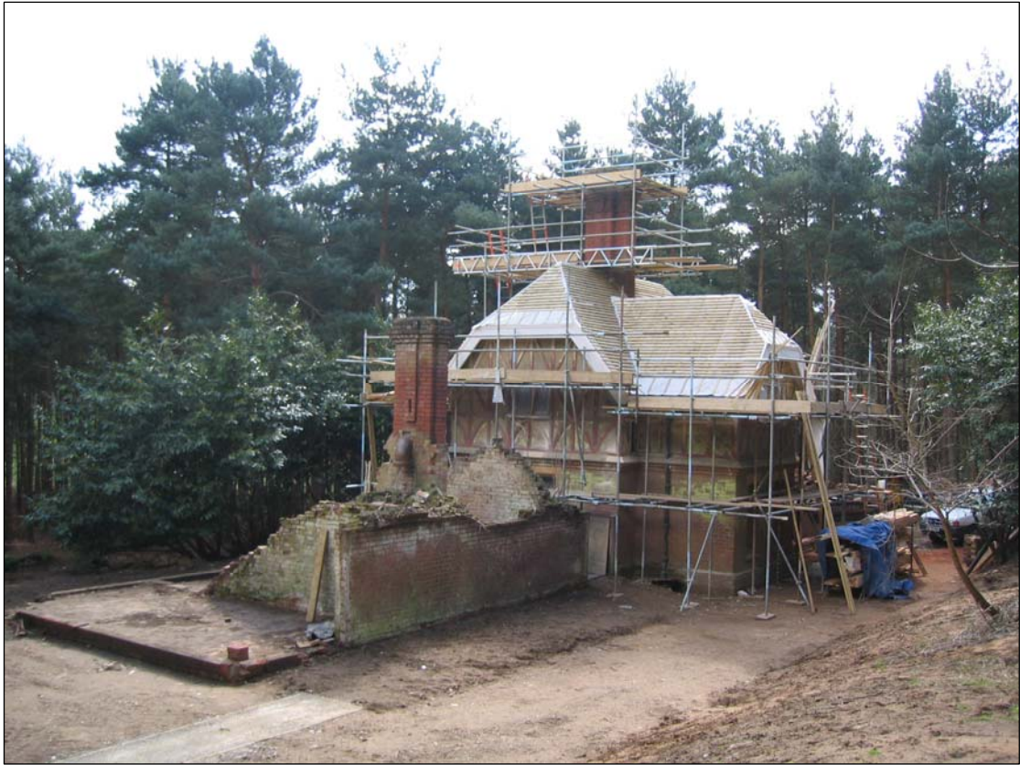
Repairs to the roof and chimneystacks well underway.
