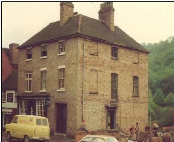
The building before and during restoration showing the blocked up windows and irregular glazing.
