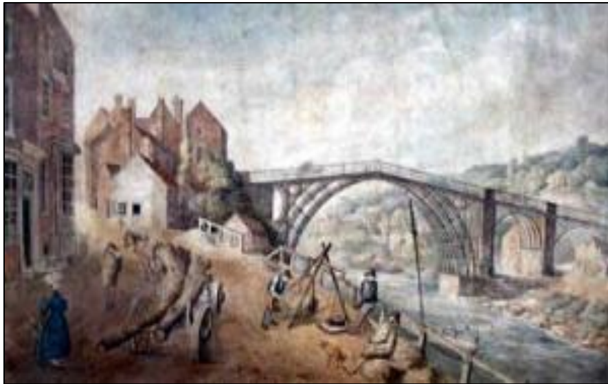
A heavily laden cart makes its way up Tontine Hill and three men weigh wool on the north bank. Iron land arches were built on the south side of the river in 1821 to reduce the weight of the abutment.
