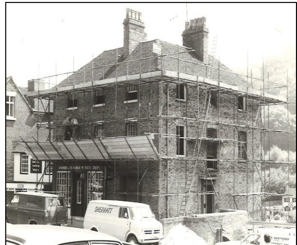
The building before and during restoration showing the blocked up windows and irregular glazing.
