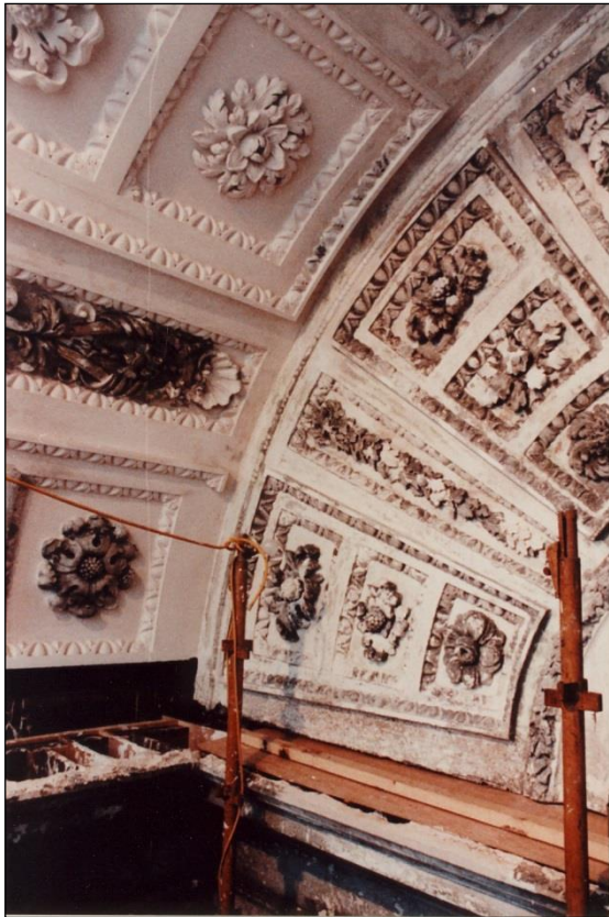
New plasterwork can be distinguished from old by its colour. One whole panel (on the left) had perished completely and had to be renewed.
