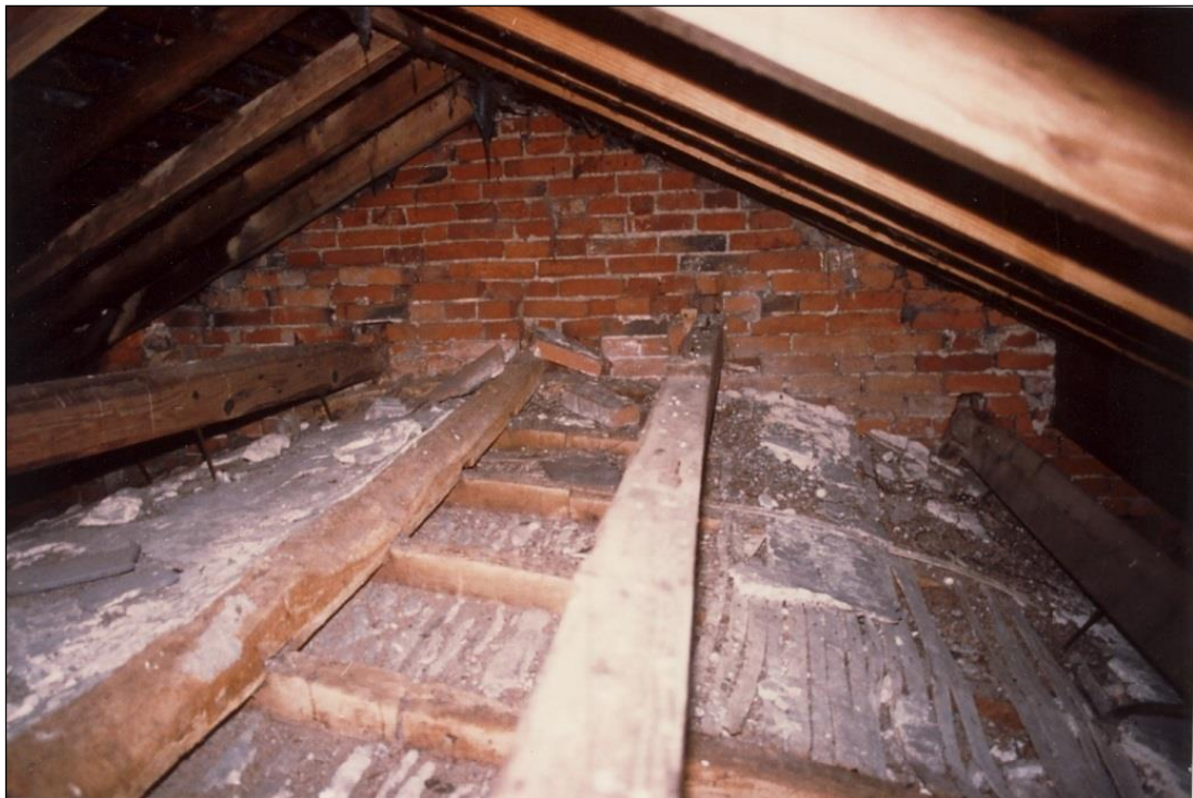
Repaired purlins and new steel ties in the roof structure.
