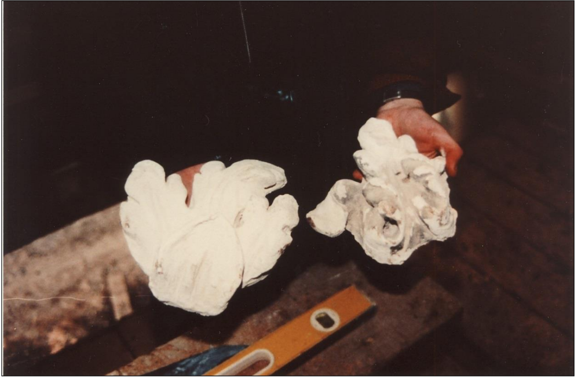
Repaired fragments of plaster, ready for refixing.
