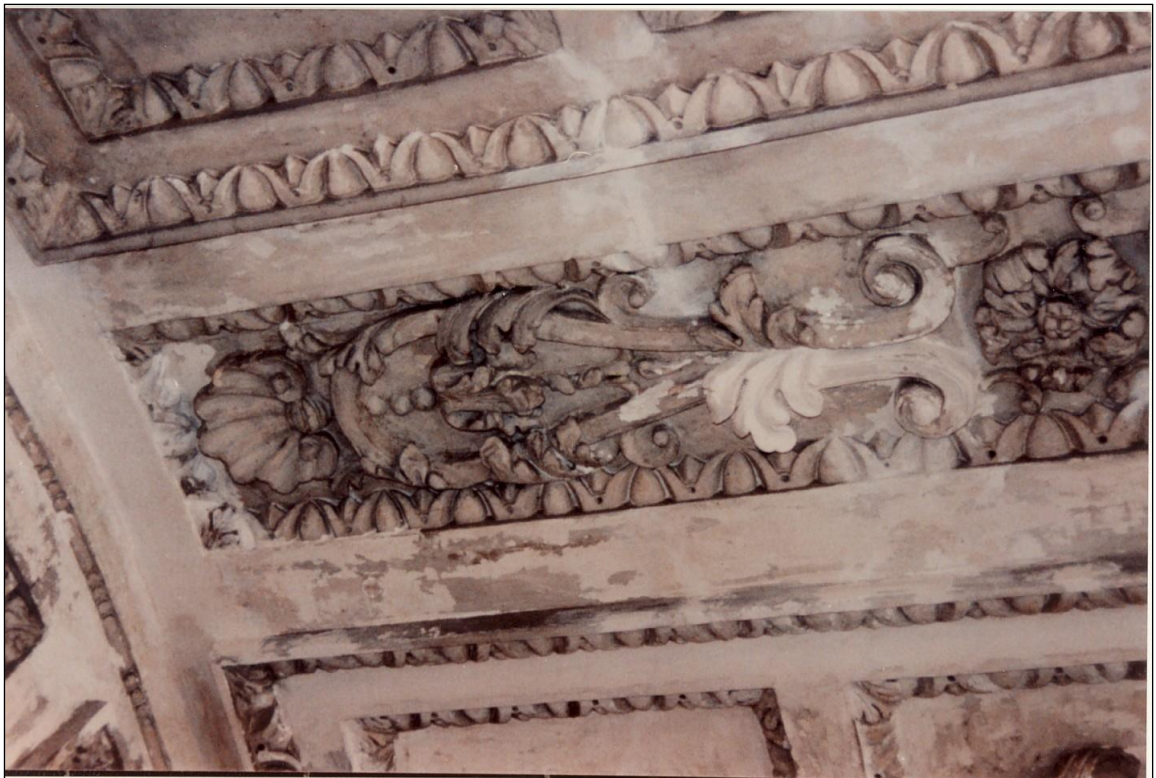
Typical plaster repair.
