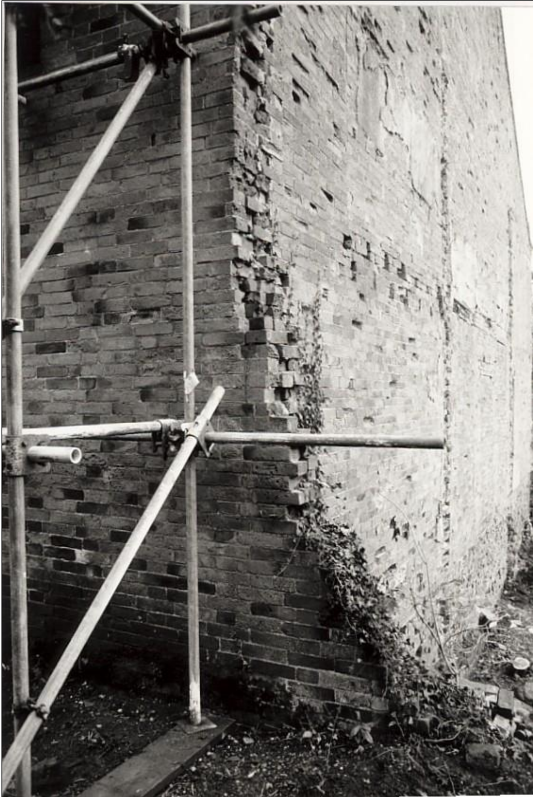
6. The northwest corner, showing that the side walls of the front portion of the pavilion formerly continued in an unbroken line to the far rear corners of the original structure.
