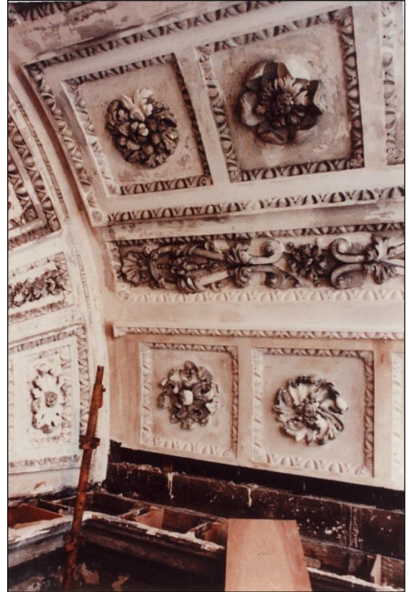
New plasterwork can be distinguished from old by its colour. One whole panel (on the left) had perished completely and had to be renewed.
