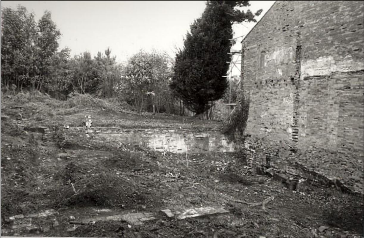
6. Looking north towards the side revetment wall of the former basement pit.
