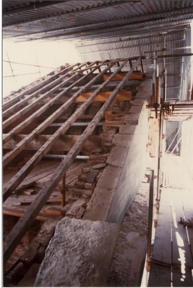
Repaired purlins and new steel ties in the roof structure.
