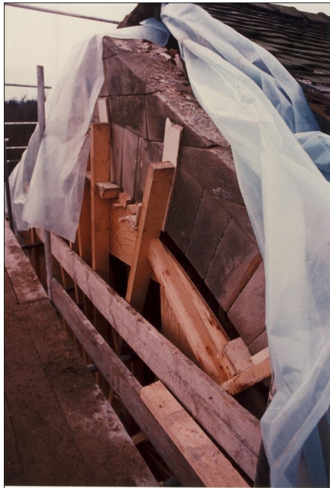
The template used to support the arch while the roof and pediment were repaired and secured.
