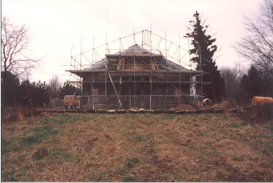
The template used to support the arch while the roof and pediment were repaired and secured.
