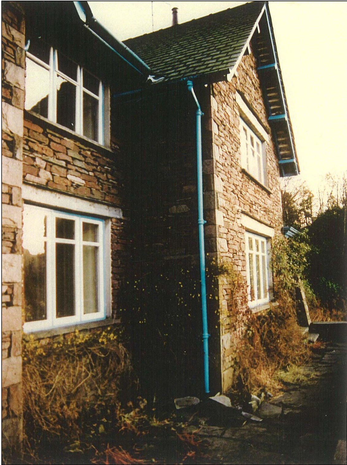
The south west front with blue paint
