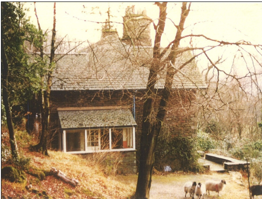
The kitchen extension was removed.
