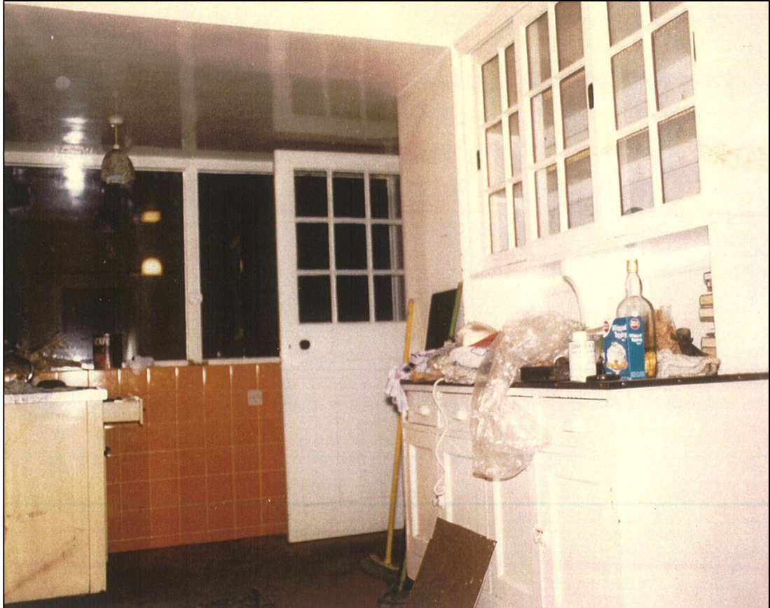
The interior of the kitchen extension. The cupboard is now in the boiler-room.
