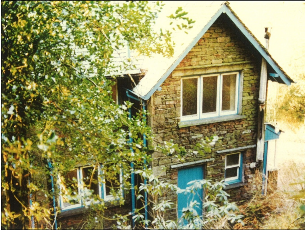
The north east side showing the flue for the oil central heating, now removed, and the blue paint.
