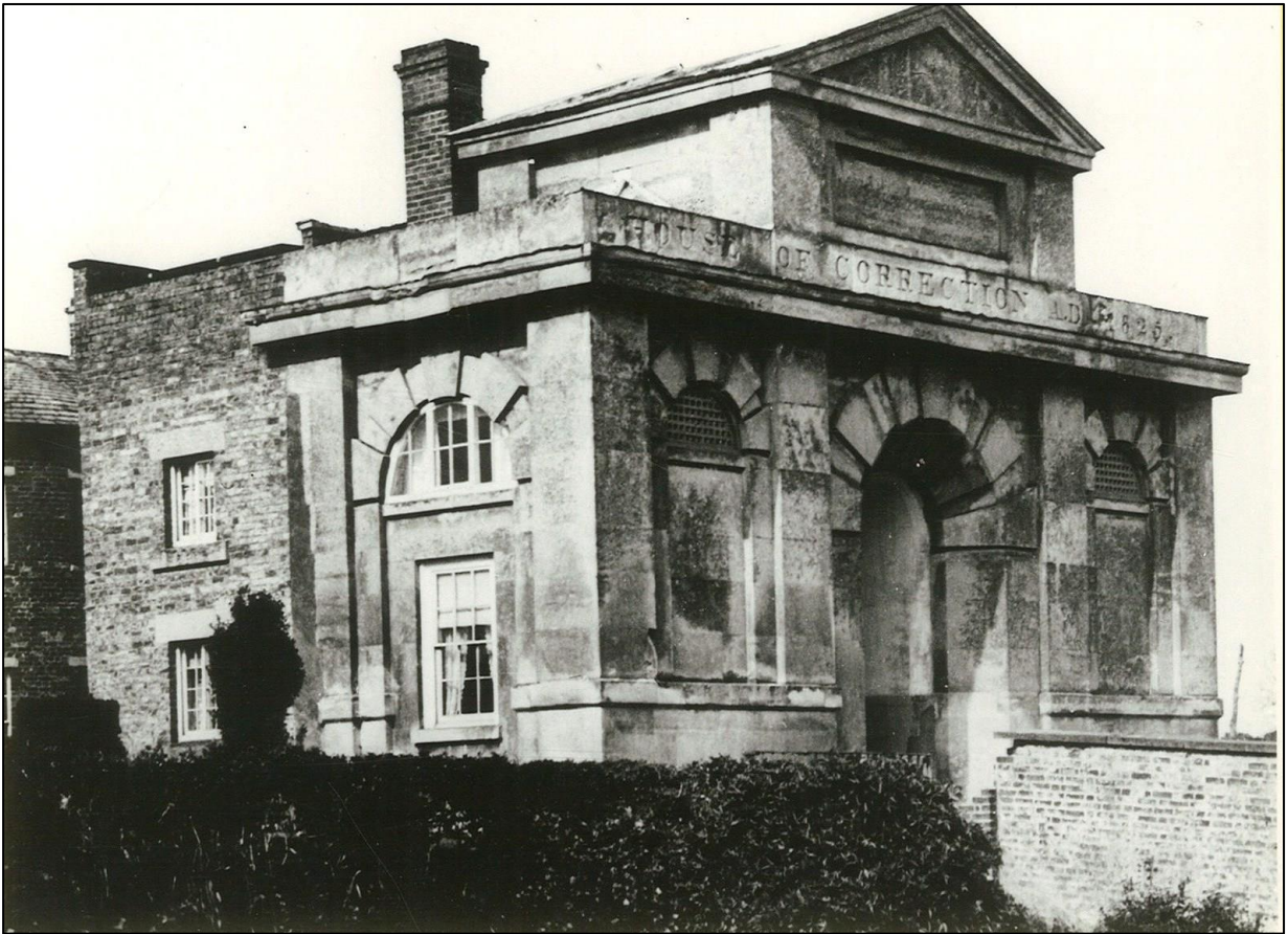
The 1930s brick addition still with the prison buildings behind
