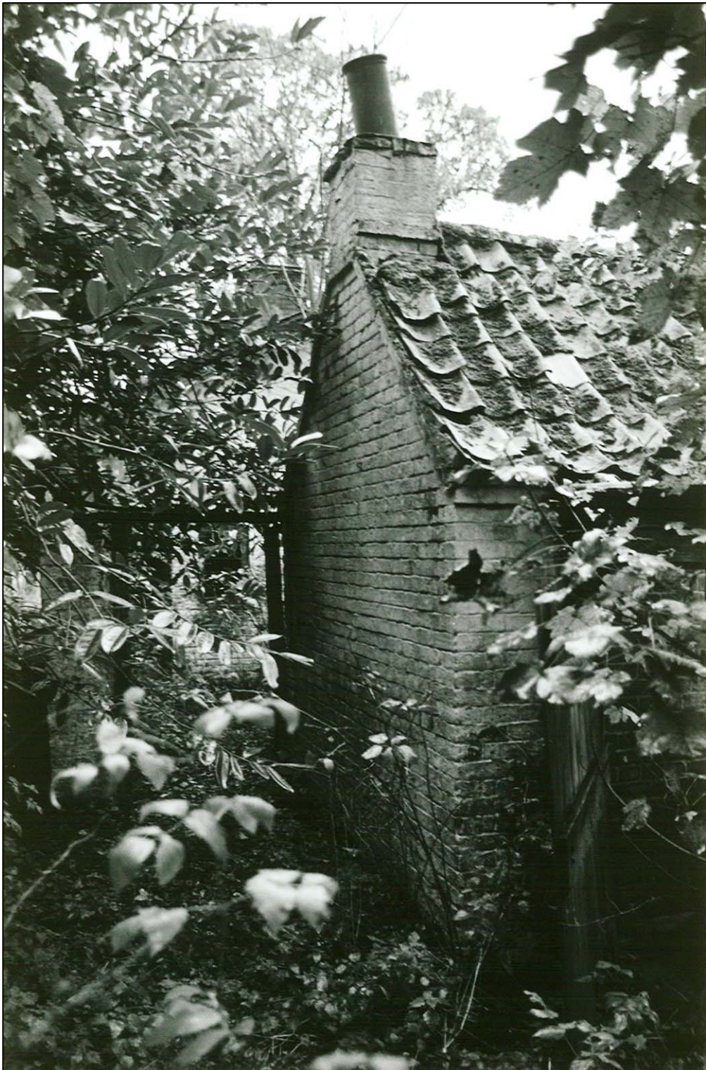
The rear of the wash house
