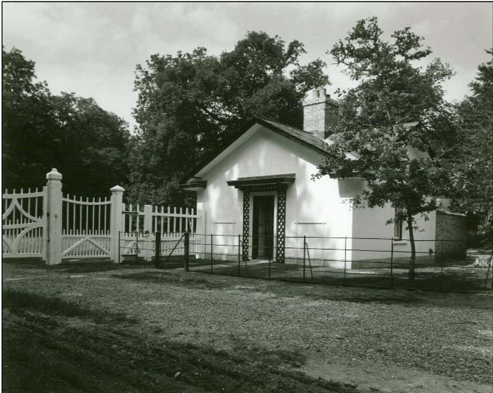
The work completed
