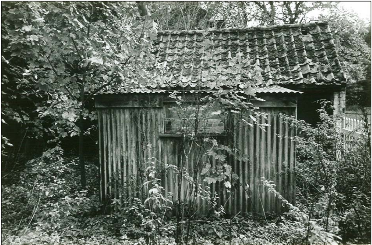
The lean-to wash shed removed
