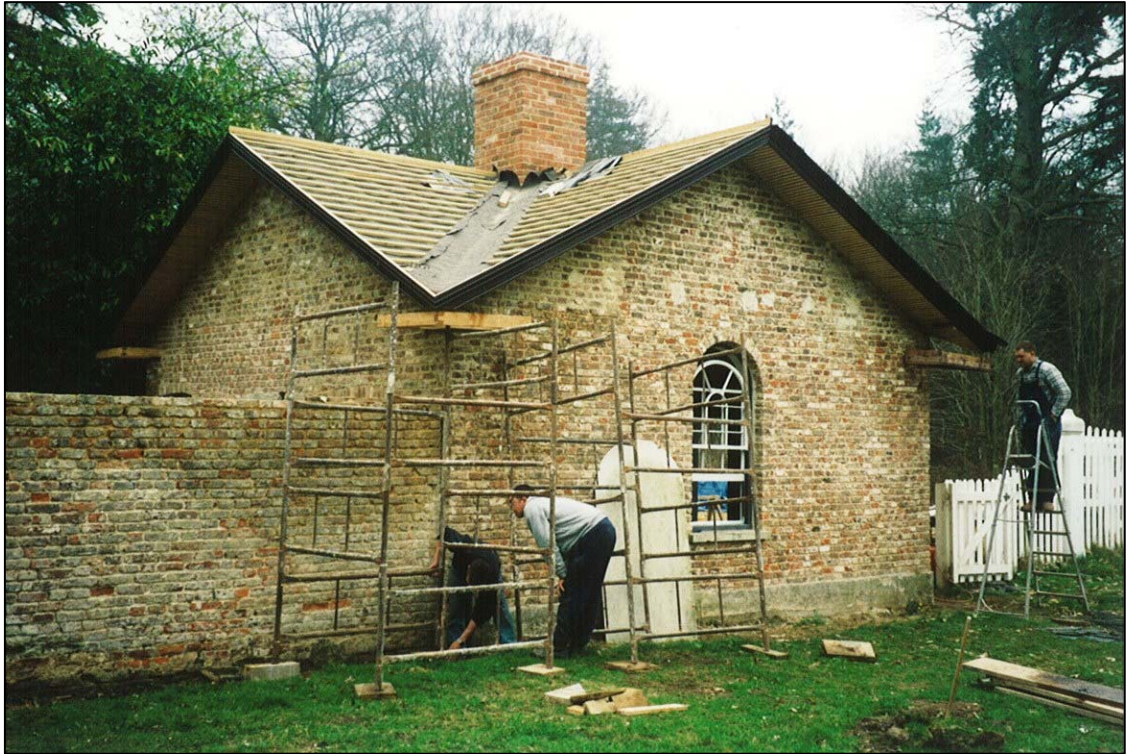
The lodge with the render removed
