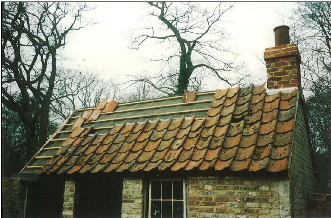
Reroofing the wash house with pantiles
