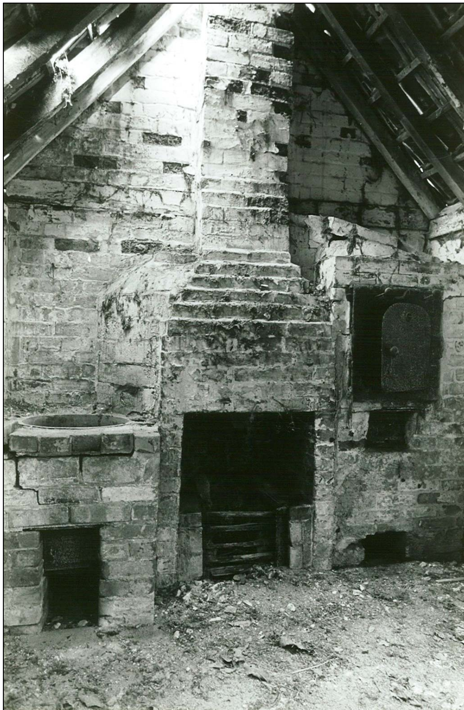
The interior of the wash house
