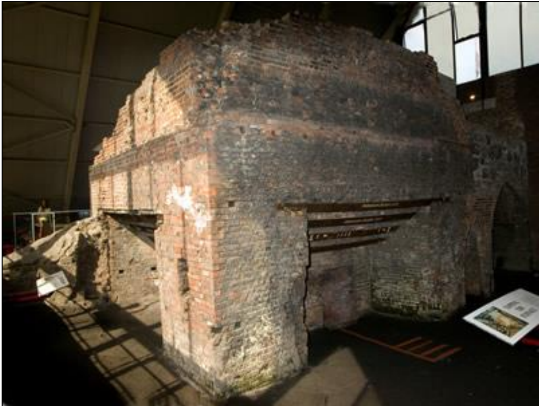
The remains of Abraham Darby's coke-fired blast furnace at Coalbrookdale. By using coke, Darby was able to build taller, and therefore hotter, furnaces.
