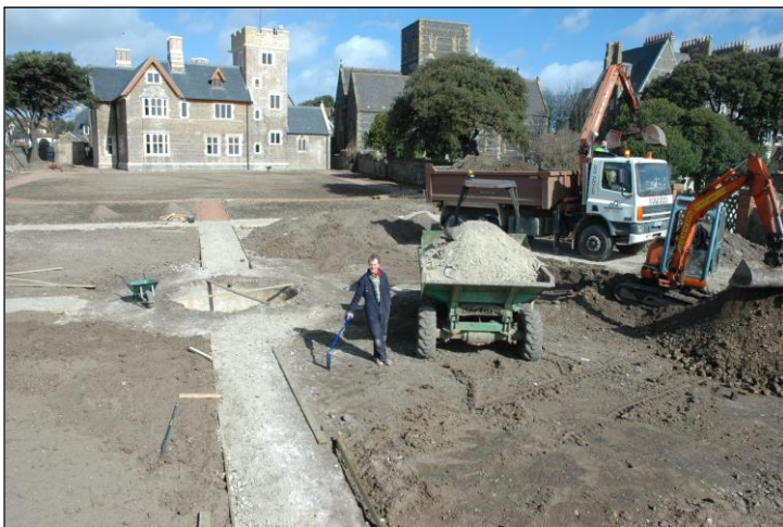
John Evetts (above) and Ian Bolton (right, working on the retaining wall of the viewing mound) spent weeks and much care recovering and laying out the garden through spring 2006. The original, beaten chalk footings for the paths show clearly through the soil.
