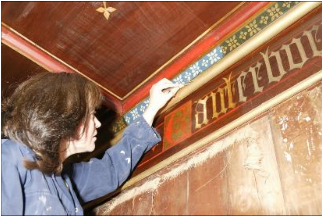
Cleaning the library frieze (July 2004)
