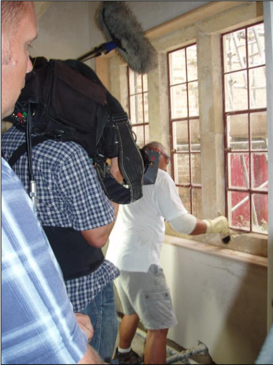
Filming the repair of the kitchen bay, Sept 05.
