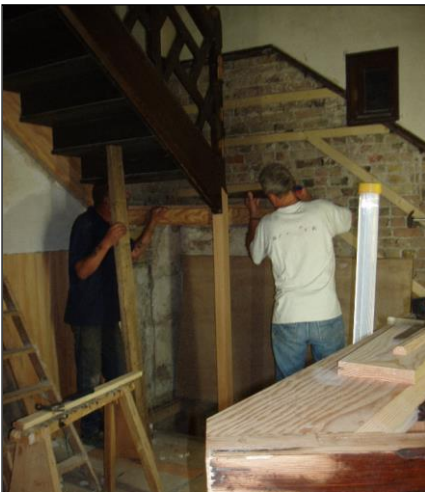
The stairs dismantled and under repair (summer 2005)
