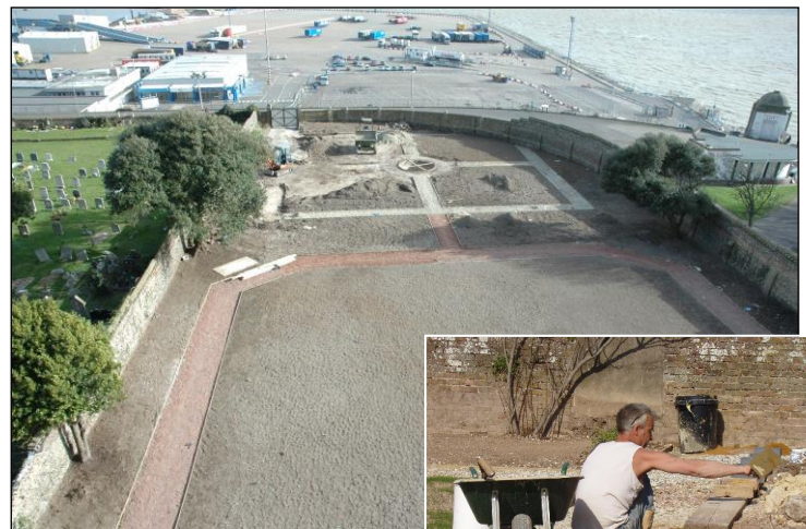
John Evetts (above) and Ian Bolton (right, working on the retaining wall of the viewing mound) spent weeks and much care recovering and laying out the garden through spring 2006. The original, beaten chalk footings for the paths show clearly through the soil.
