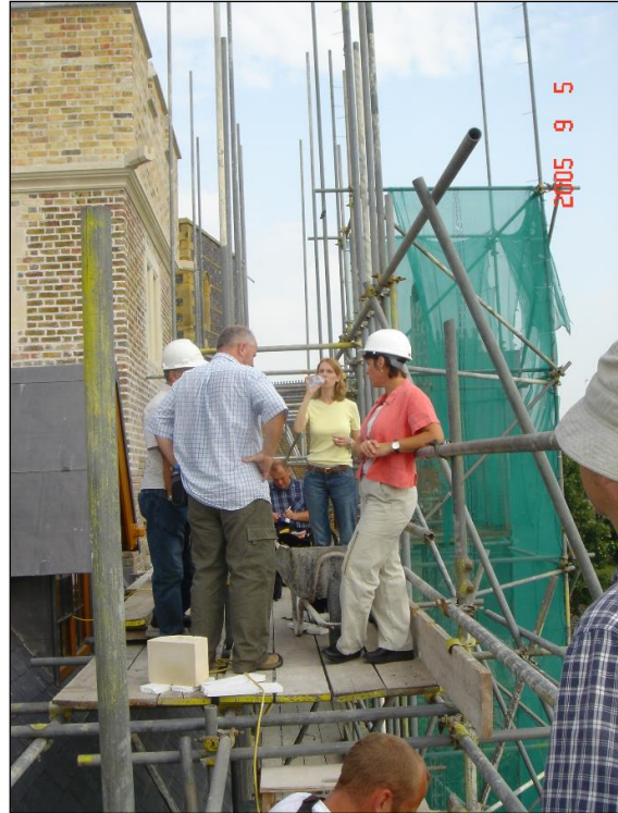
The crew on the scaffolding, at roof level.
