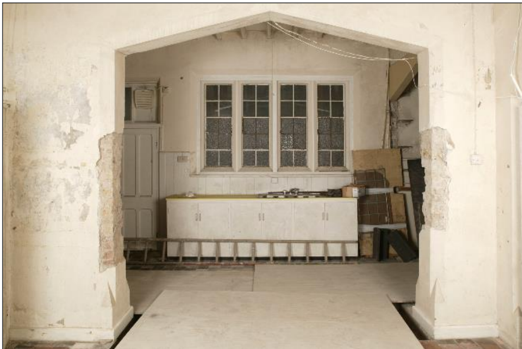
Edward Pugin's kitchen extension before it was taken down.
