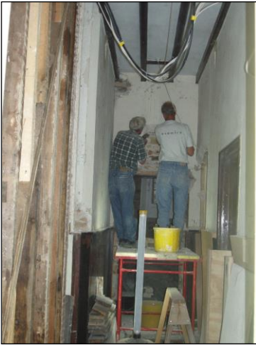
Chasing in electrical cables outside the dining room (August 2004).
