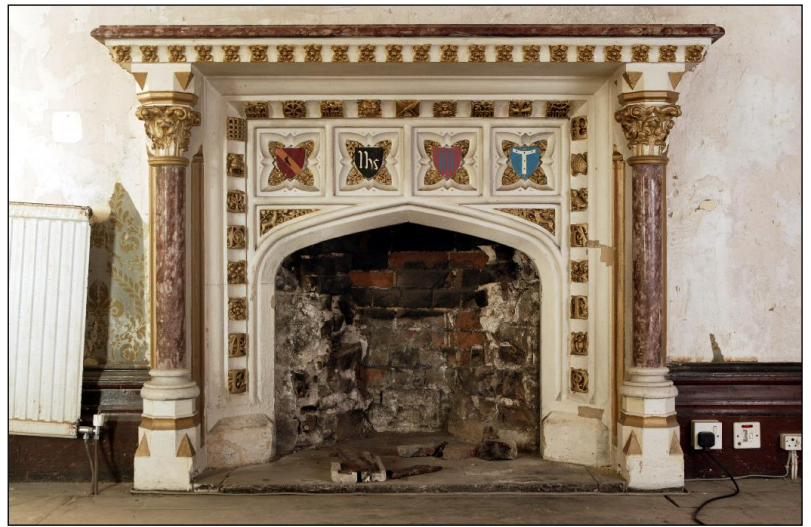
The sitting room fireplace at The Grange before restoration
