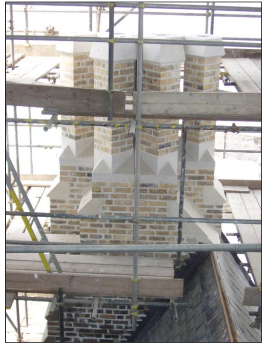
Clockwise from top left: An apprentice working on roof timbers; replacing the window to Pugin's room; one of the new chimney stacks, roof still awaiting the lead flashing; positioning the cross on the chapel roof
