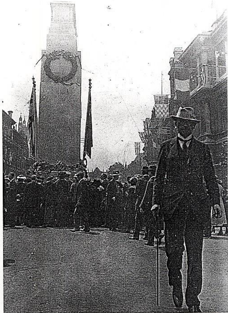
Lutyens at the temporary Cenotaph in Whitehall, which he designed in 1919. It was hastily constructed to be in place for the victory celebrations of July 19
