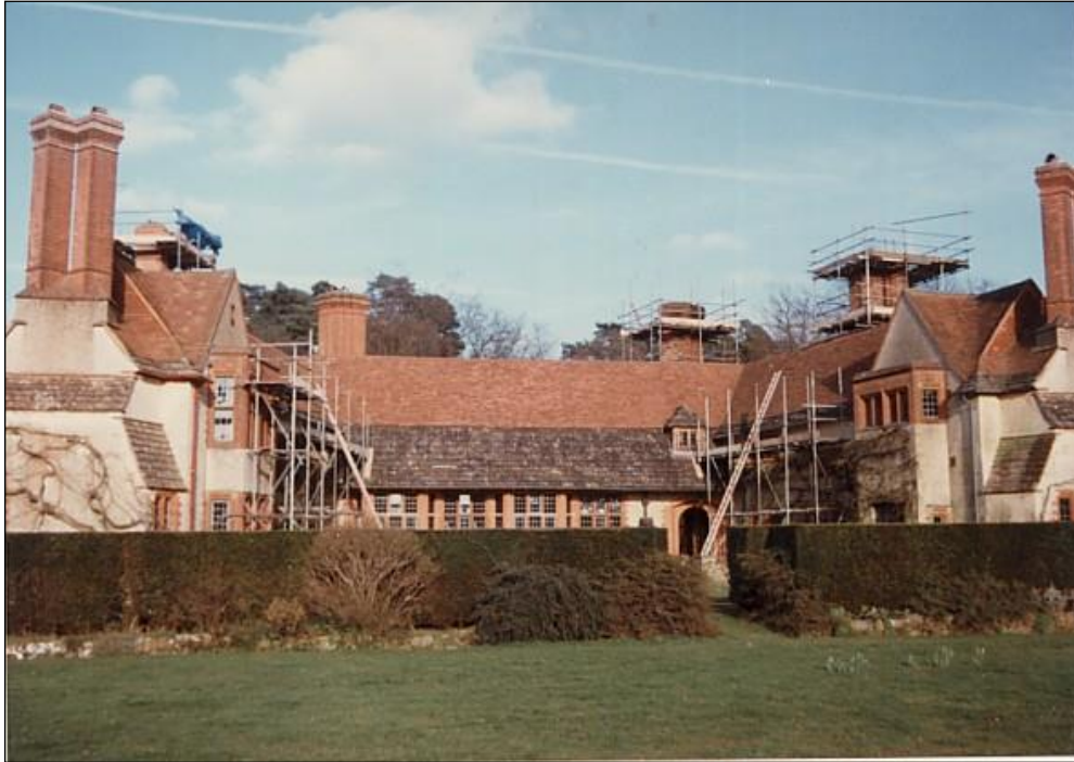
Scaffolding in place for repair to the chimneys and guttering.
