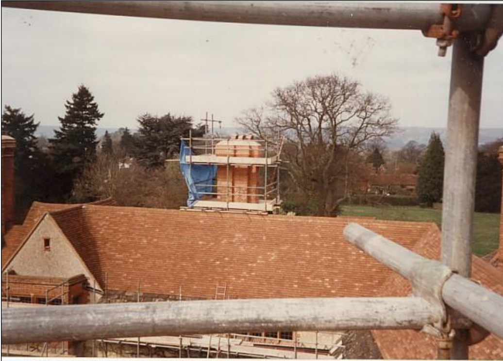
The middle chimney on the north side was rebuilt.
