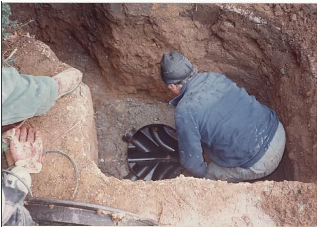
The new manhole by the back door.
