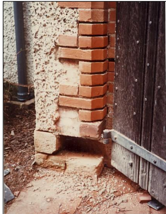
The skittle alley door. The stone plinth was repaired.
