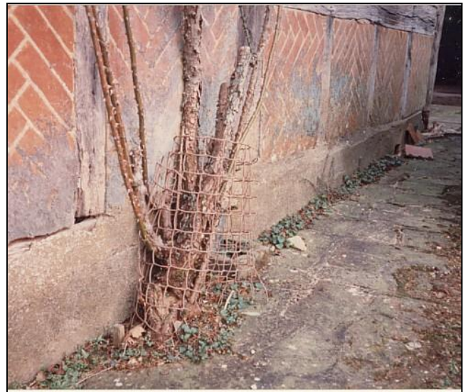
The west wall. Render covered old brick repairs and a defective sole plate.
