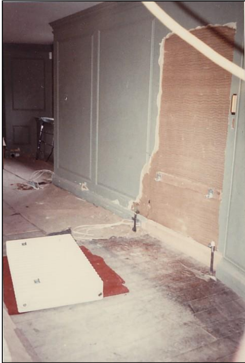
The hatch in the sitting room was blocked up.
