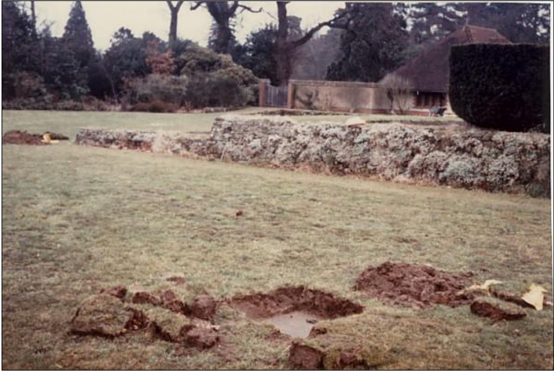
The junction manhole to the main drain by the road.
