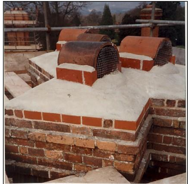
New flaunching and grilles on the south east chimney.
