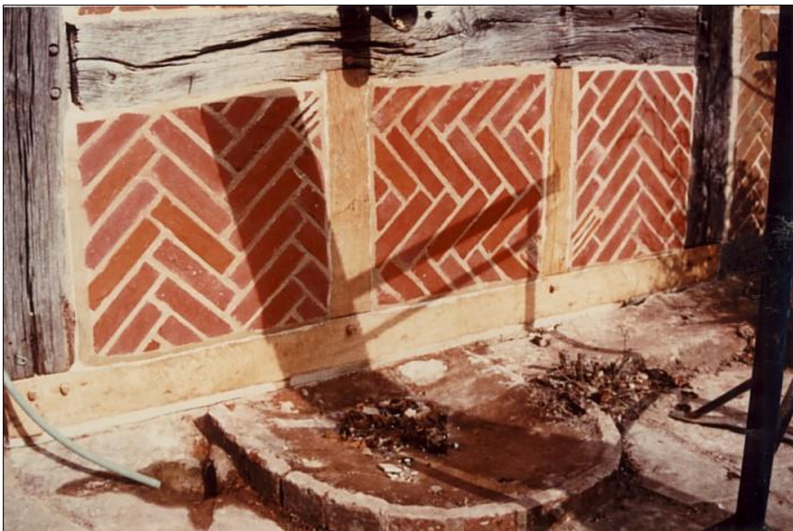
The repairs: a new sole plate, studs and pipe.
