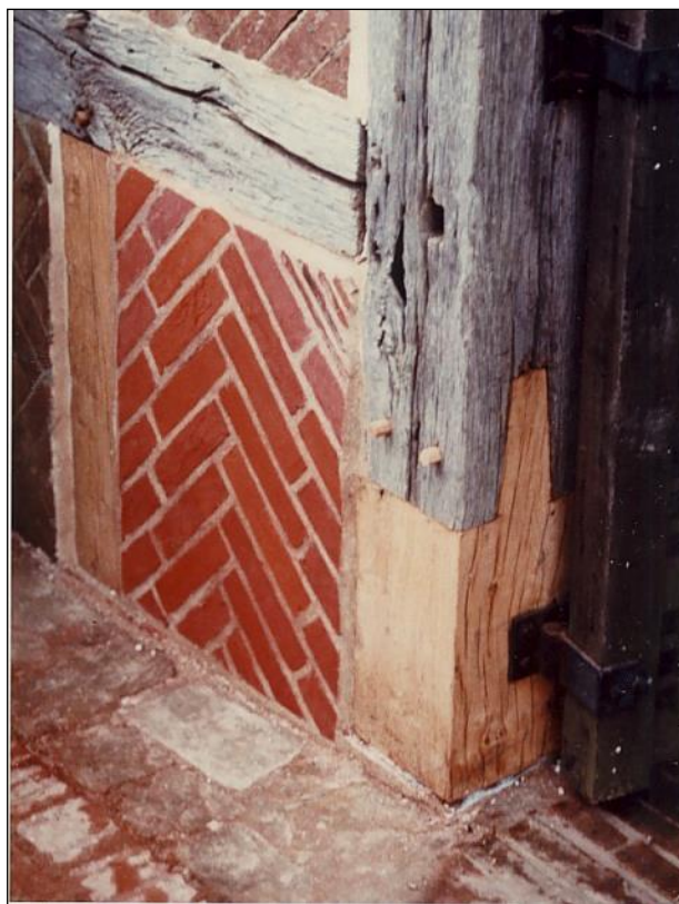
The east post of the north entrance archway before and after repair.
