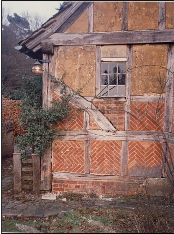
The west wall. Render covered old brick repairs and a defective sole plate.
