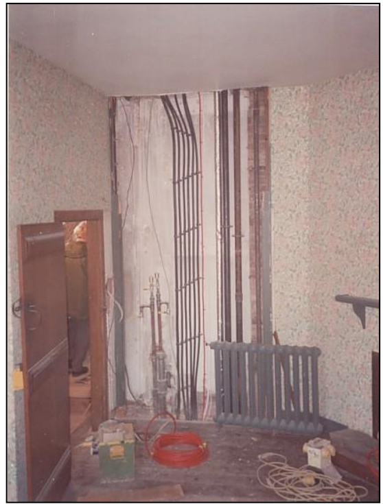
Bedroom no. 4, work in progress.
