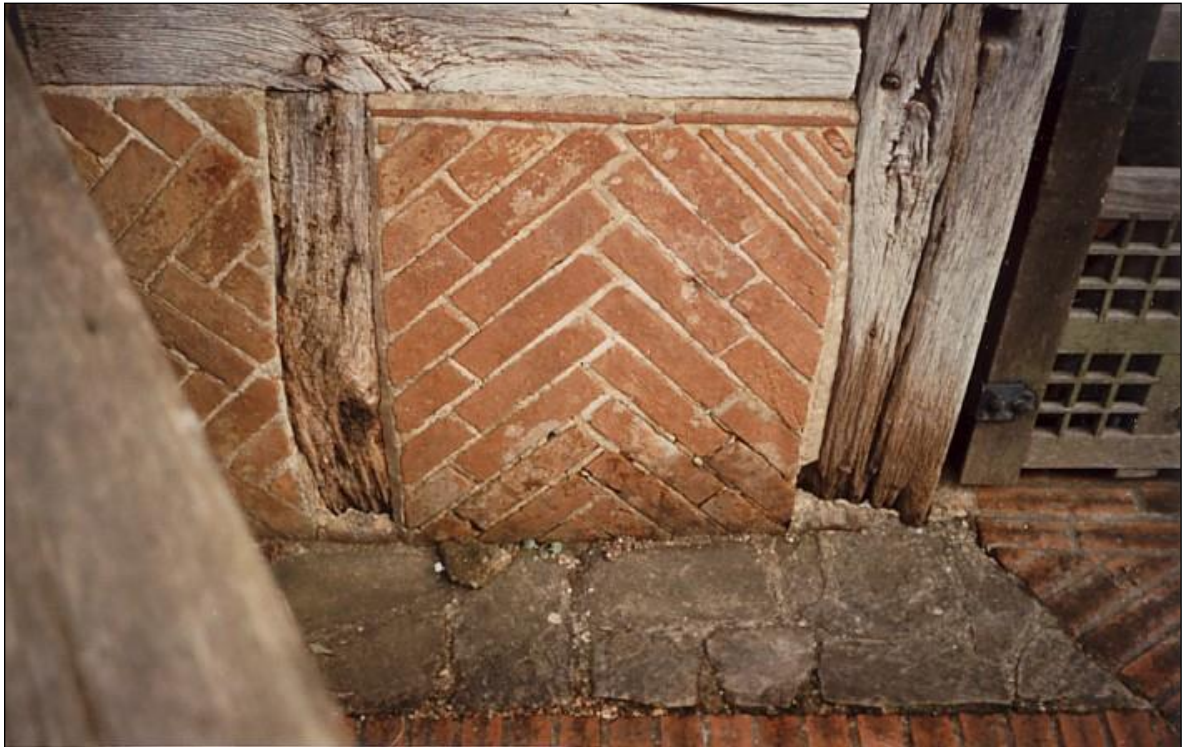
The east post of the north entrance archway before and after repair.
