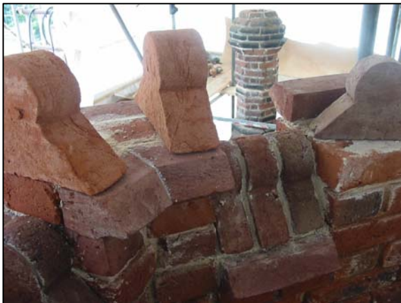
Coping stones waiting to be set.
