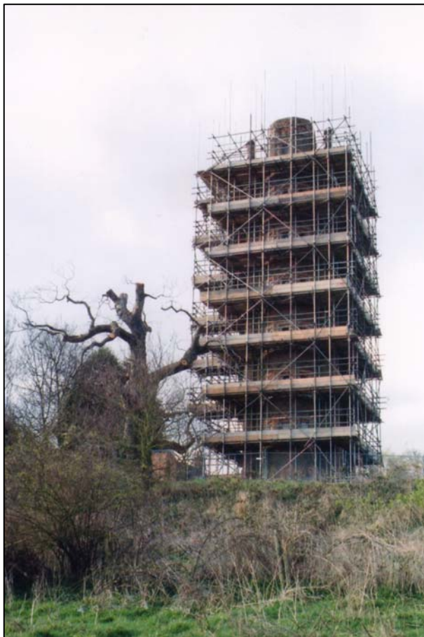
Early spring 2003: scaffolding up...
