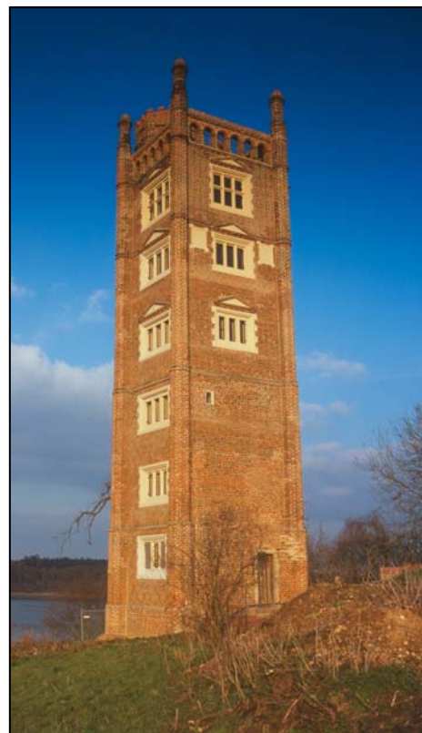
(The tower after restoration to compare)
