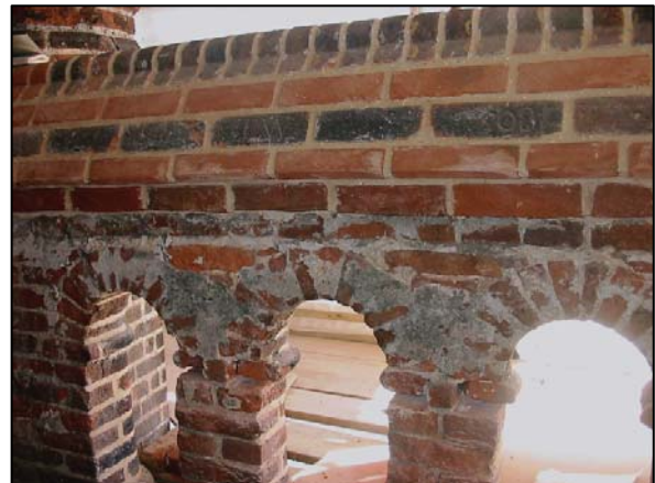
The finished job, old bricks carefully reused with clumsy former repairs also apparent
