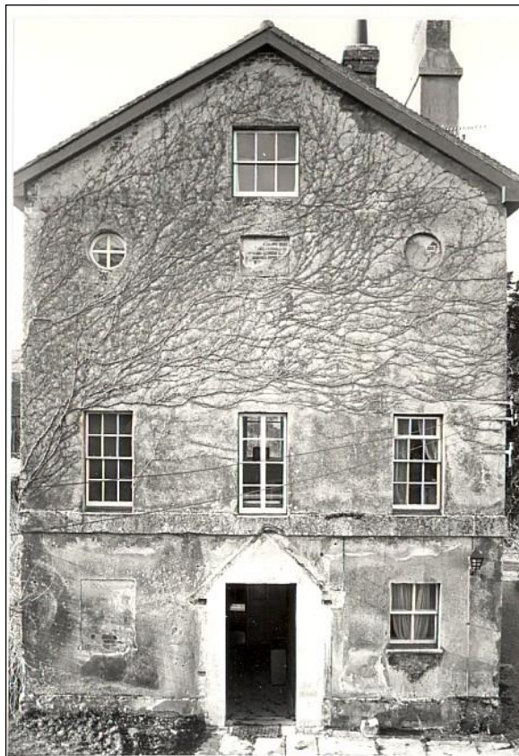
The mark left by the passageway linking the house and stable built in the 19th century is clearly visible.
