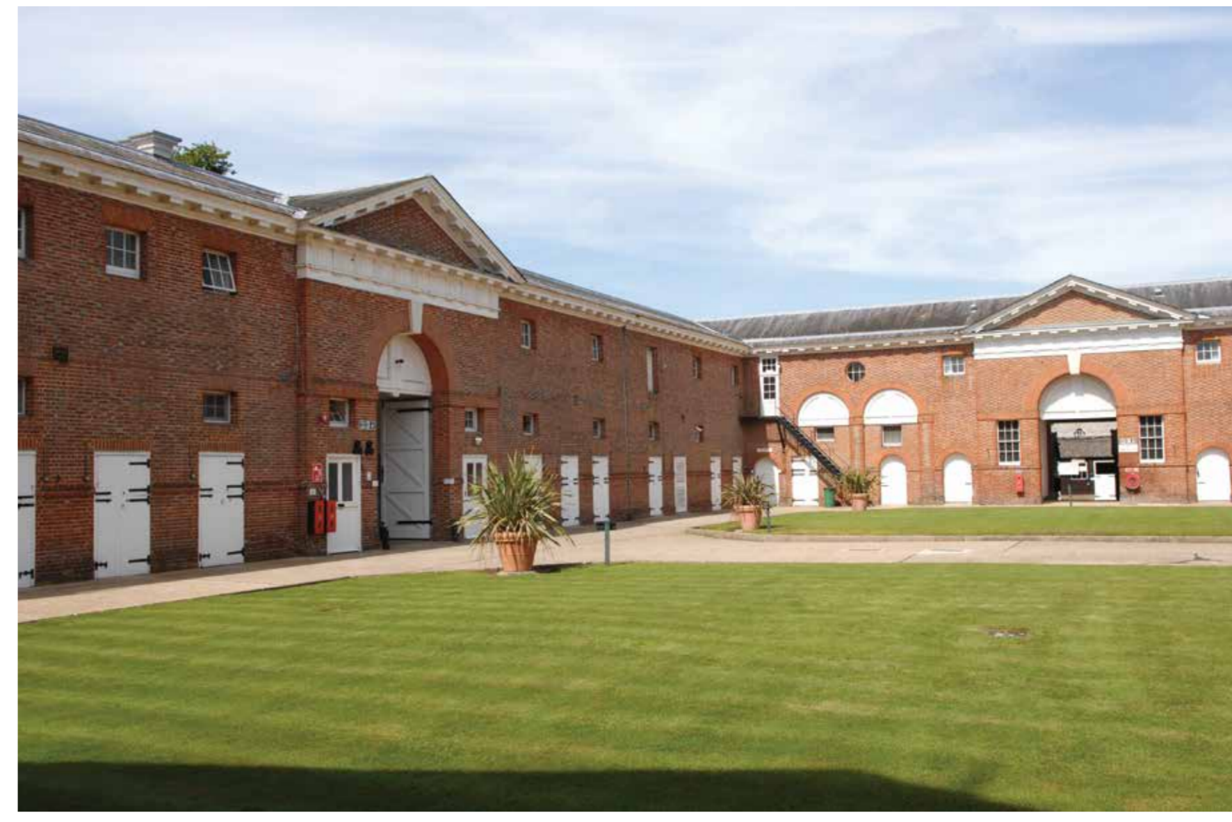
The brick courtyard of the Stables
