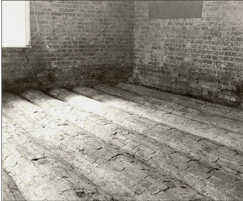
Brick under paving on the ground floor.
