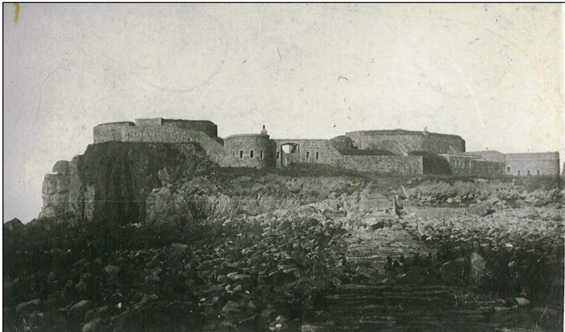
The old causeway, before it was covered with concrete
