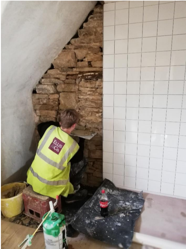
Careful repointing in lime mortar.
