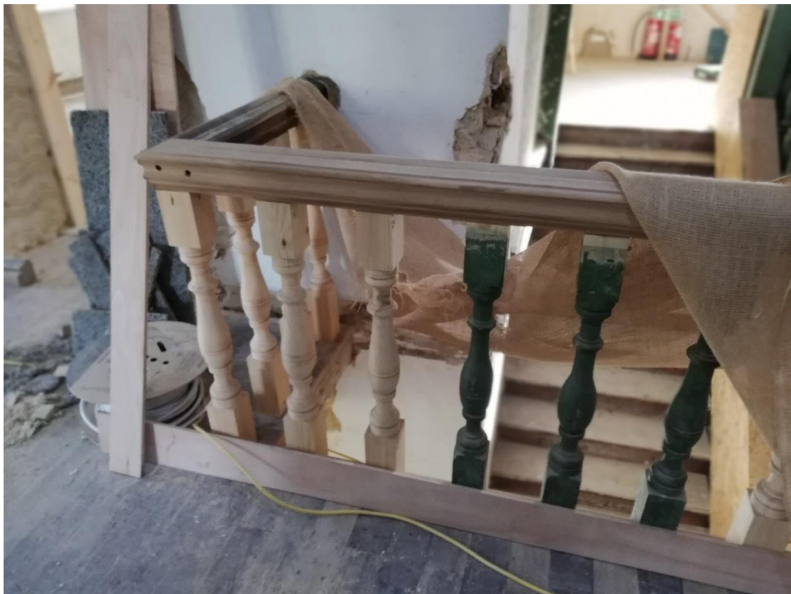
Extension of the landing balustrade, the new posts turned by Landmark's joiner.
