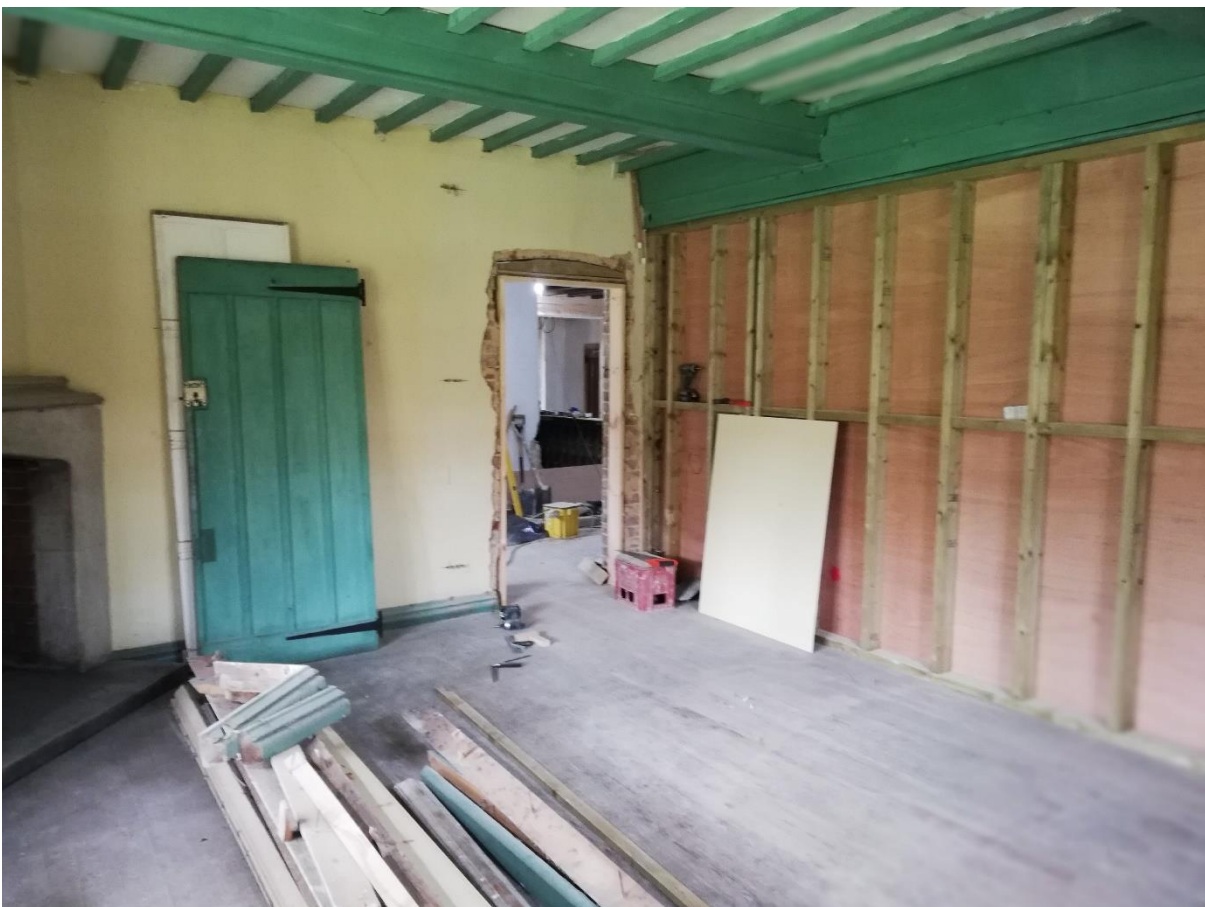
New first floor partition reinstated on its former line.
