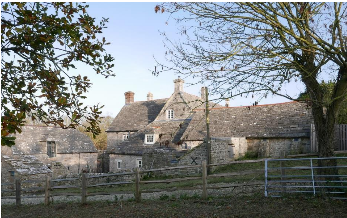
Dunshay from the west is a jumble of accreted outbuildings around a little courtyard. Christopher Dolling's late 16 th -century range is the one with the dormer window, now overshadowed by the later wings. On its right today is the large cider barn, and on its left is the detached Dairy.
