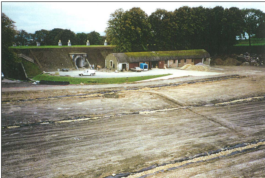
Drainage was installed under the parade ground in 1994
