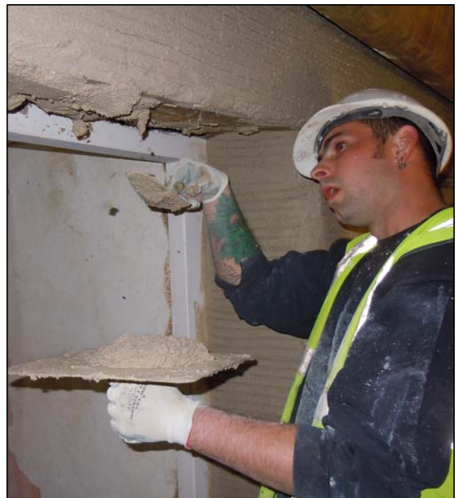
Plastering the first floor walls with lime plaster. Clockwise from top left: the wall is dampened to ensure a good take; the base coat of plaster is applied; next it is 'scratched' to ensure adhesion of the final top coat; some areas are easier to plaster than others!
