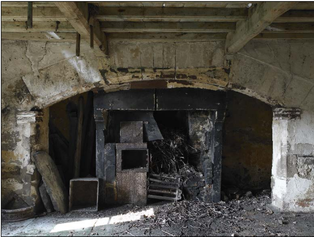
The inglenook fireplace before restoration.
