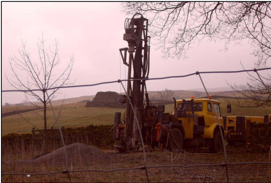
Drilling the borehole for Cowside's water supply.
