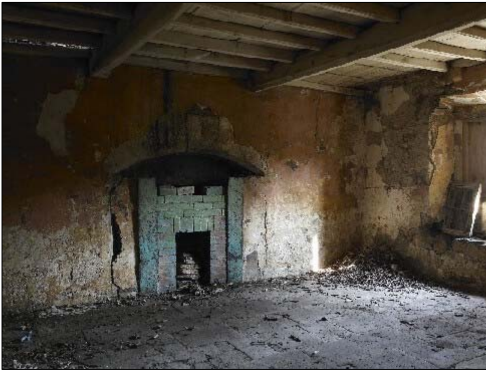
The parlour before restoration, its hearth infilled with mid 20 th -century brickwork. At this stage, the wall paintings lay undiscovered in the corner.
