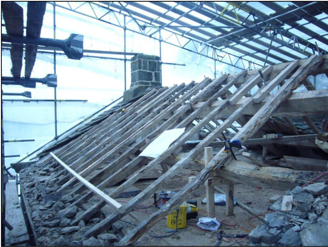
Autumn 2009. Wrapped against the elements, the roof tiles have been carefully removed, revealing remarkably slender rafters for the weight borne. When the snows came, it was a comfort to know that the roof was sound.
