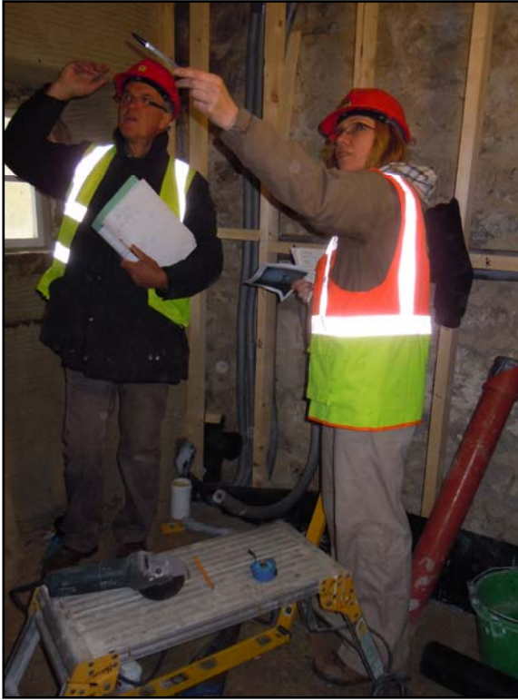
Architect Linda Locket and Landmark's furnishings manager John Evetts reviewing the arrangements in the bathroom over the washhouse.
