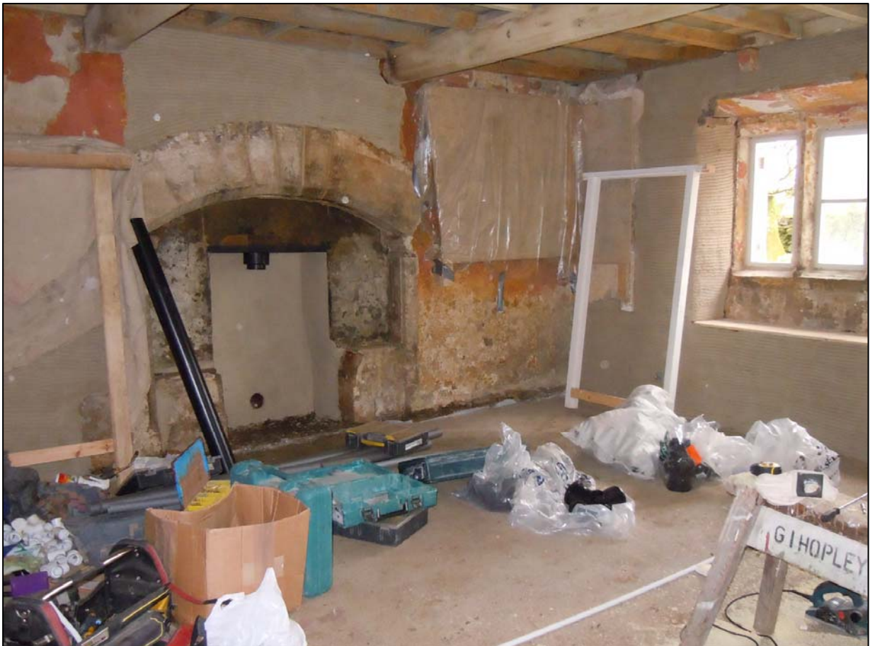
The parlour in April 2011, now re-glazed and with the as yet unrevealed wall paintings still masked for protection.
