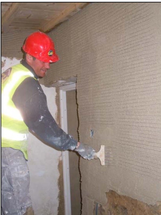
Plastering the first floor walls with lime plaster. Clockwise from top left: the wall is dampened to ensure a good take; the base coat of plaster is applied; next it is 'scratched' to ensure adhesion of the final top coat; some areas are easier to plaster than others!
