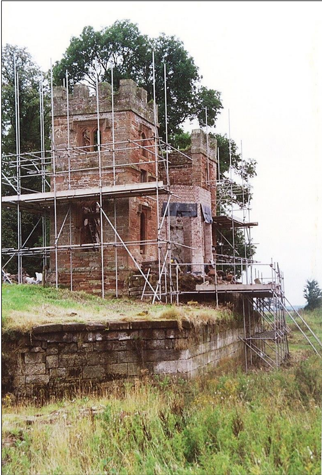
During restoration in 1994 – soil has built up again to hide the coops.
