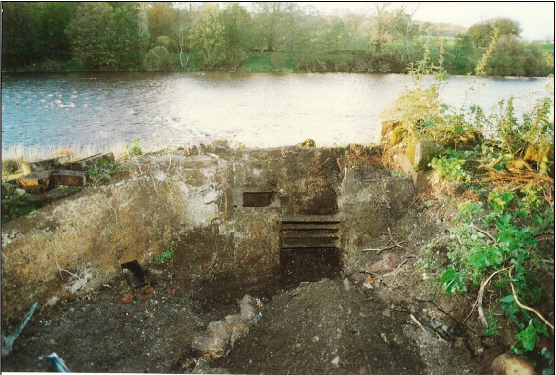
Excavating the bay.
