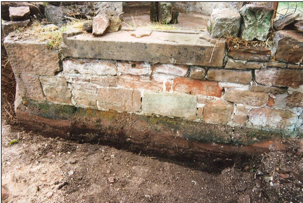
A surviving window sill
