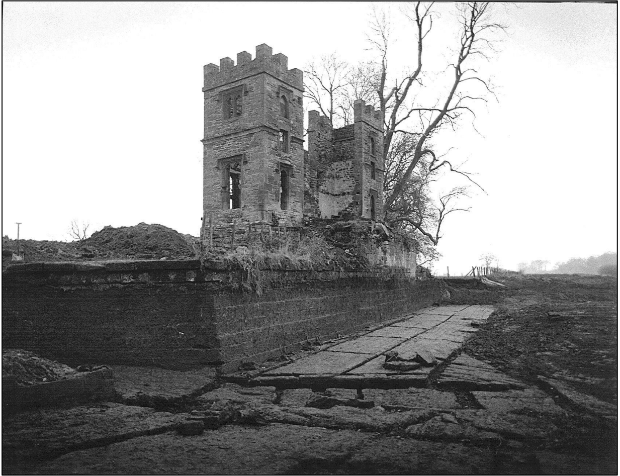
The excavated platforms for the coops, since covered over.
