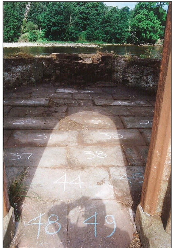
The raised ground level in front of the bay (left). The paving stones in the main room, numbered ready for lifting (right)
