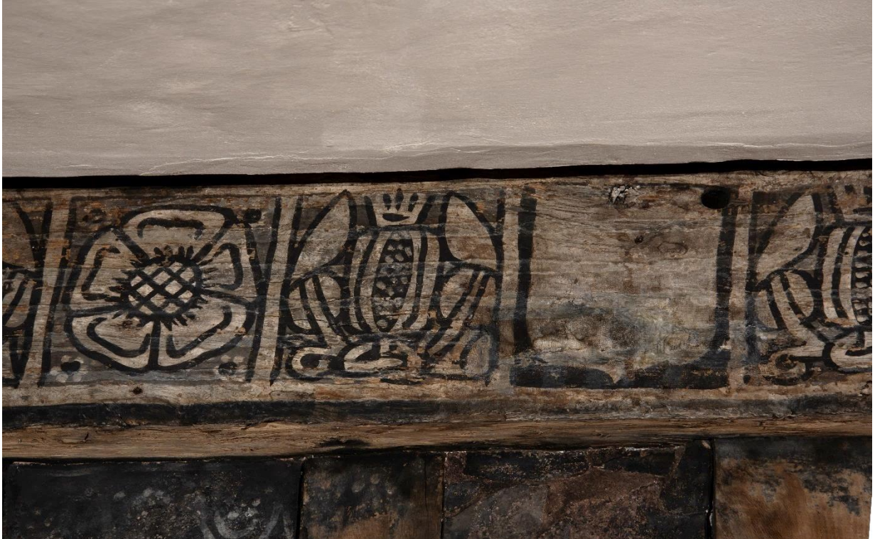
Detail of the grisaille frieze that runs round the wall plate at Calverley, of Tudor roses and pomegranates and blank shields. It was perhaps added in the primary phase of the Parlour Block, before the main painted scheme on the walls.
