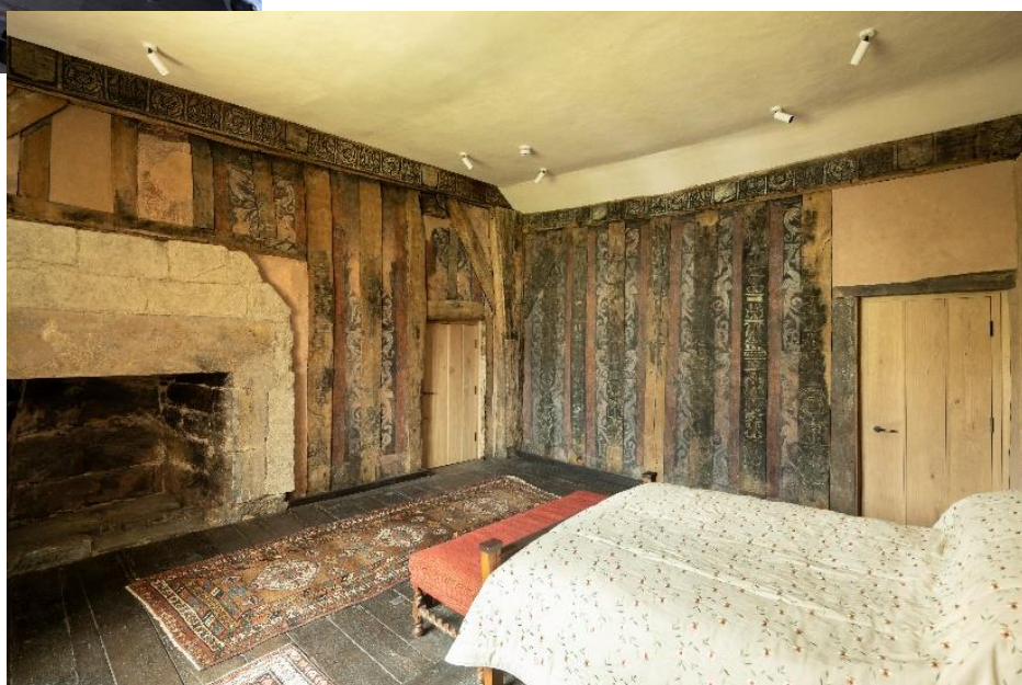
The Painted Chamber in 2017, with the small 20 th -century fireplace, and the same view today.
