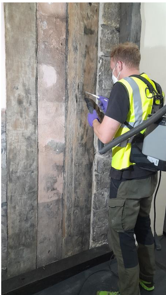
Fig.17 Thick dust on the wooden stud.
