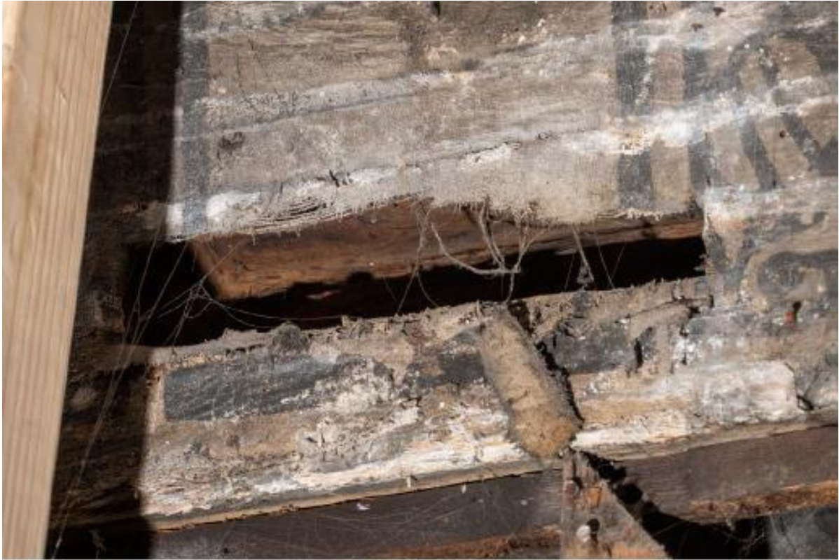
Remnants of a canvas patch used to disguise a mortice hole in the wall plate, tacked in place by the Calverley artist.
