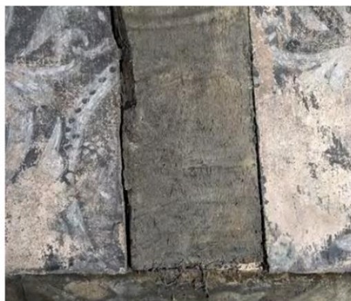
Fig.17 Thick dust on the wooden stud.
