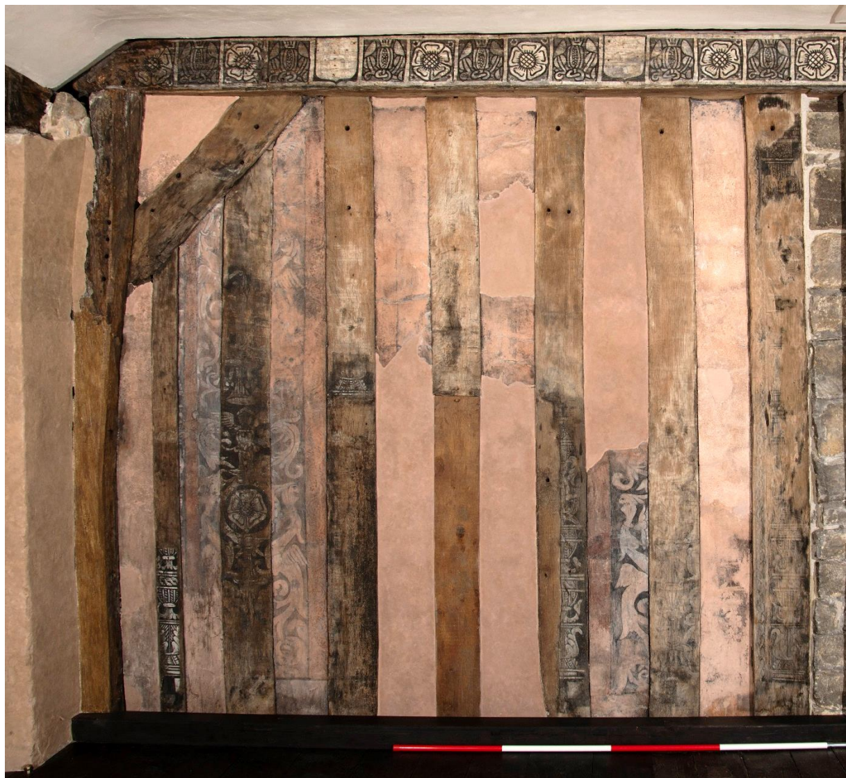
The southeast wall (detail). To note:
