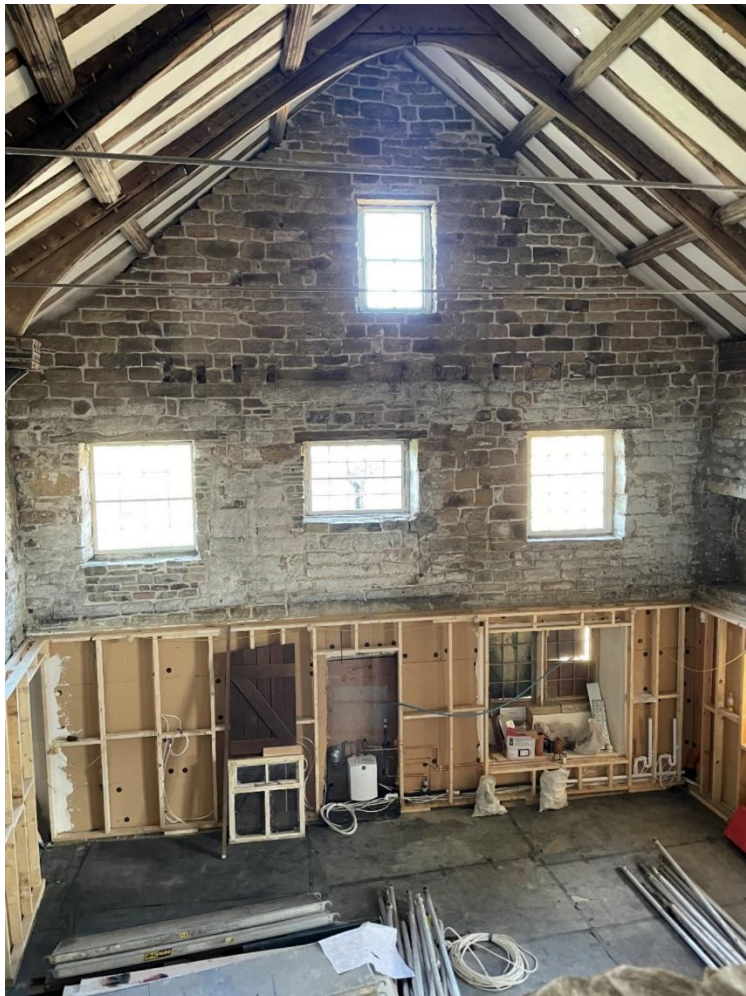
The framework in place for the panelling. The finished panelling provides additional insulation as well as holding pipework for the kitchen and electrical ducting, and being aesthetically pleasing by drawing the space together.
