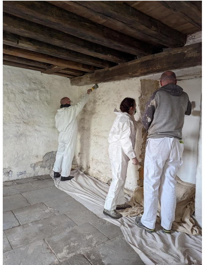
Volunteers learnt about limewash and then used it to redecorate the chapel walls.
