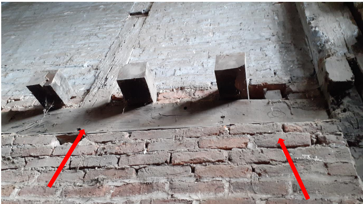
Examples carpenter's scribed setting out marks for the 1320's hall block (now called the Solar Block).
