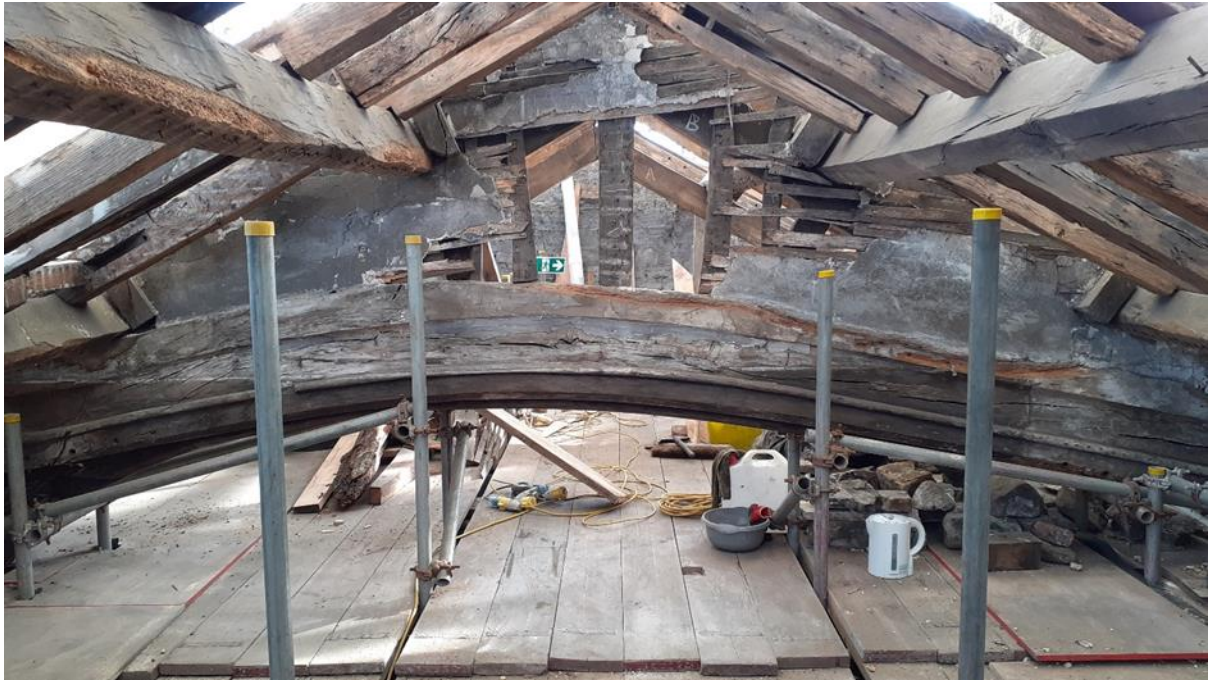
Remnants of lath and plaster above a roof truss in the Solar Block, dating from the 19 th century when three storeys were created in the block. The fabric has been incorporated into the repaired apex.
