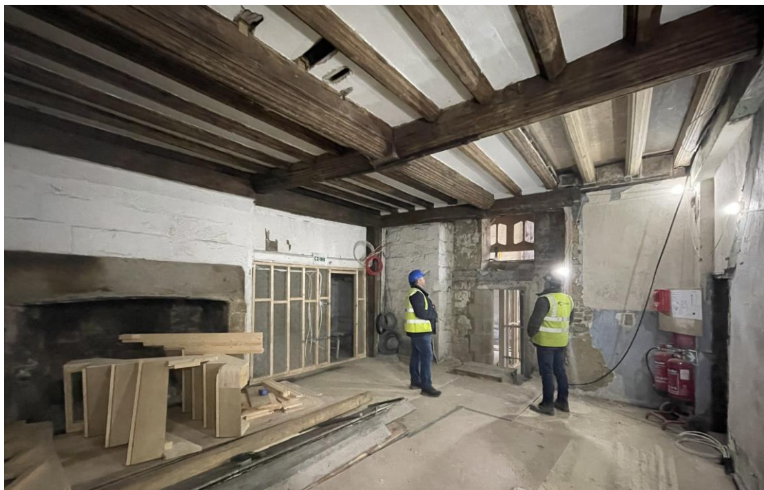
Left: the cottage sitting room (now a bedroom) propped as a precautionary measure. Right: the cottage stairs before removal. By now, the wall paintings had been discovered in the room above and can be glimpsed beneath protective Perspex on the left. Below: the room midway through works. The former breach in the ceiling for the staircase has been made good. The far wall has yet to be finished. The new staircase for the adjacent cottage is under construction.
