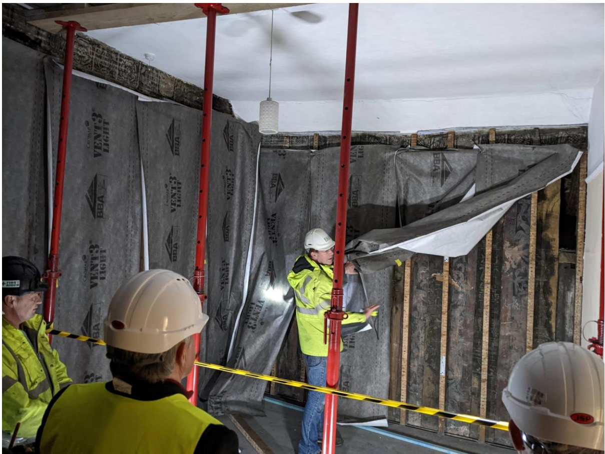
With permission to remove the lath and plaster walls, but the supporting stud work still in place for now, for a couple of years the wall paintings were carefully protected, later with Perspex sheets, revealed only occasionally.
