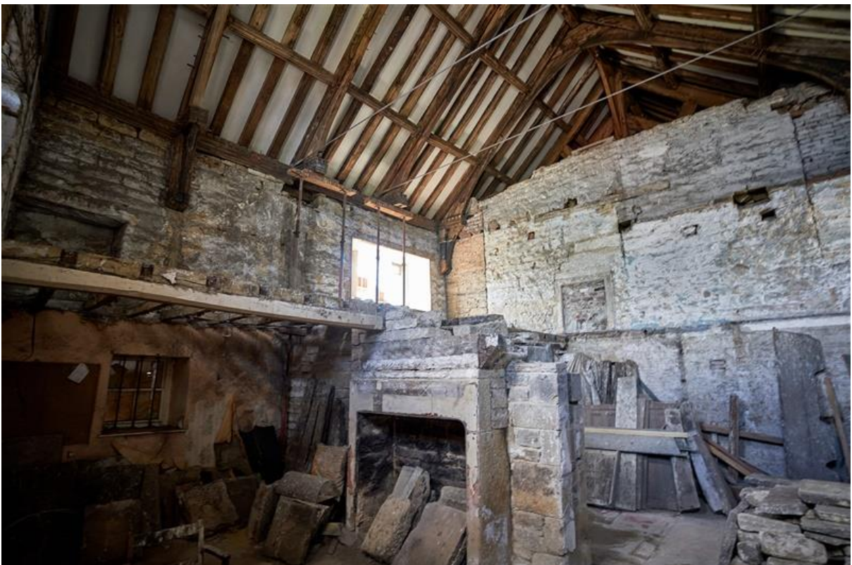
The Great Hall in 2020. The remains of cottage chimney breasts have yet to be cleared. While they remained in situ, it was impossible to find a viable alternative use for the Great Hall. Heaps of carefully salvaged stone and other materials lie on the original flagstone floor.
