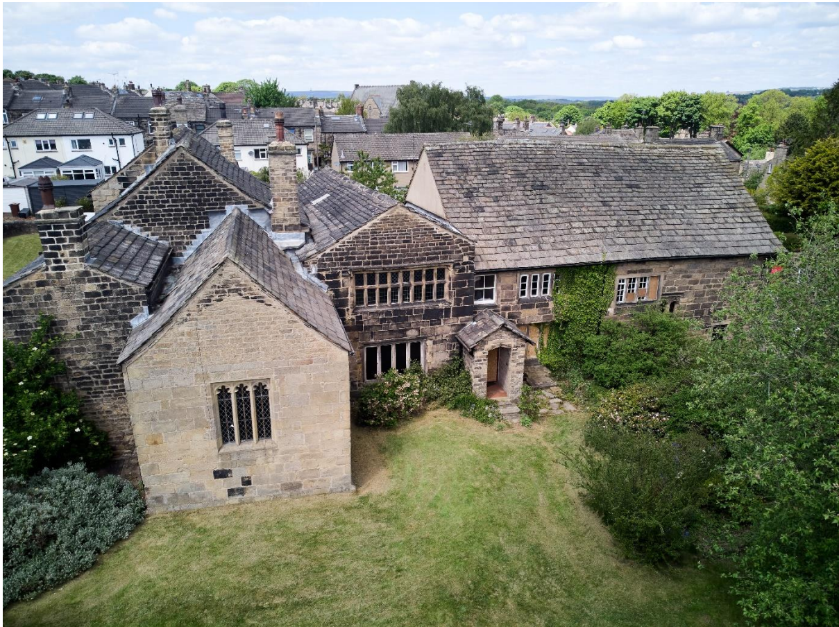
The exterior of Calverley Old Hall in 2020. Much work has been done since to conserve and repair the entire shell, but the intention was that its external appearance should change as little as possible. The little front porch, a late addition, has since been removed.
