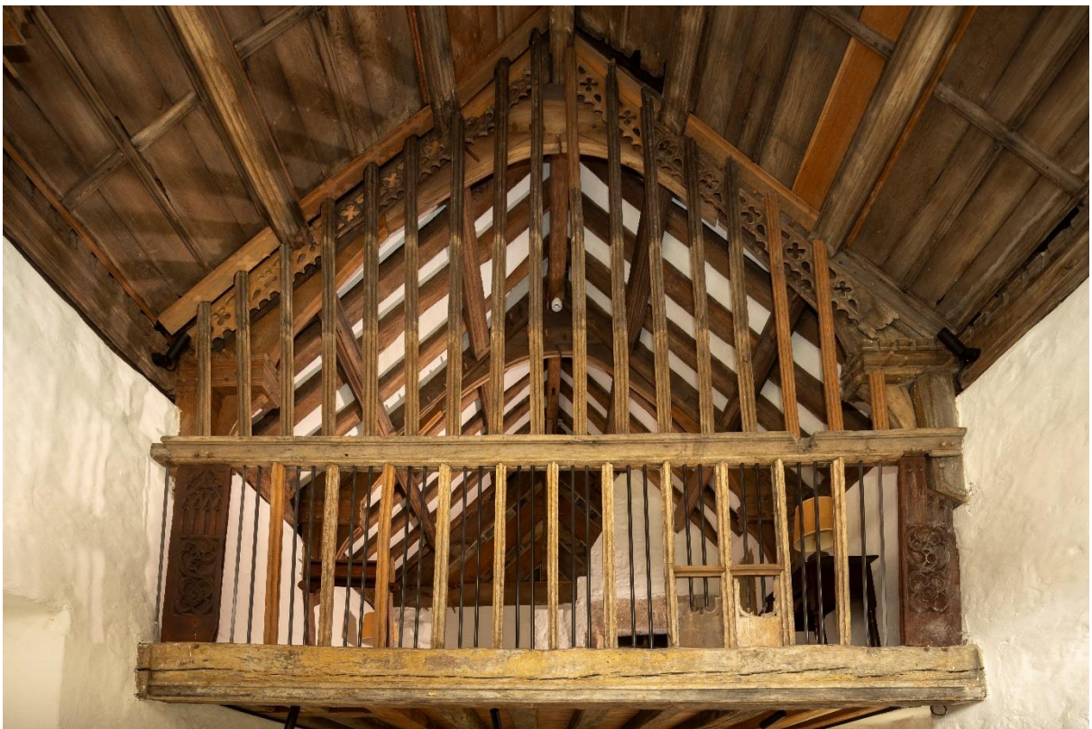
The chapel gallery seen from below, 2024.
