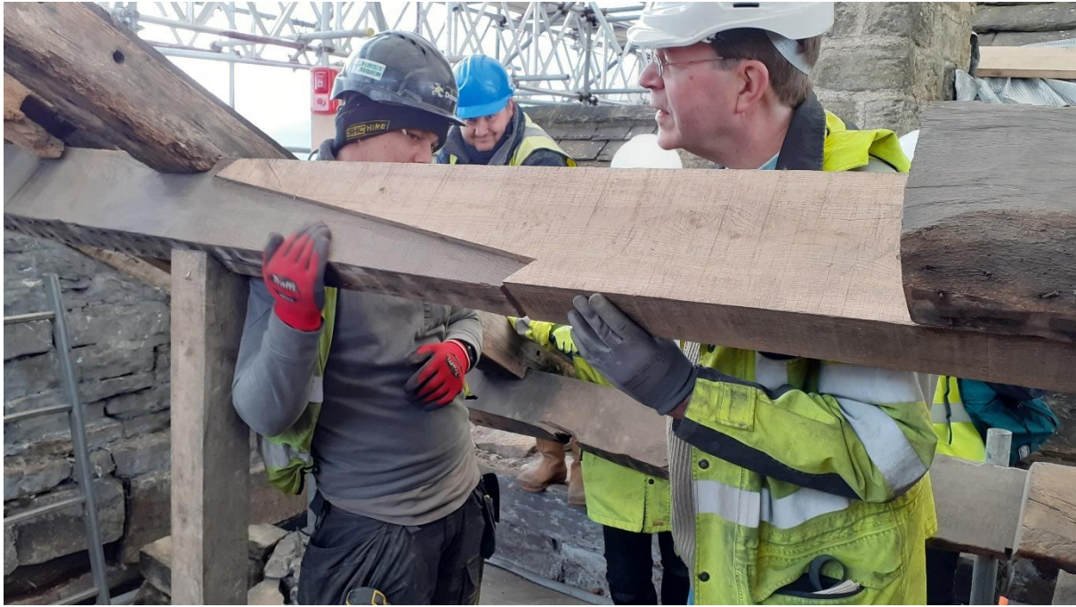
Archaeologist Jonathan Clark inspects a scarf joint repair to a decayed purlin.
