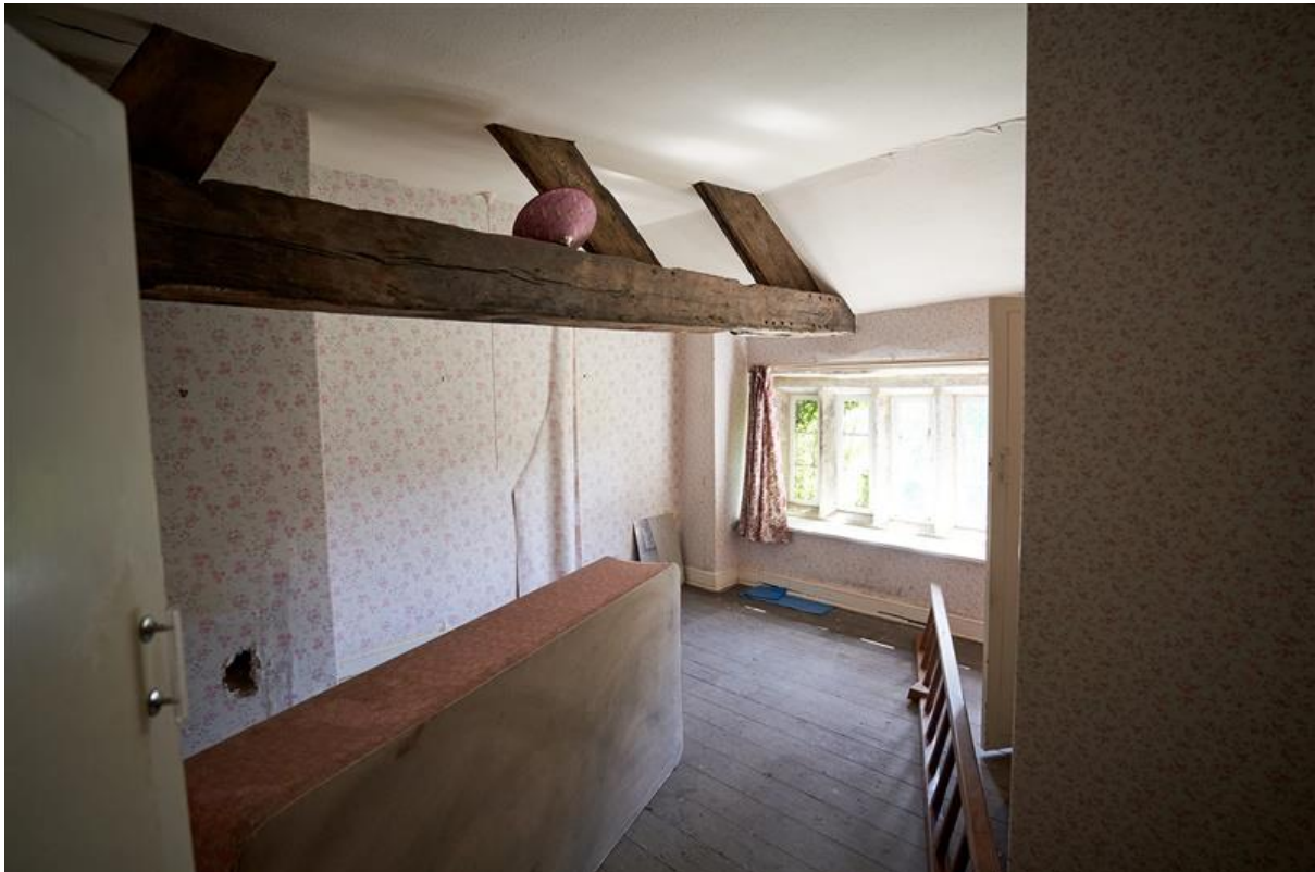
Below: the medieval spere truss protruding through a cottage bedroom.
