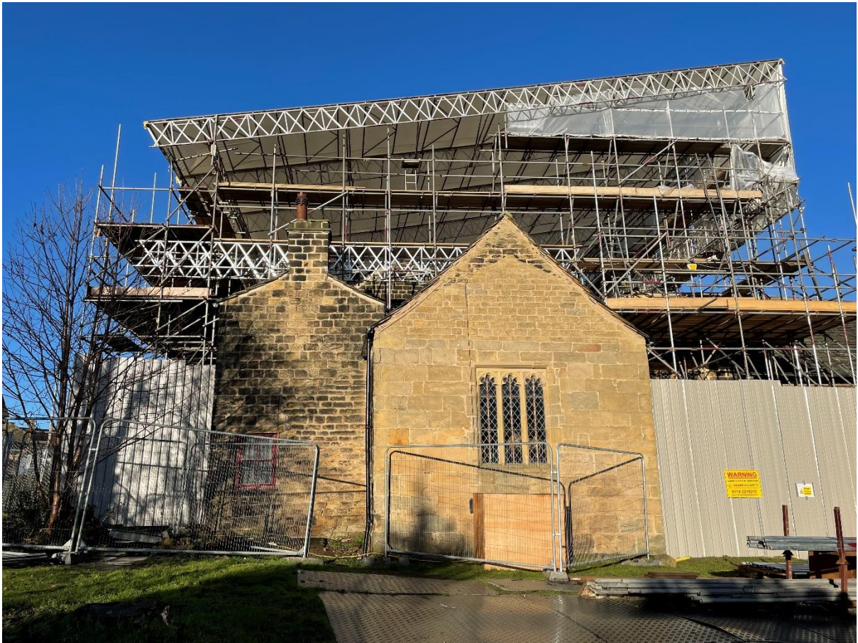
Scaffolding going up for the re-roofing works in January 2022.
