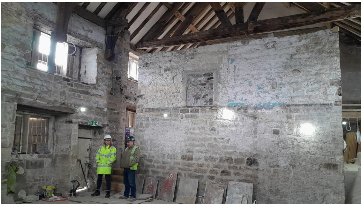
Linda Lockett and Andy Dewhurst contemplate the challenge of installing the panelling in the Great Hall. The image top right shows how far out of true the southeast wall was.
