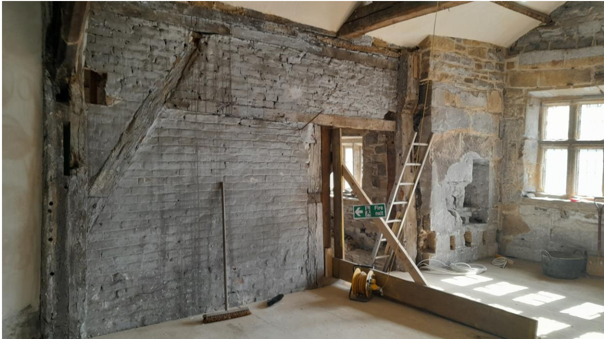
Residual framing from the 1320s hall block, and the original doorway into the first-floor hall, now in use once more, after raising the lintel to take account of modern statures.
