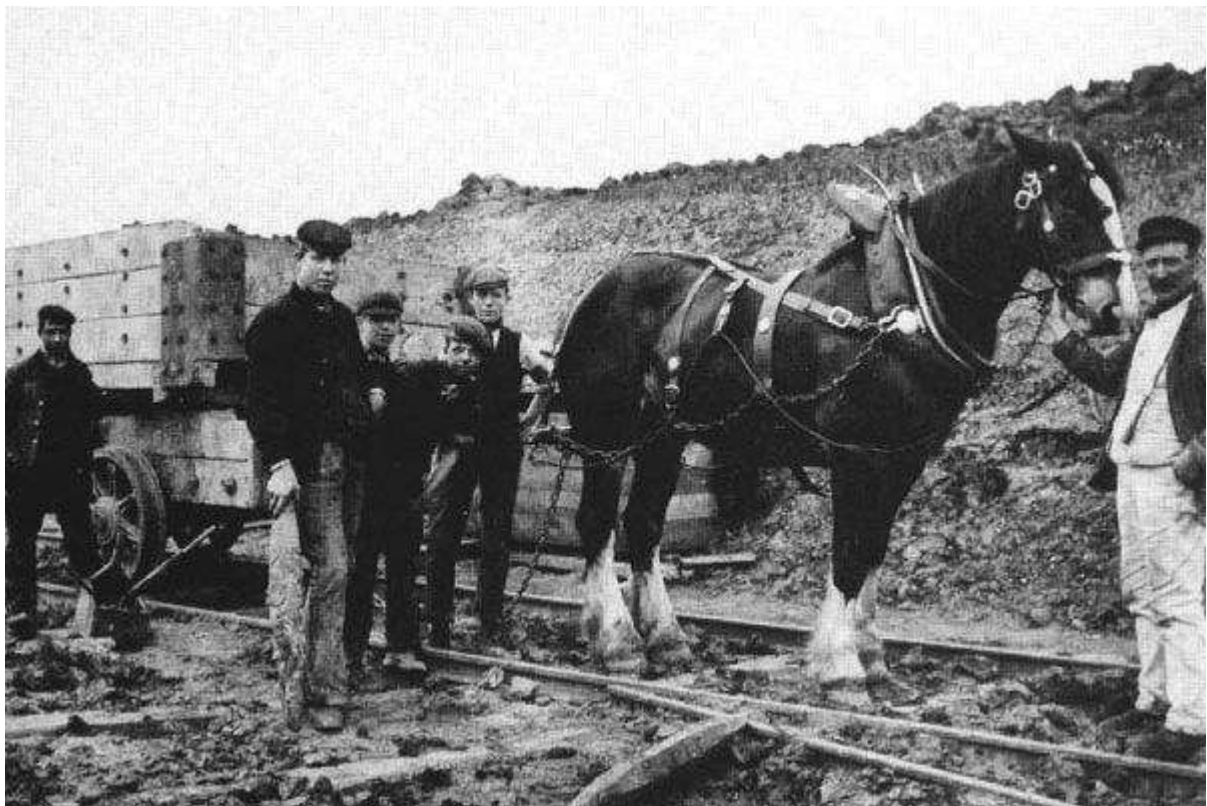
The Embankment was a huge feat of engineering (top, under construction- note Madocks' initials on the wagon). It was executed with the simplest tools and equipment such as this later photo of a horse tram bringing a load of sleepers (location not known).
