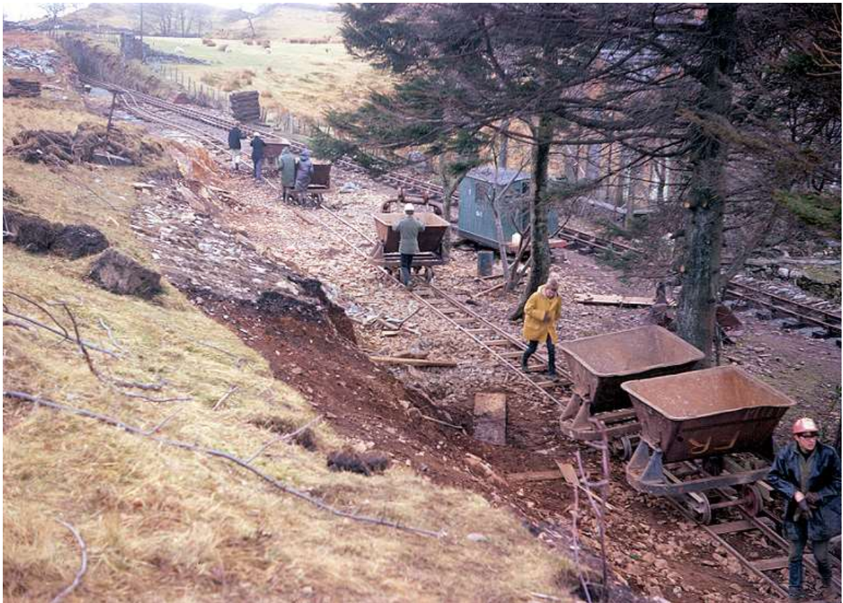
Volunteers working on widening the Dduallt station site in the early 1970s. Note the body of the old brake van being used as a site hut.
