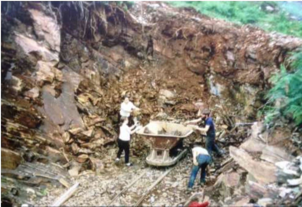
Cutting the line of the new track.
