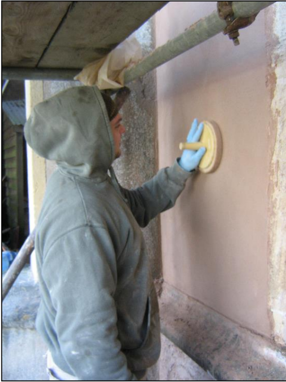
Finishing the render for a smooth finish.
