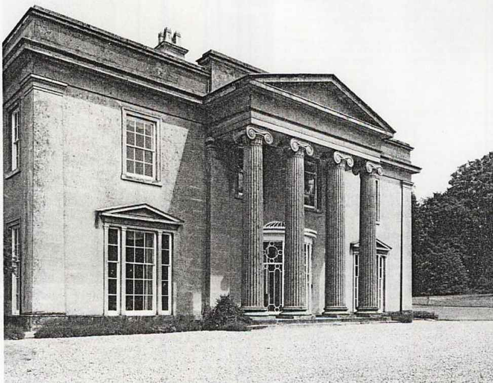
1—THE MAIN FRONT. The portico and circulation areas are the most elaborate parts of the House. The sequence of orders is Ionic, Tuscan and Doric
