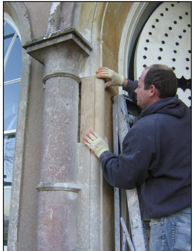
Piecing in a stone repair.
