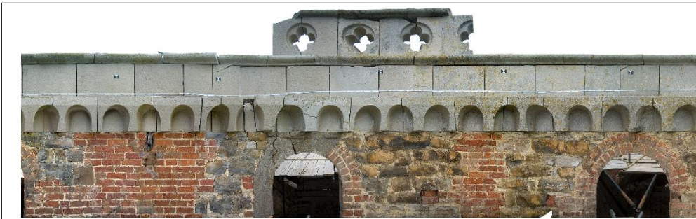
An example of rectified photography and the 3D laser camera used to capture it, using the rectangular 'telltales' for alignment.
