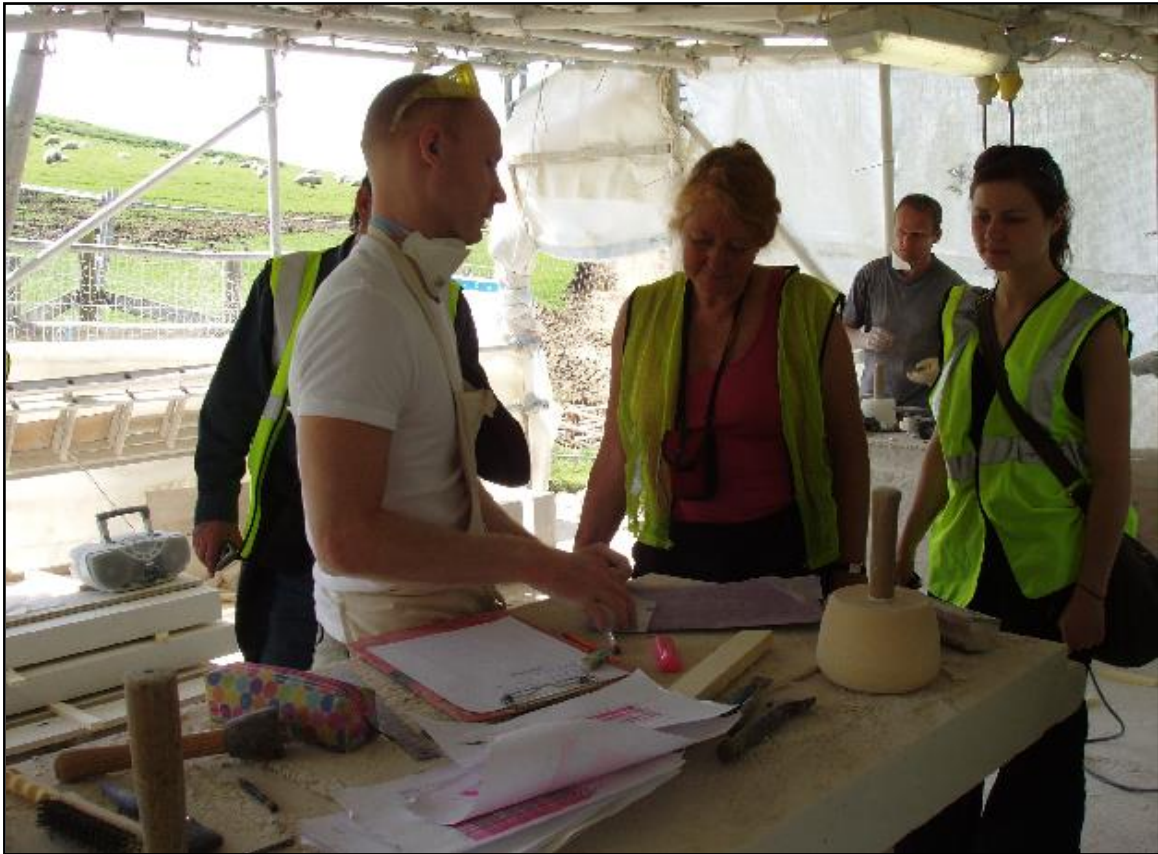
One of Carrek's masons explains the use of templates to a group of visiting students in the bankers' shed.
