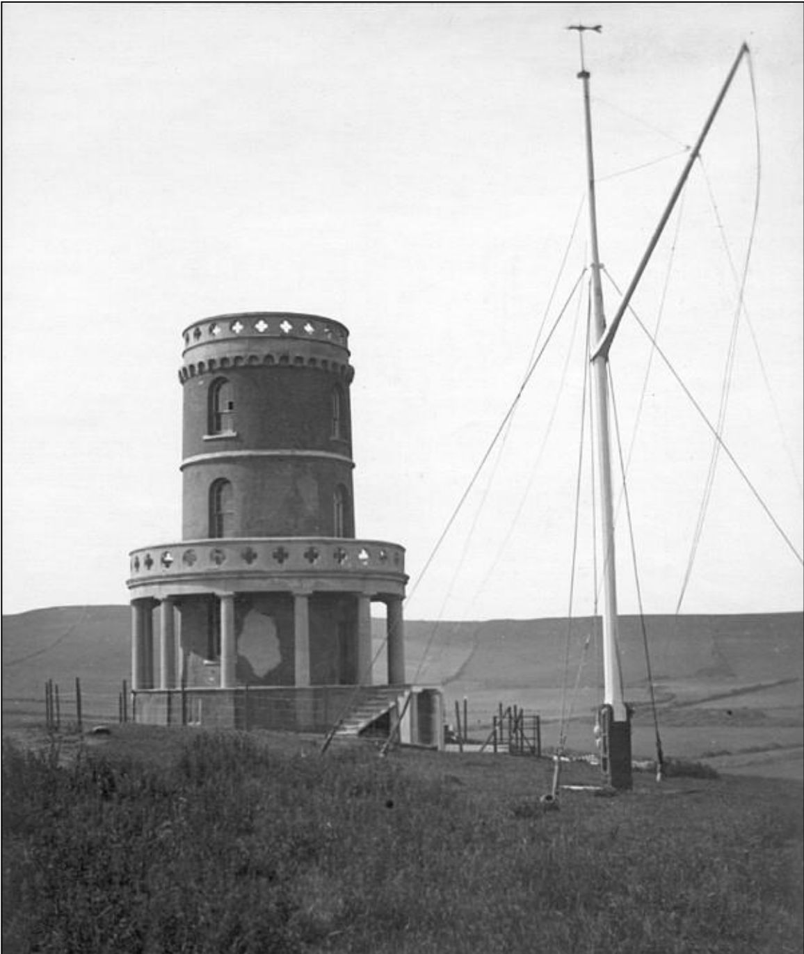
This photo from c1900 shows the tower still in use as a coastguard station. Their flagpole is anchored to the muzzles of four Napoleonic cannon sunk into the ground. After one of these was stolen, another was sold and the remaining two can still be seen at the front of Smedmore House. At this date, the tower is still in generally good condition apart from some missing render and this clear photo was a useful reference during restoration.
