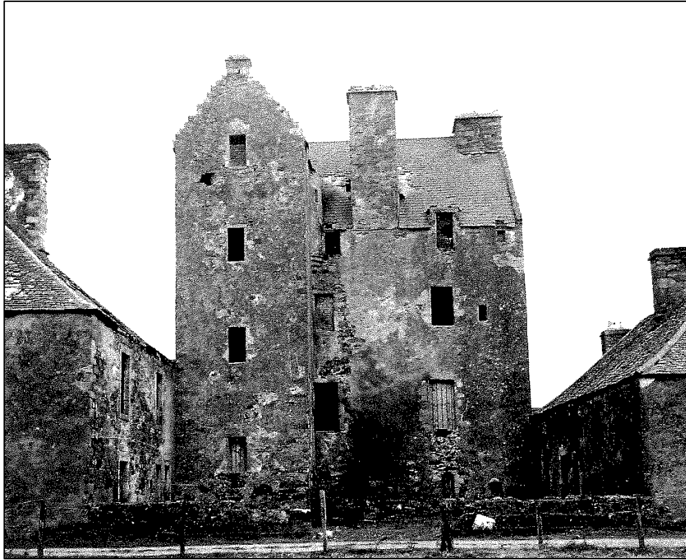
The east side in 1950. It shows the roof in serious disrepair.
