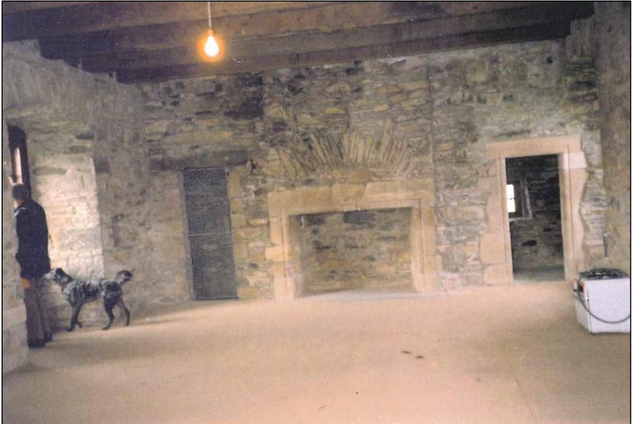
The sitting room in 1989, looking north. The floor has been covered with hardboard.
