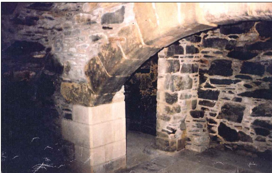
The base of the arch repaired by Historic Scotland in 1976-8.
