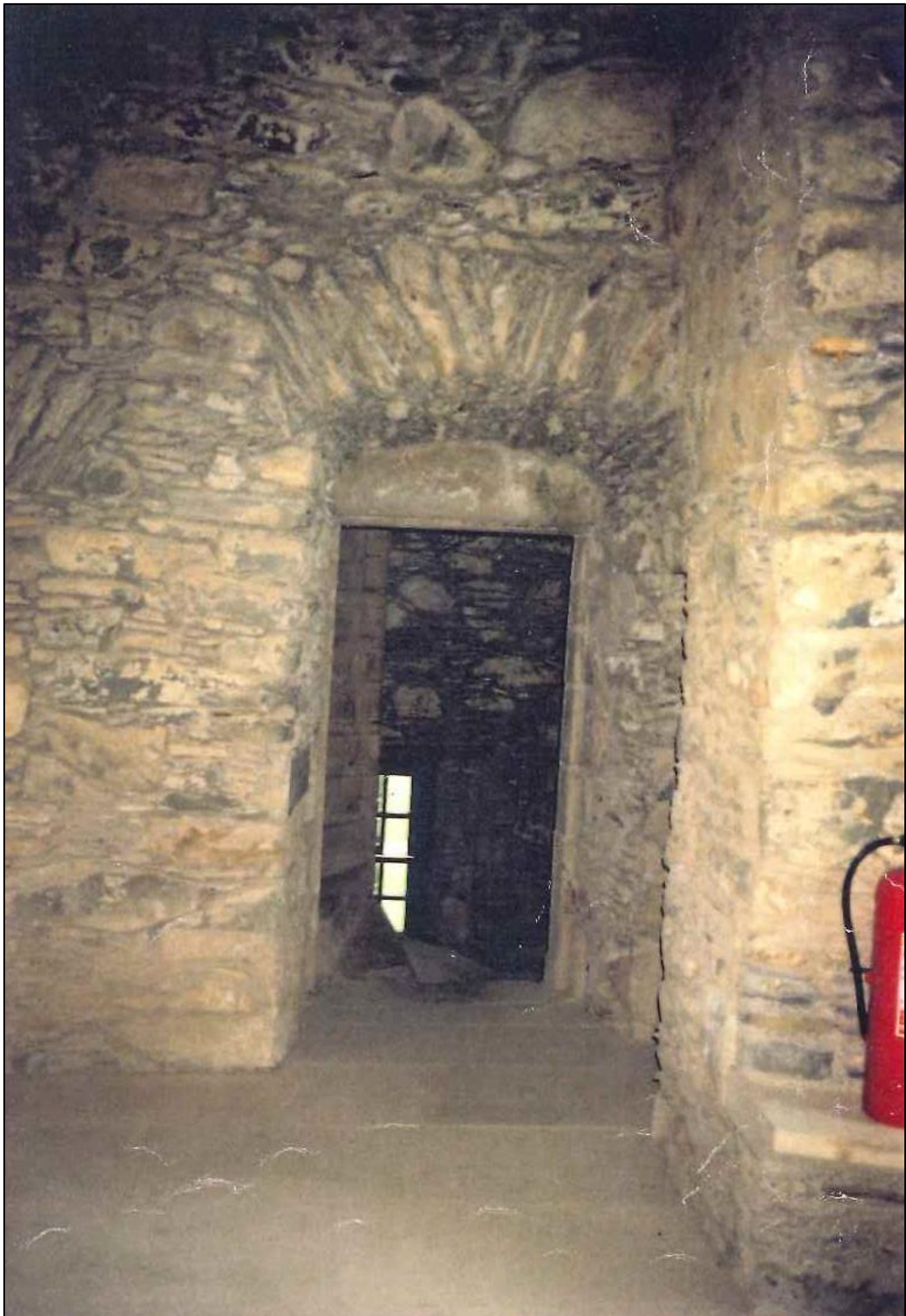
The door from the main stair in 1989.
