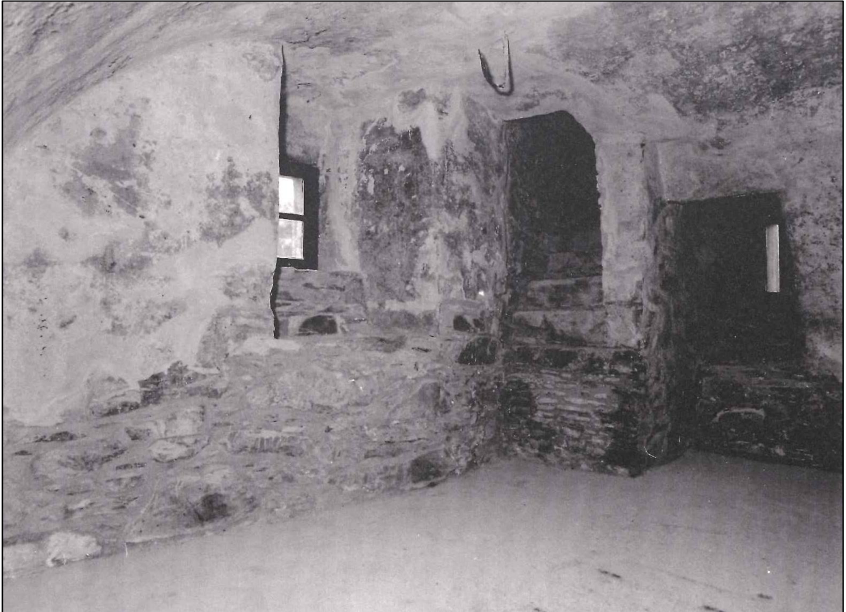
The stair discovered by Historic Scotland leading from the pantry to the servery in the great hall. It stopped two feet above floor level (photo from
