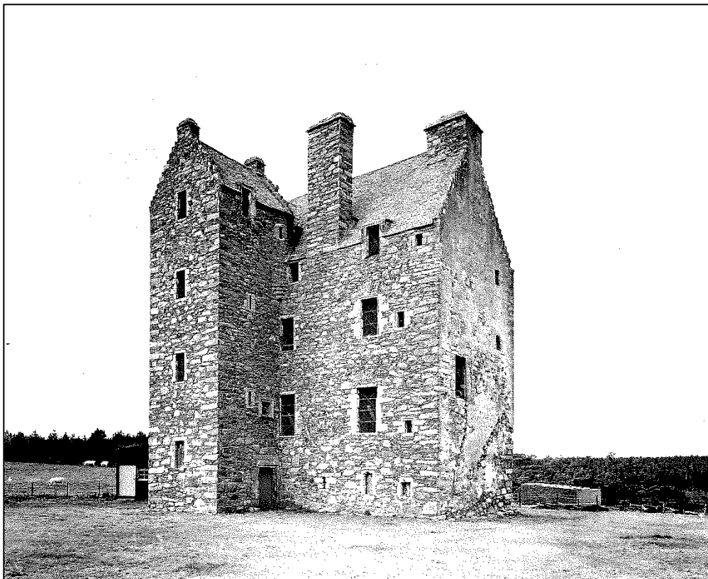
September 1966. The wings had been removed and the castle re-roofed with old slates in 1950-55. In 1966 the harling was stripped off the east side and the walls repointed.
