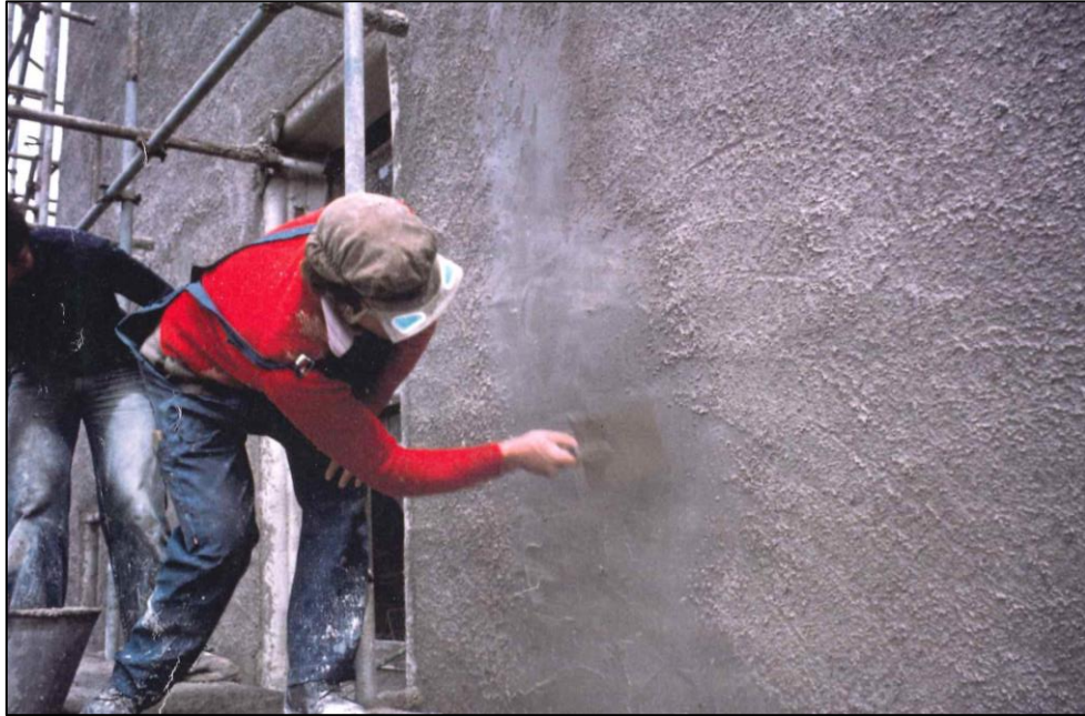
Harling in progress, 1987.
