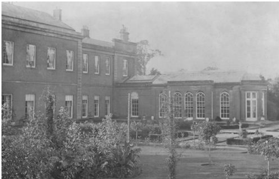
Badger Hall, demolished in 1953, stood NE of St Giles's Church. A smaller house built in 1719 (top) was greatly extended and remodelled for Hawkins Browne by James Wyatt in 1779-83. The large brick conservatory seen in the bottom picture was added in the late 19 th century.
