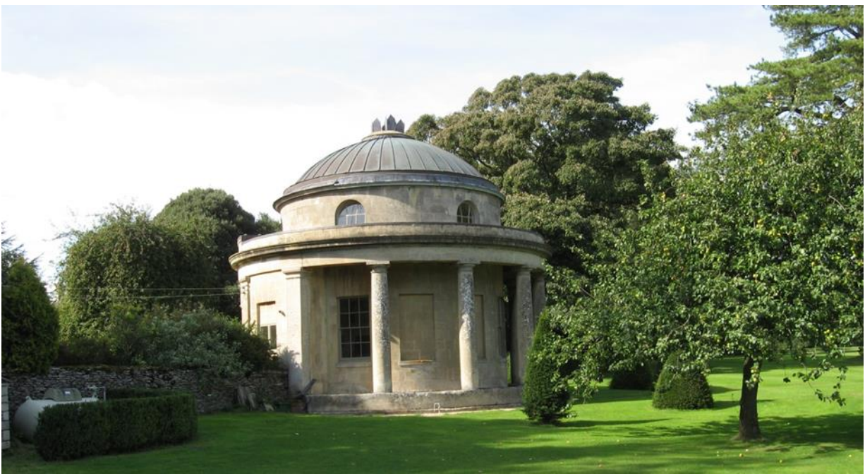
Bath Lodge, Doddington Park, Gloucestershire is another pavilion by Wyatt (who was active there 1796-1813). It shares with The Birdhouse Wyatt's characteristic baseless Doric columns. 'Wyatt's use of the Doric order is one of the keys to understanding his architecture and its easy and assured variation; his classical learning was worn lightly, producing a harmoniously eclectic and sophisticated synthesis.' (JM Robinson 2012, p.280).
