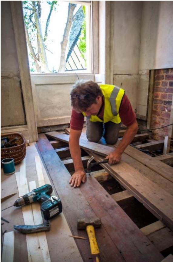
Left: Angus repairs floorboards, retained wherever possible. Right: Jim and Steve working on the reinstated stair finial, created from a bedpost.
