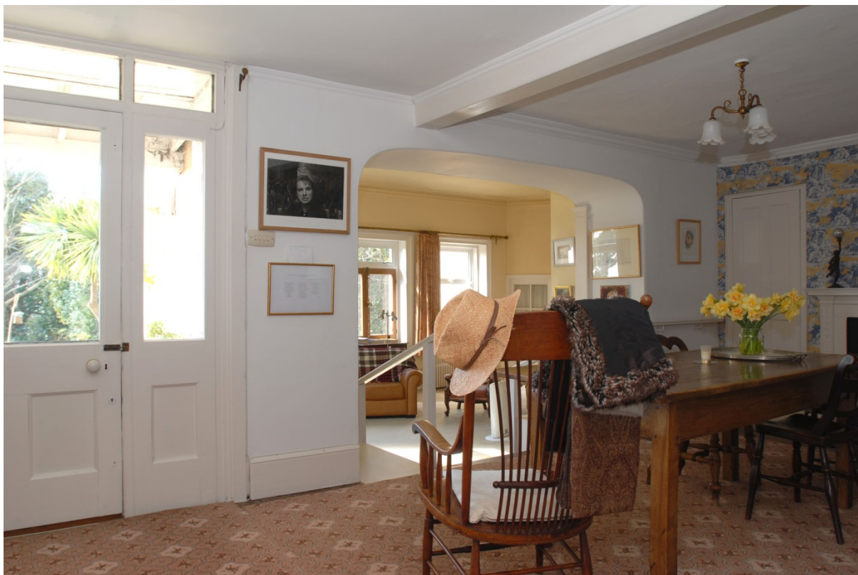
The view through from the rear hallway to the later extension, as knocked through during the 20 th century, with the partition wall beneath the cross beam also removed.
