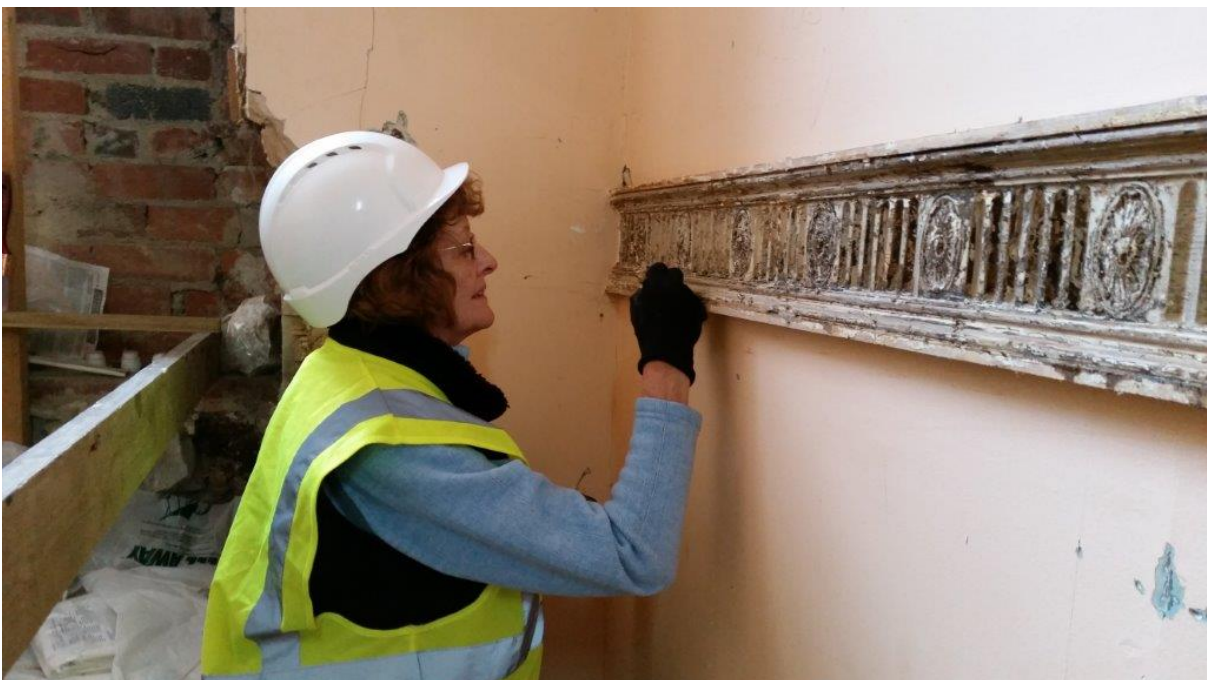
Removing layers of paint from the Coade embellished dado rail on the stairs and from cornices elsewhere was a time consuming and painstaking task, on which we were grateful for volunteer help.
