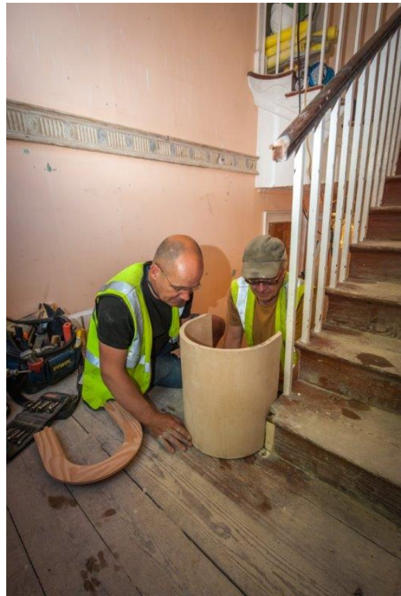
Left: Angus repairs floorboards, retained wherever possible. Right: Jim and Steve working on the reinstated stair finial, created from a bedpost.
