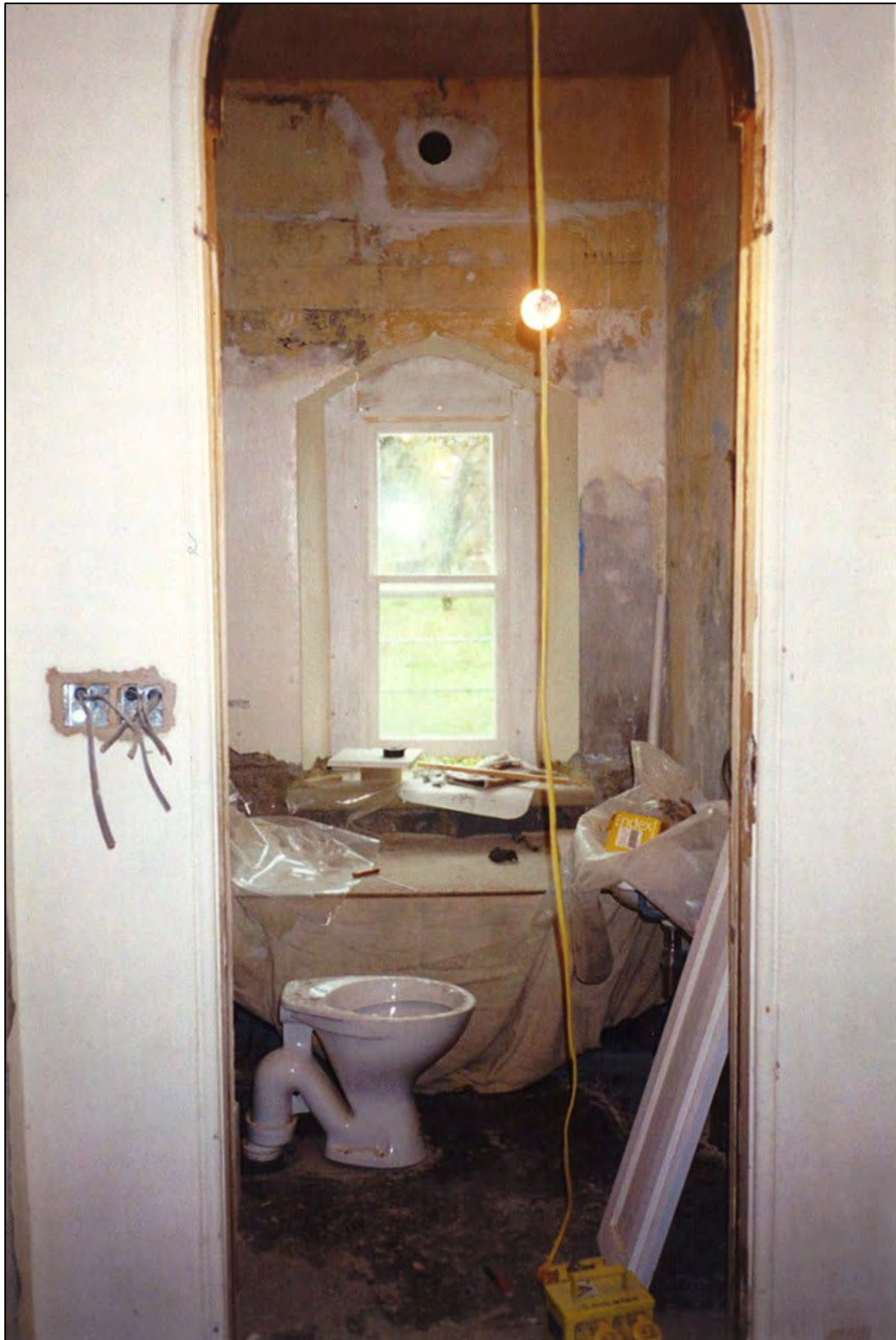
The bathroom in the early stages of renovation.
