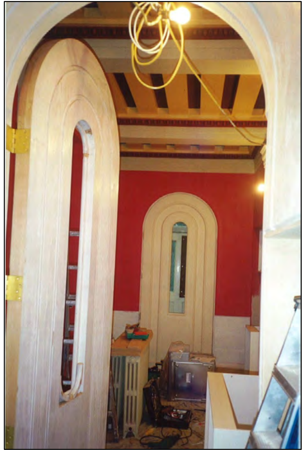
...and nearing completion.
