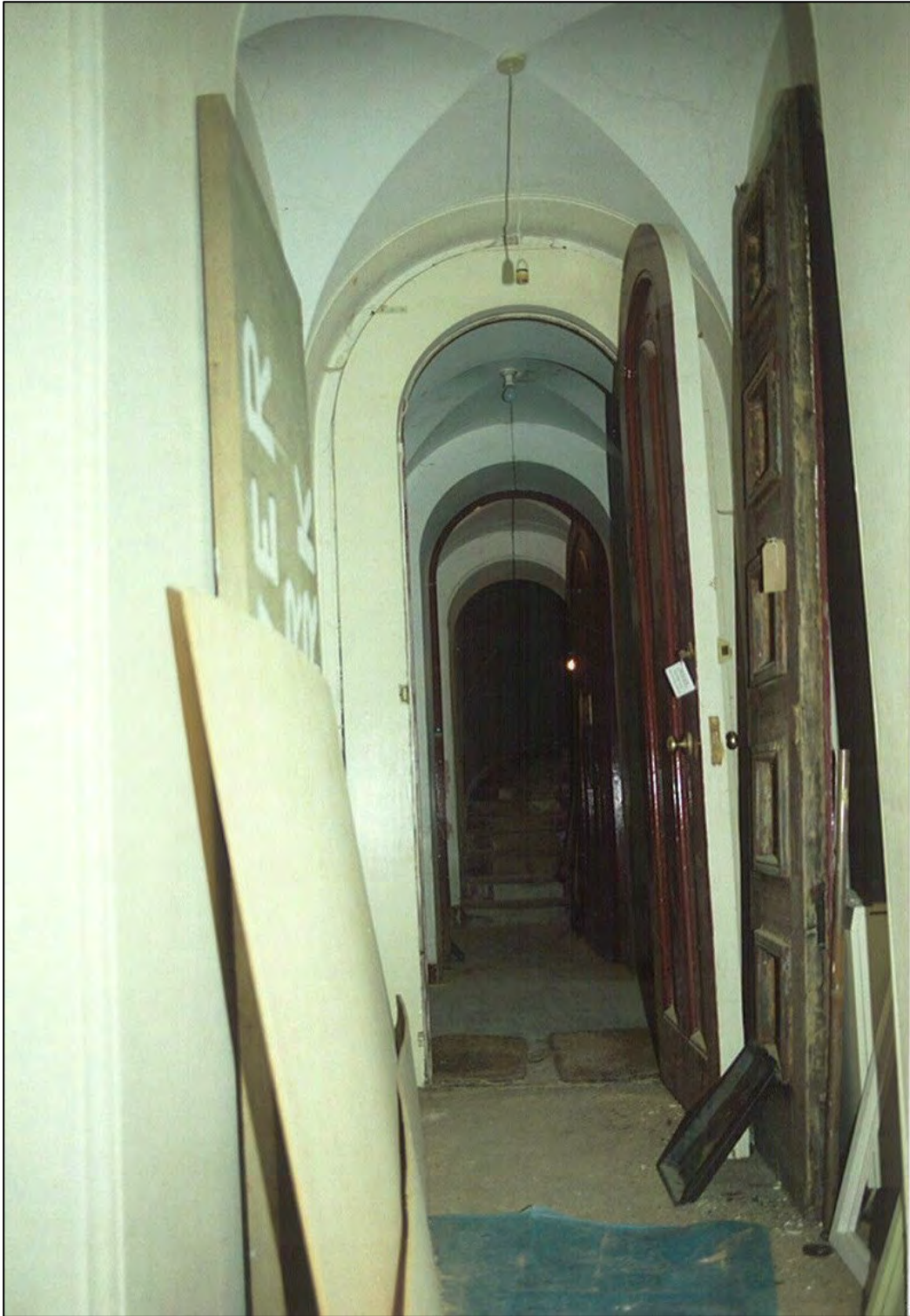
View along the corridor to the foot of the Tower steps.
