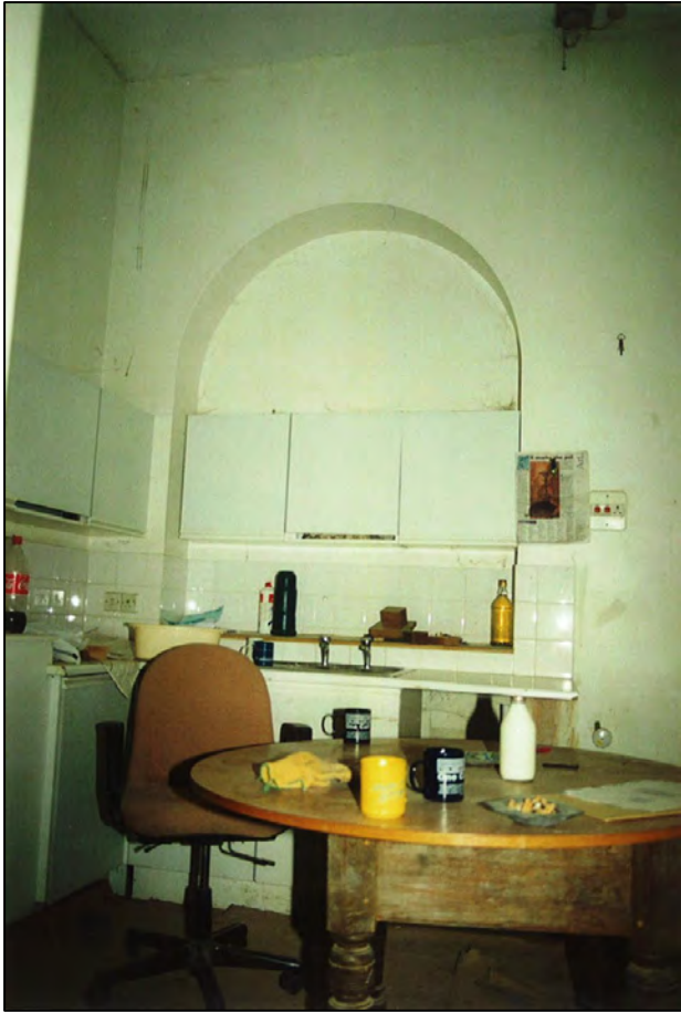
The kitchen before work started...
