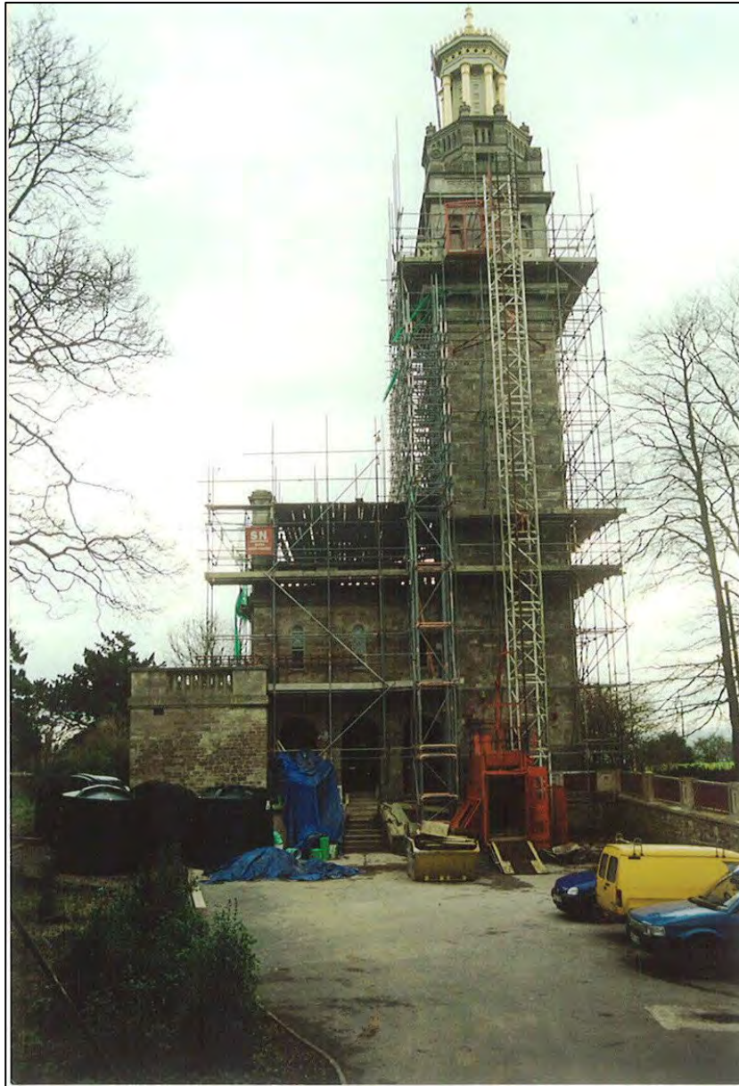
Figure 55: The Tower during the Beckford Tower Trust restoration, 1997-9.
