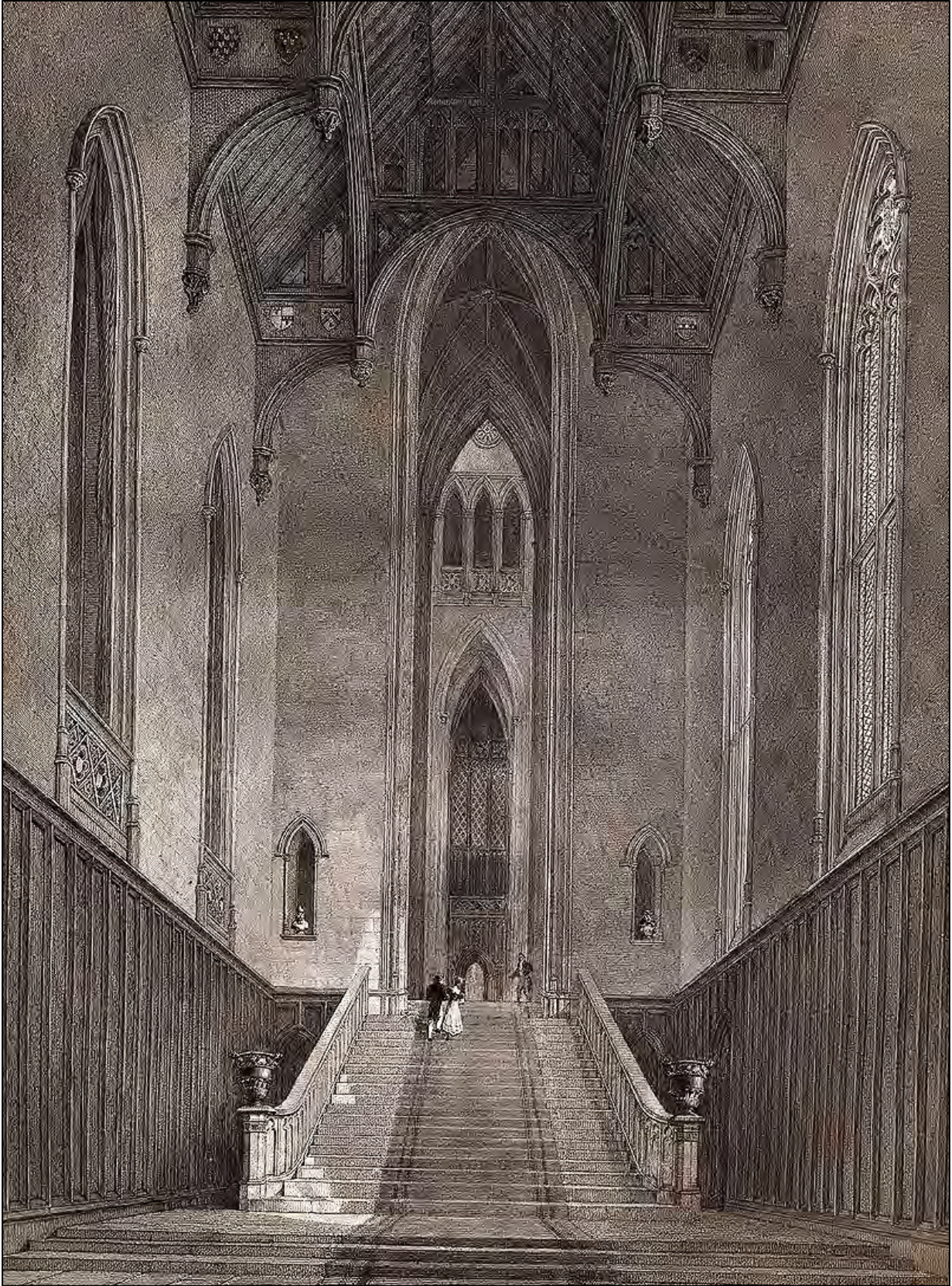
Figure 20: The Great Western Hall at Fonthill, leading through to the Octagon. The steps were an afterthought when Beckford realised that the space was unsuitable for a dining room.
