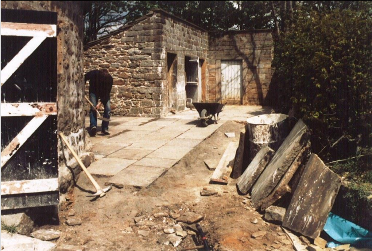
The old concrete that surrounded the building was replaced by stone flags.
