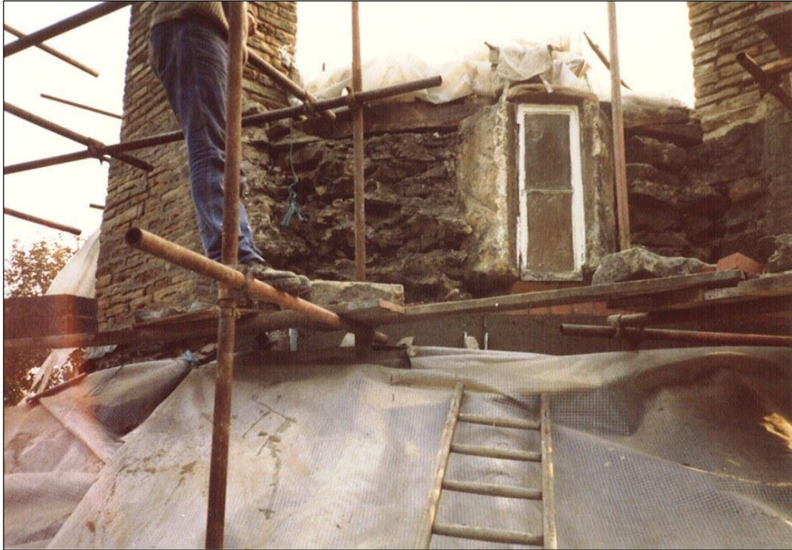
The top of the inner drum with the render removed, before facing repairs.
