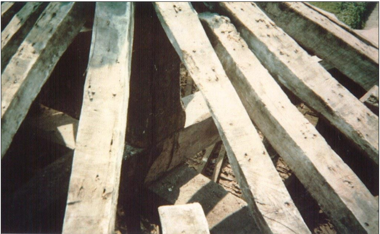
Crown post of upper roof structure.
