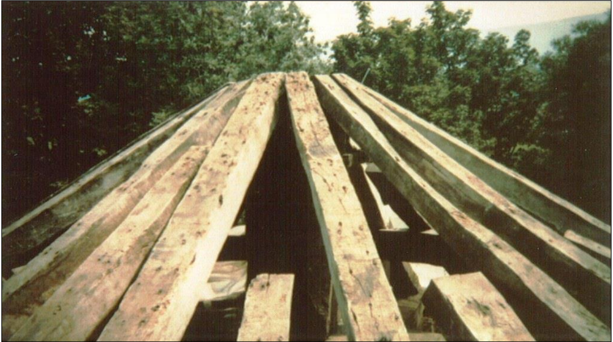
Upper roof structure.
