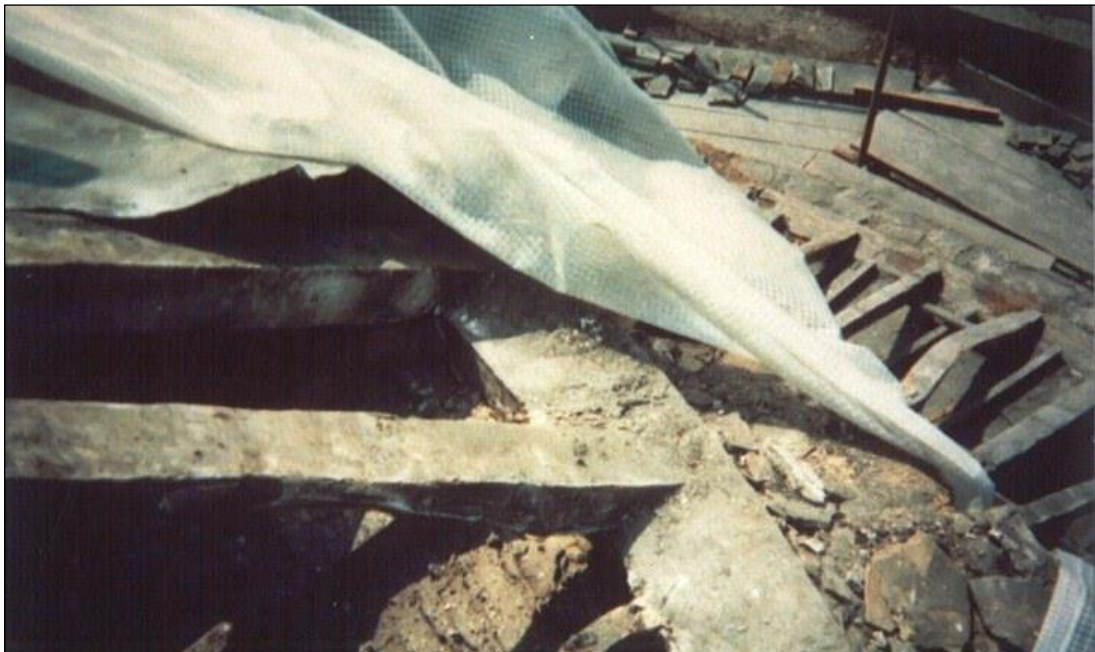
Wallplate of upper roof.
