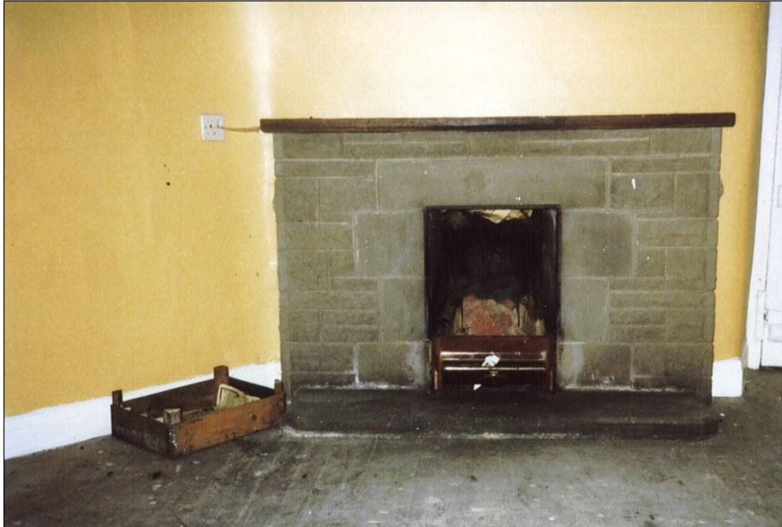
The fireplace in the sitting room, fitted in 1958. The softwood floorboards were replaced with elm here and in the bedrooms.
